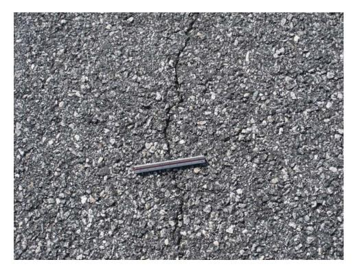
A01CS-20. Longitudinal and Transverse Cracking (Sample Unit #21).
