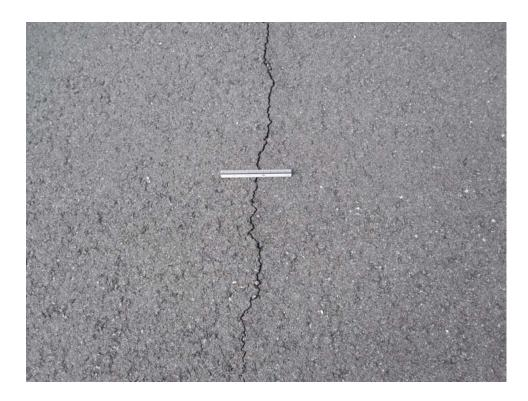
R624CS-10E. Longitudinal and Transverse Cracking (Sample Unit #46).
