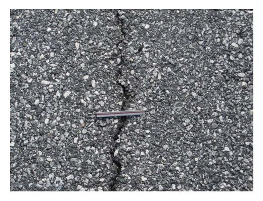
TFCS-40. Longitudinal and Transverse Cracking (Sample Unit #03).
