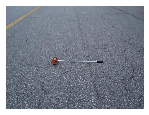
TCCS-30. Block Cracking (Sample Unit #01).
