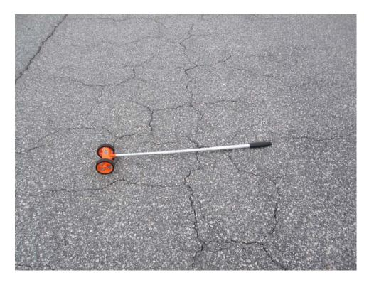
TCCS-40. Block Cracking (Sample Unit #14).
