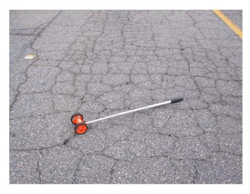
THANGCS-10. Alligator Cracking (Sample Unit #04).
