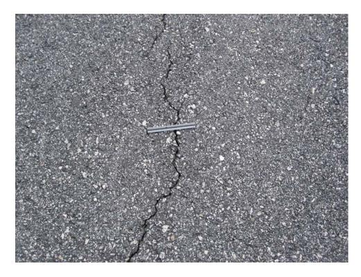
TACS-10. Longitudinal and Transverse Cracking (Sample Unit #02).
