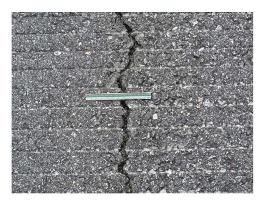
R624CS-20E. Longitudinal and Transverse Cracking (Sample Unit #01).
