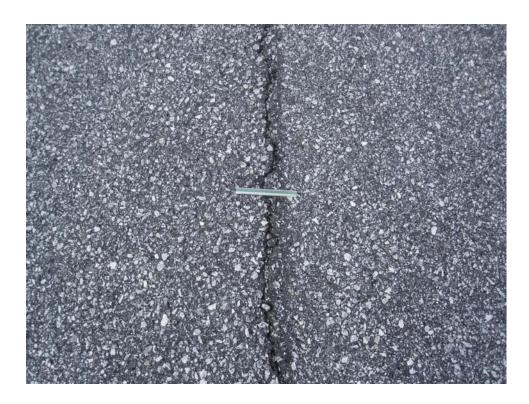
TDCS-10. Longitudinal and Transverse Cracking (Sample Unit #16).
