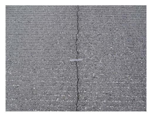
R624CS-20W. Longitudinal and Transverse Cracking (Sample Unit #15).
