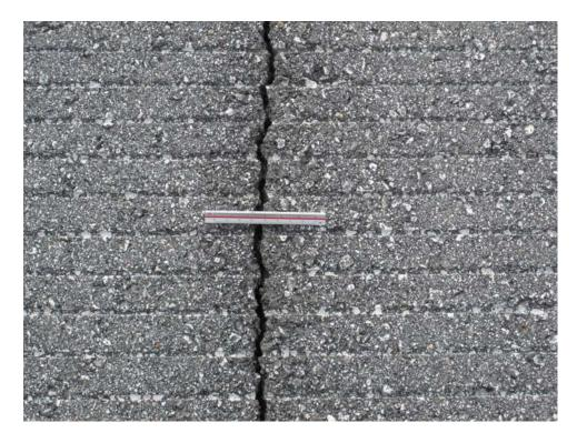
R624CS-20C. Longitudinal and Transverse Cracking (Sample Unit #06).
