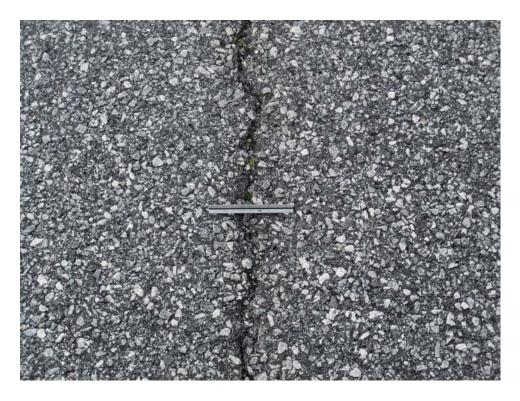
TDCS-20. Longitudinal and Transverse Cracking (Sample Unit #08).
