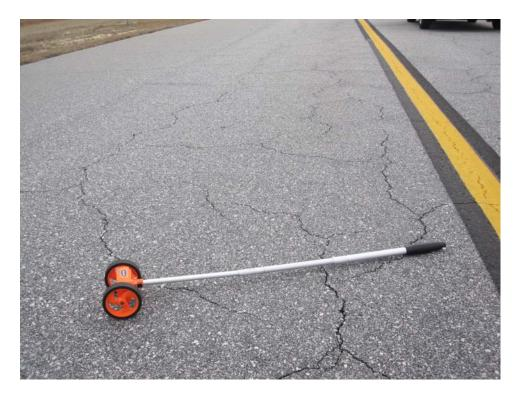
TFCS-20. Block Cracking (Sample Unit #11).
