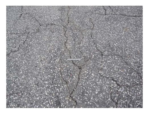
TCCS-40. Alligator Cracking (Additional Sample Unit #02).
