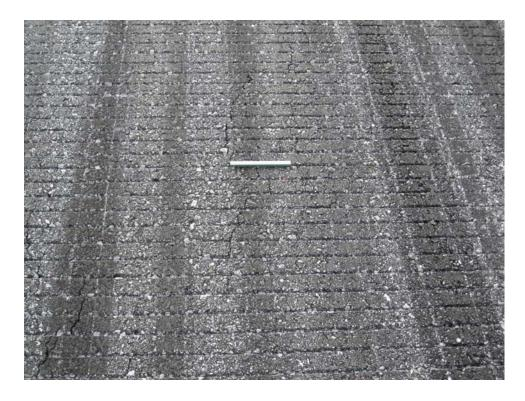
R624CS-20C. Alligator Cracking (Sample Unit #06).
