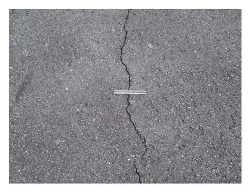
R624CS-10W. Longitudinal and Transverse Cracking (Sample Unit #44).
