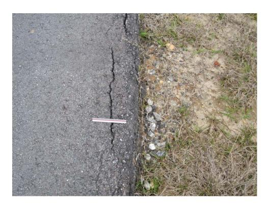
TCCS-10. Longitudinal and Transverse Cracking (Sample Unit #68).
