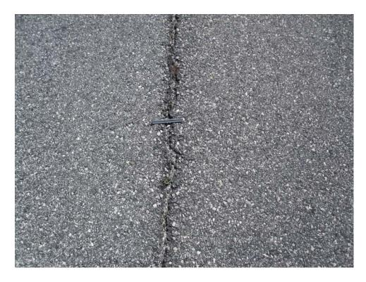
R1331CS-10N. Longitudinal and Transverse Cracking (Sample Unit #14).
