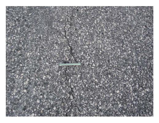
A01CS-10. Longitudinal and Transverse Cracking (Sample Unit #71).
