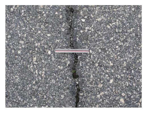
TFCS-10. Longitudinal and Transverse Cracking (Sample Unit #08).
