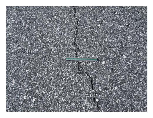
TD3CS-10. Longitudinal and Transverse Cracking (Sample Unit #03).
