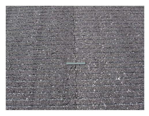
R624CS-10C. Longitudinal and Transverse Cracking (Sample Unit #35).
