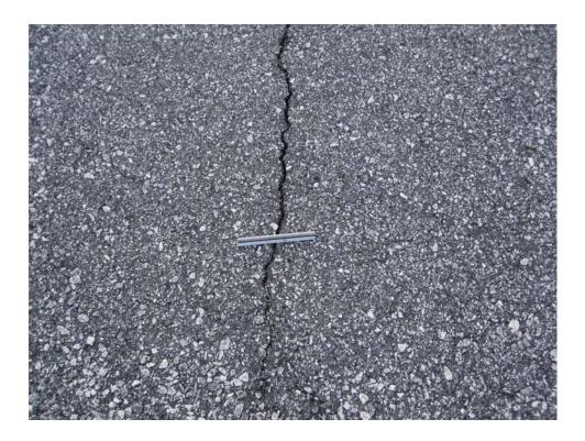
TD2CS-10. Longitudinal and Transverse Cracking (Sample Unit #02).
