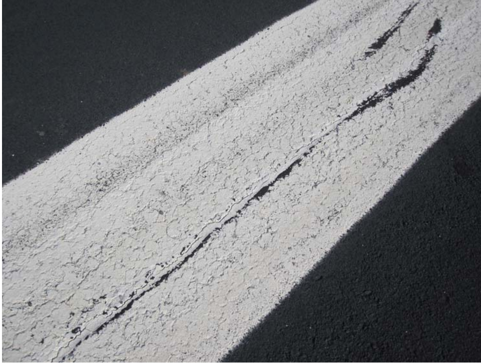
R220AT-30. Satisfactory Paint.
