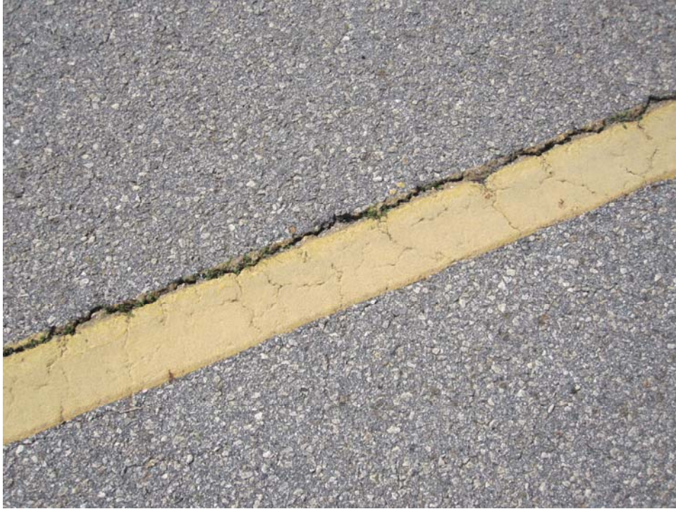
THANGAT-10. Satisfactory Paint.
