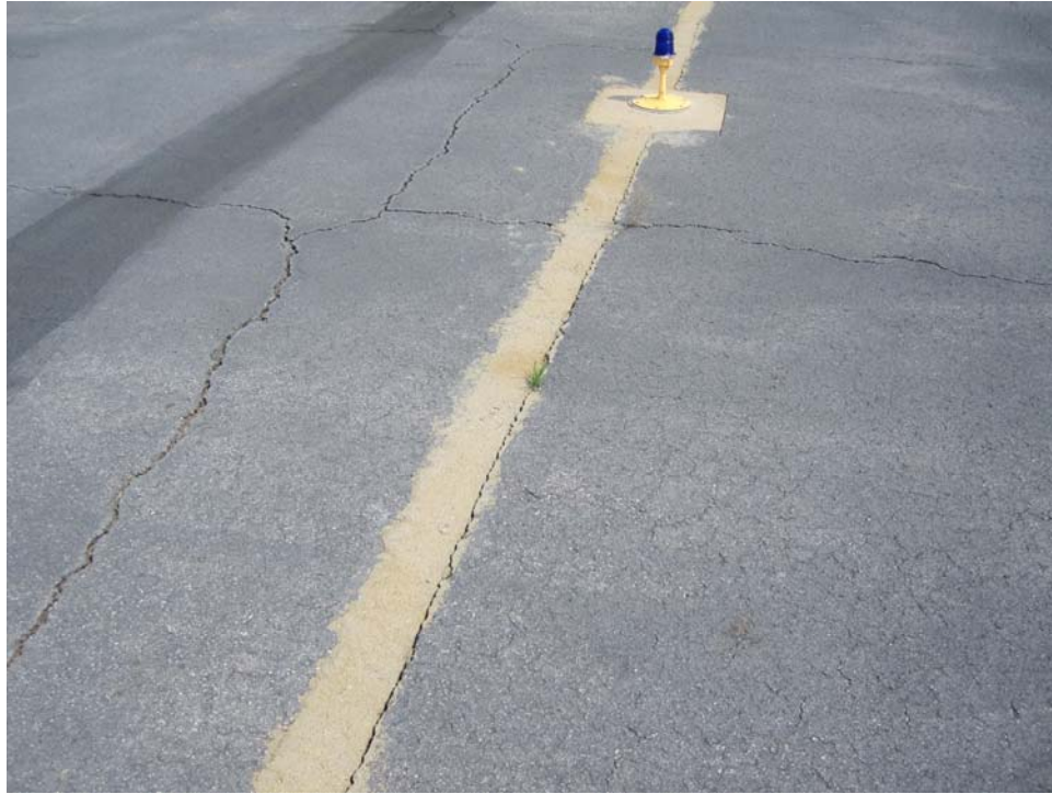
A01AT-30. Patching (Sample Unit #07).
