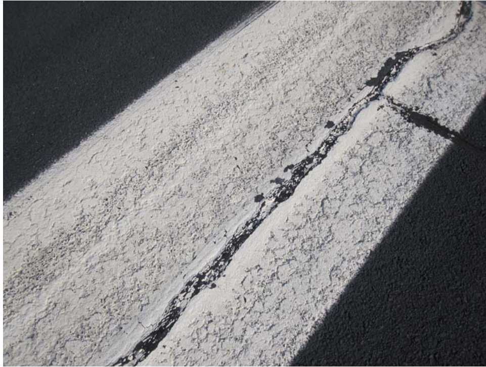
R220AT-10. Satisfactory Paint.
