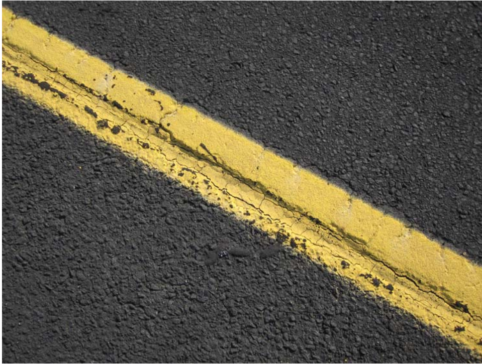
TBAT-20. Satisfactory Paint.
