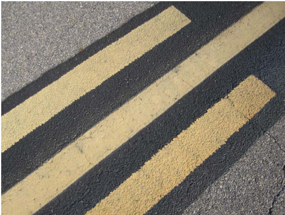
TBAT-10. Satisfactory Paint.
