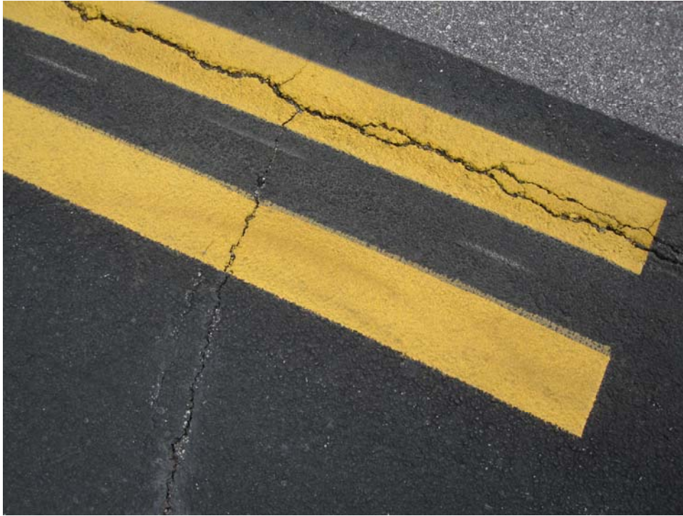
A01AT-20. Satisfactory Paint.
