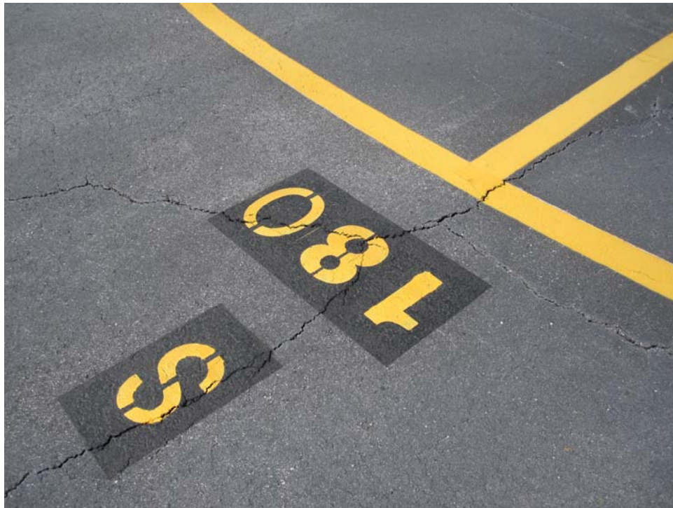
A01AT-30. Satisfactory Paint.
