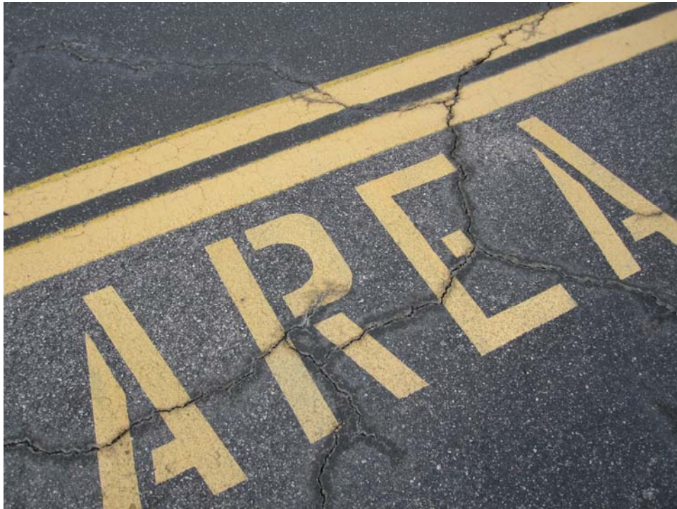
A01AT-10. Satisfactory Paint.
