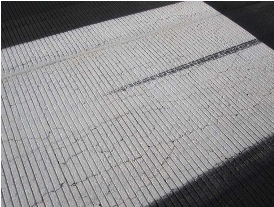
R927AT-20. Satisfactory Paint.
