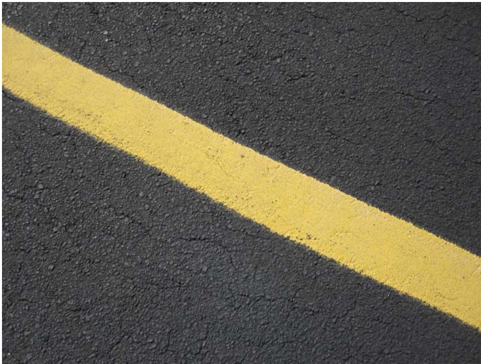
TBAT-30. Satisfactory Paint.
