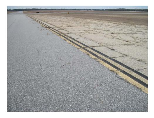
TEAY-30. Block Cracking (Sample Unit #4).
