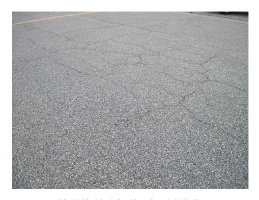
TCAY-20. Block Cracking (Sample Unit #3).
