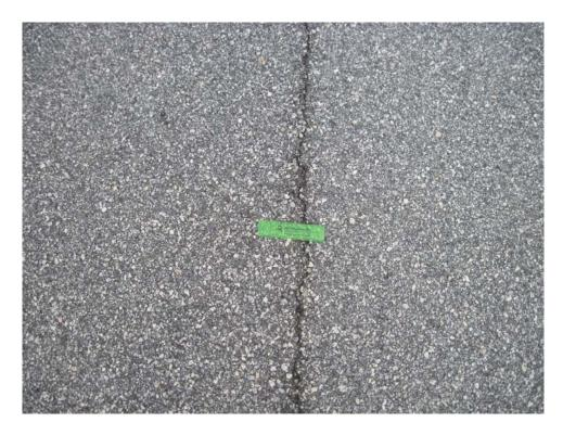
TEAY-30. Longitudinal and Transverse Cracking and Weathering (Sample Unit #2).
