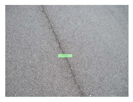
TEAY-10. Longitudinal and Transverse Cracking (Sample Unit #10).
