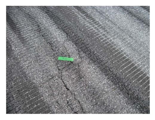
R422AY-10. Alligator Cracking (Sample Unit #120).
