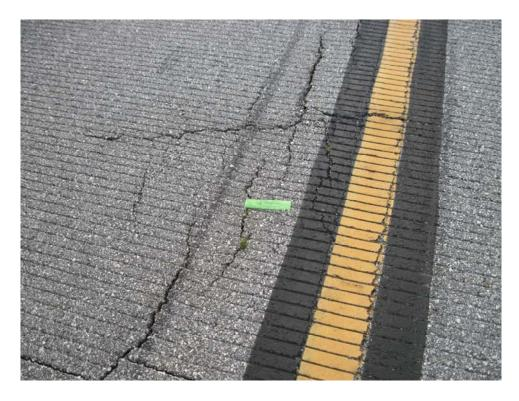
R1634AY-10. Alligator Cracking (Sample Unit #93).
