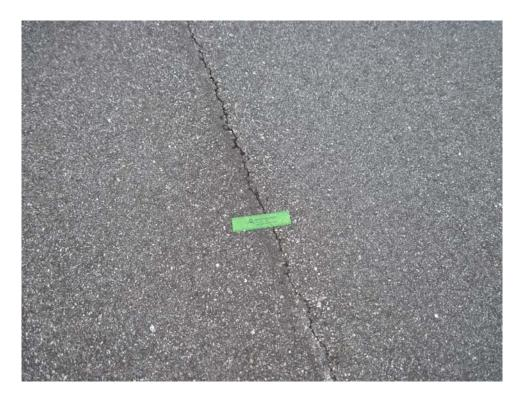
TAAY-10. Longitudinal and Transverse Cracking (Sample Unit #6).
