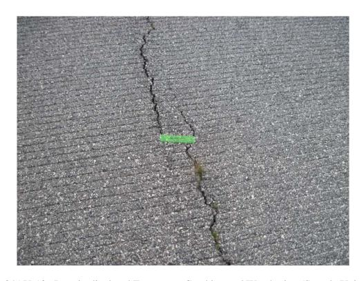
R1634AY-10. Longitudinal and Transverse Cracking and Weathering (Sample Unit #5).
