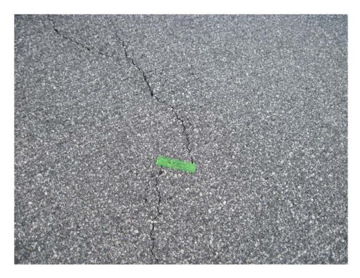
R422AY-10. Longitudinal and Transverse Cracking and Weathering (Sample Unit #134).
