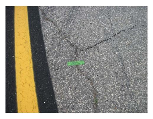
TSAY-10. Longitudinal and Transverse Cracking and Weathering (Sample Unit #1).
