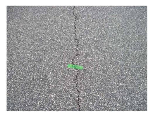
A02AY-10. Longitudinal and Transverse Cracking (Sample Unit #4).
