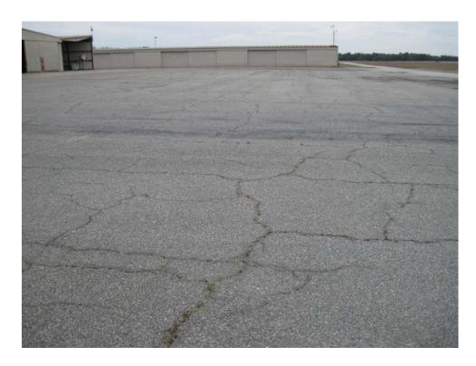
A01AY-10. Block Cracking (Sample Unit #11).
