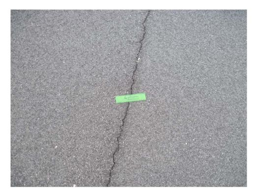
TBAY-10. Longitudinal and Transverse Cracking (Sample Unit # 12).
