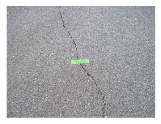
TCAY-10. Longitudinal and Transverse Cracking (Sample Unit #3).
