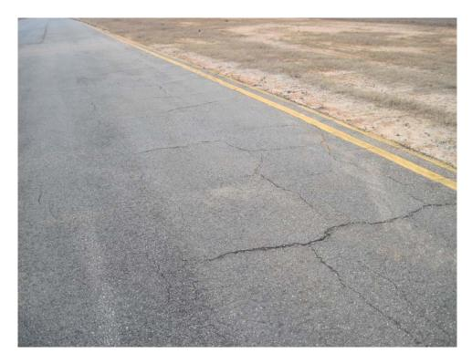
TEAY-20. Block Cracking (Sample Unit #3).
