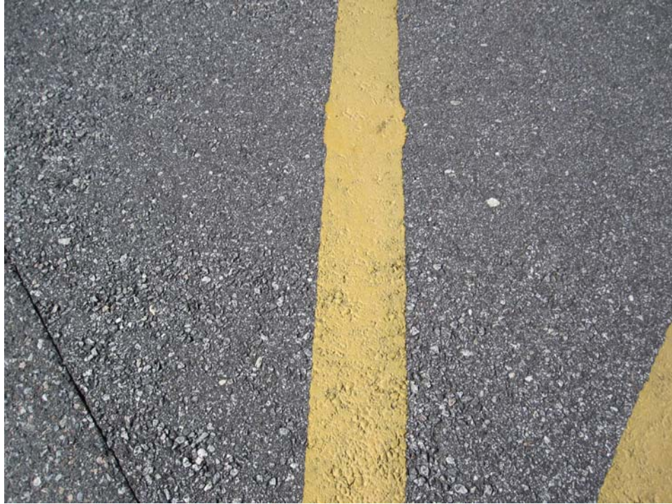
TAAD-10. Satisfactory Paint.
