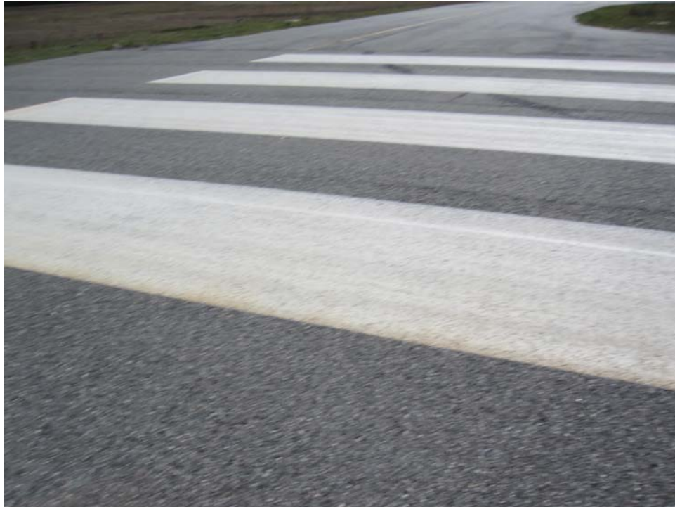
R523AD-10. Satisfactory Paint.
