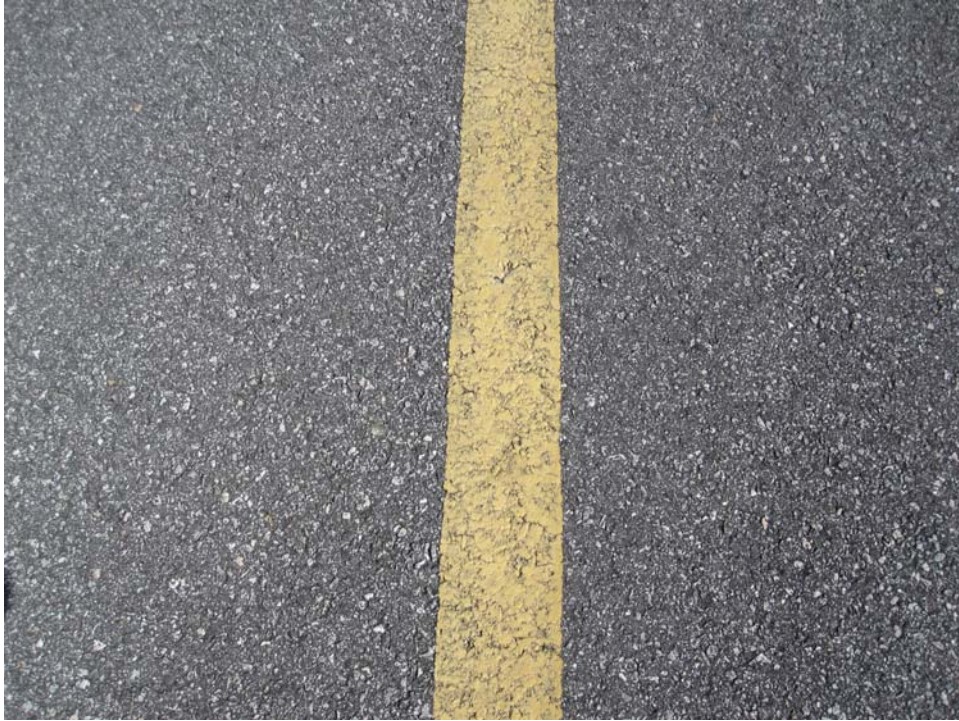
TBAD-20. Satisfactory Paint.
