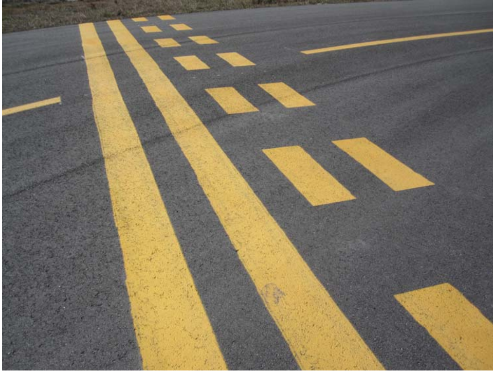
TBAD-10. Satisfactory Paint.
