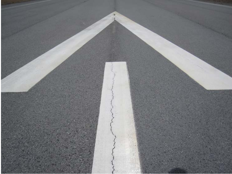
R1533AD-10. Satisfactory Paint.
