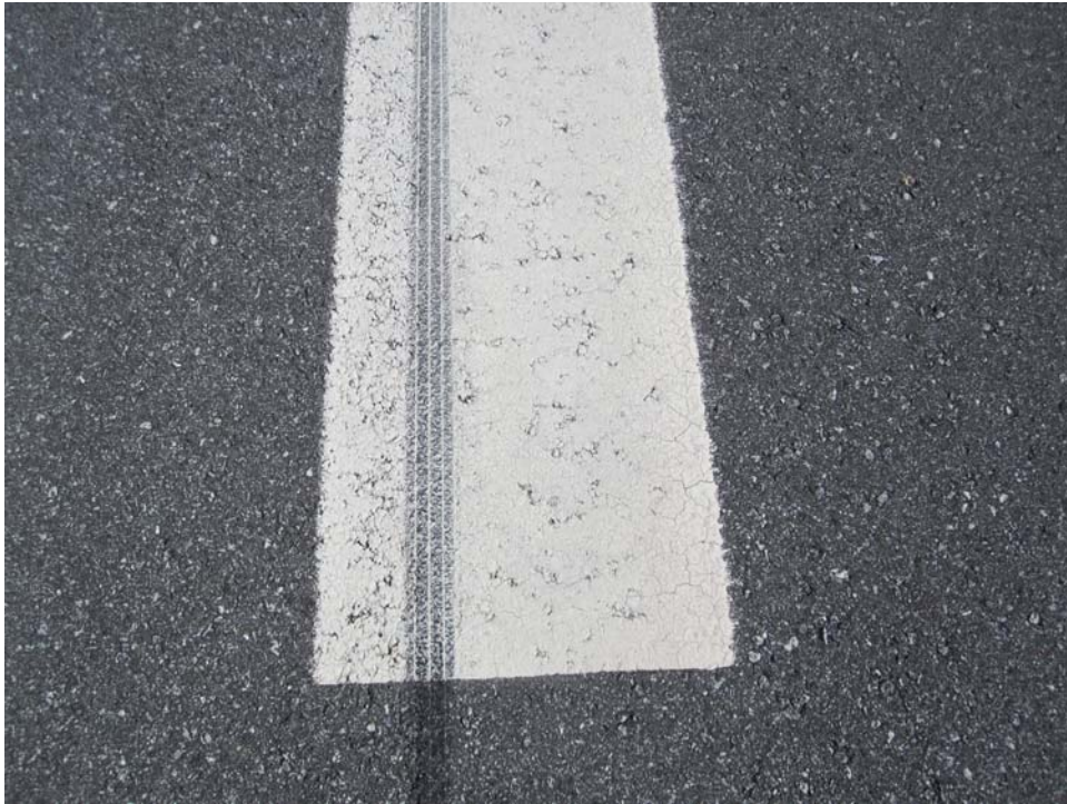
R523AD-20. Satisfactory Paint.
