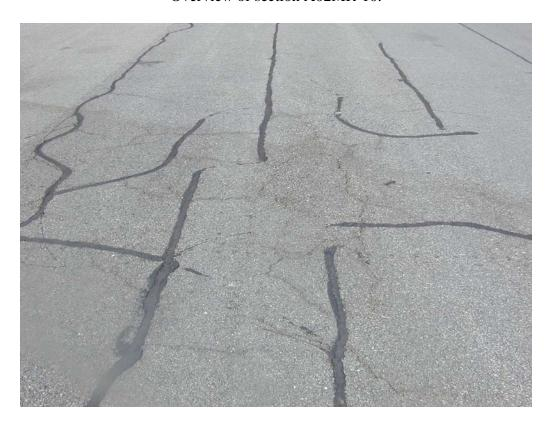
Alligator cracking in section A02MR-10.
