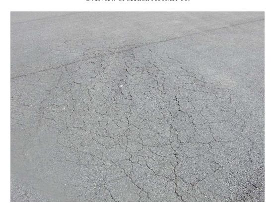
Alligator cracking in section A01MR-60.
