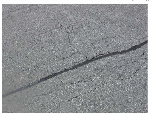
Alligator cracking in section TBMR-10.
