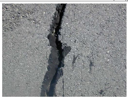
L&T cracking in section TAMR-10.
