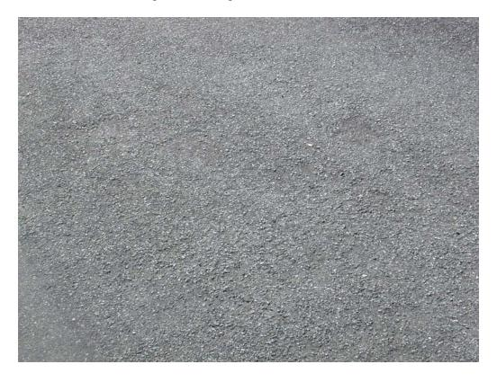
Raveling and Weathering in section A01MR-50.
