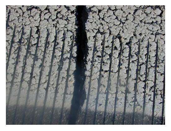
L&T cracking in section R927MR-10.
