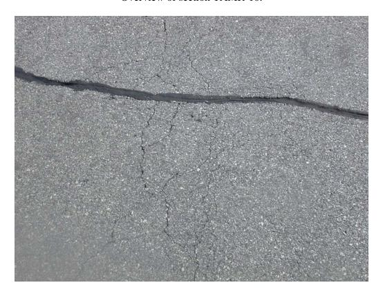
Alligator cracking in section TAMR-10.
