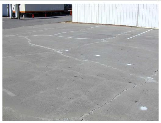
Shattered slab in section A01MR-20.
