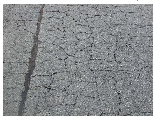
Alligator cracking in section A01MR-50.
