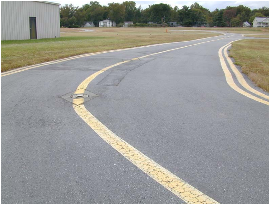
Overview of section HELIAP-10.
