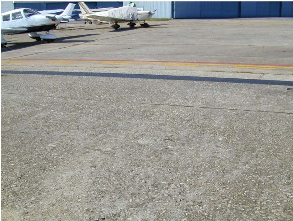
Overview of section ANWRAMPAP-20.
