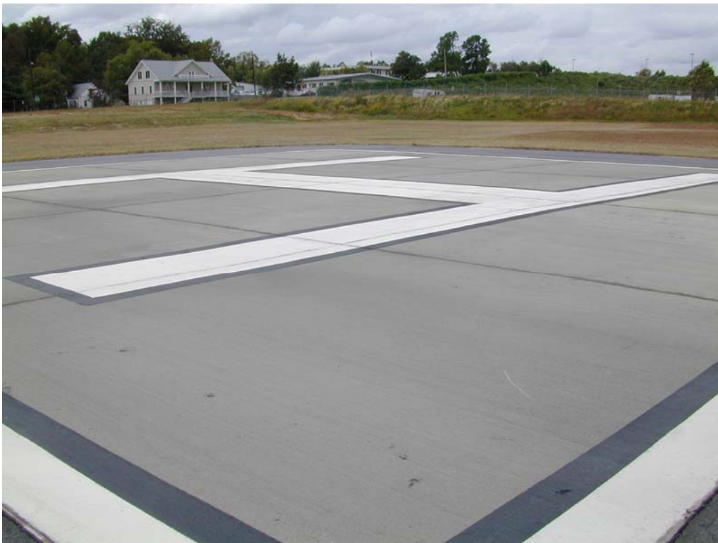
Overview of section HELIAP-20.
