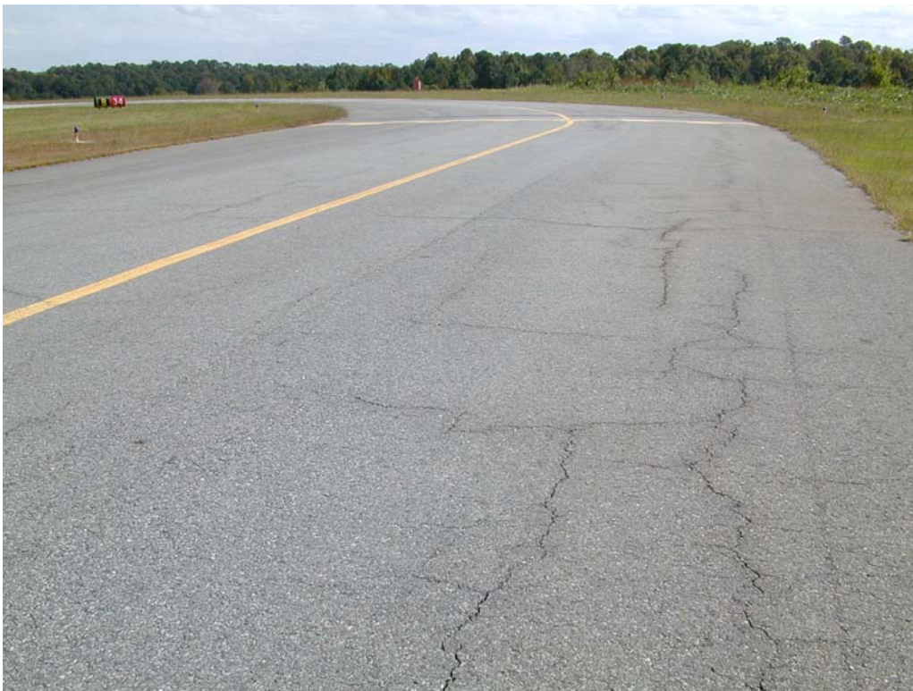
Overview of section TBAP-10.
