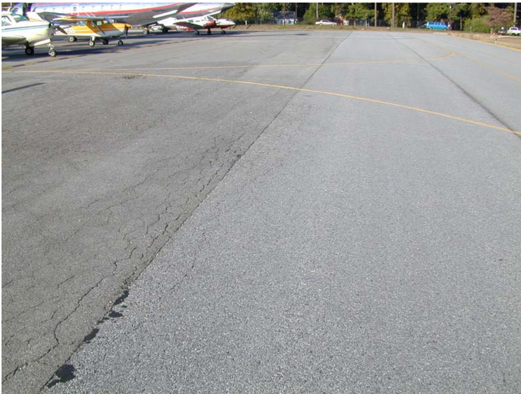
Overview of area being replaced in section TKAP-20.
