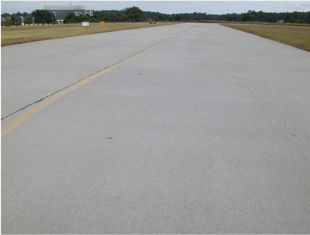
Overview of section TAAP-30.
