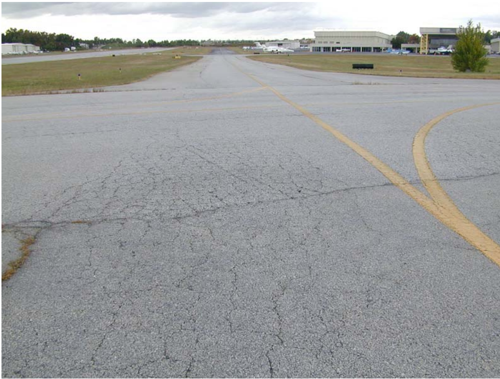
Alligator cracking (additional sample unit) in section TDAP-10.
