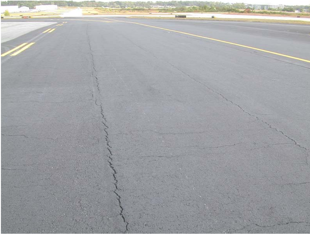
Overview of section TAAP-20.
