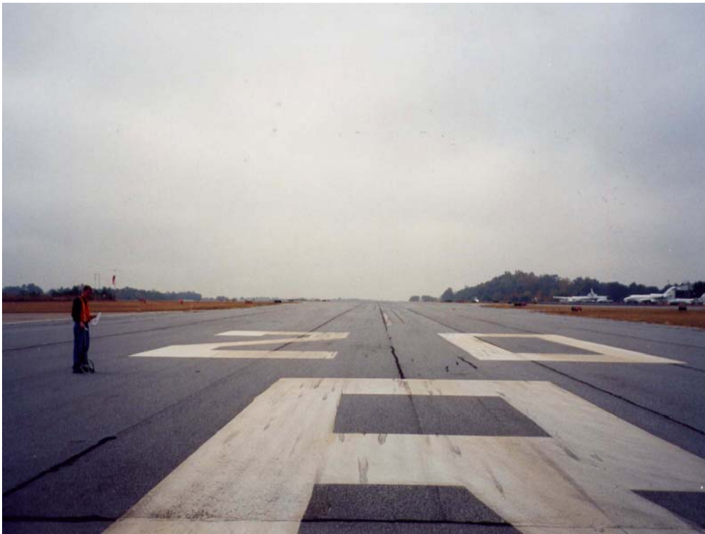
Overview of section R2L20RAP-10.
