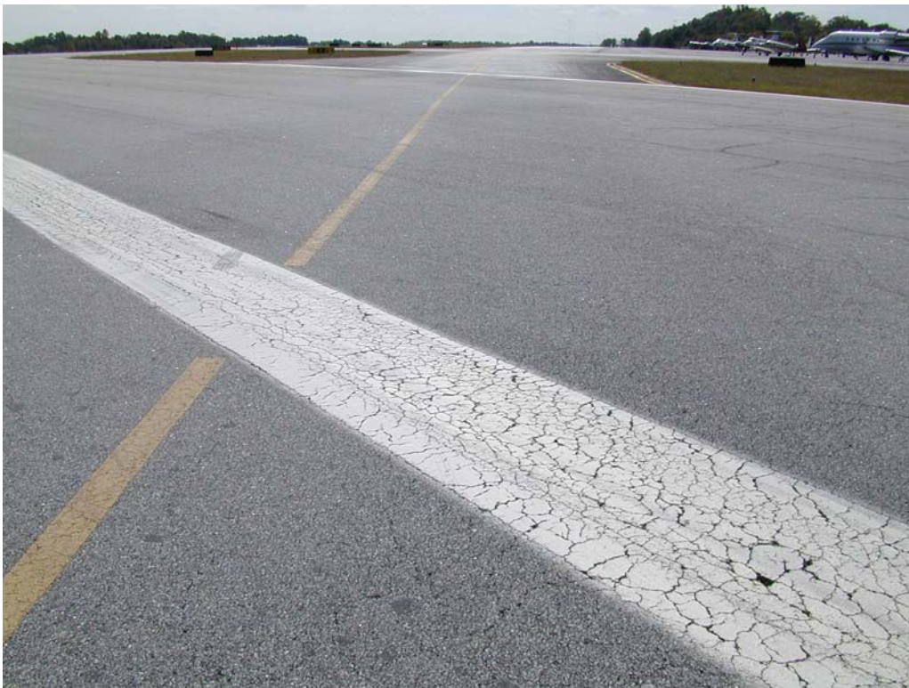
Overview of area being replaced in section R1634AP-10.
