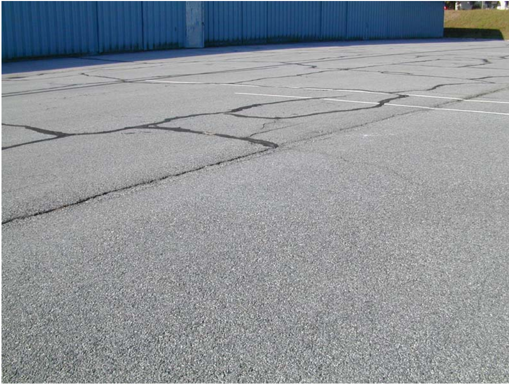
Overview of section ANWRAMPAP-10.
