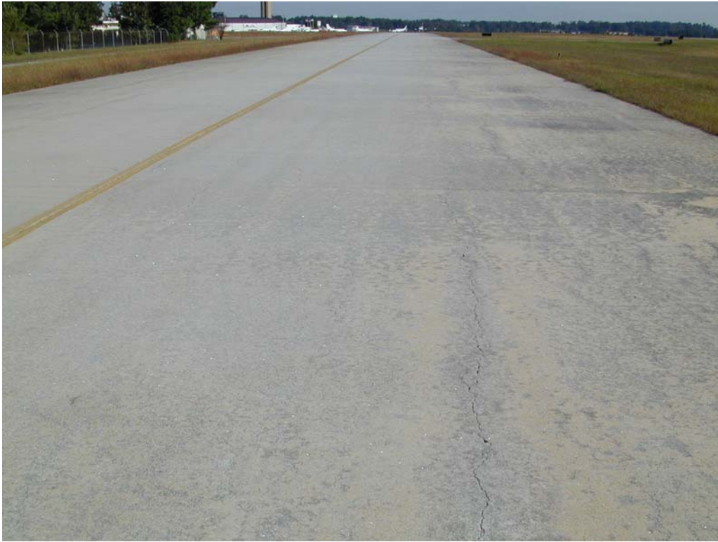
Overview of section TAAP-10.
