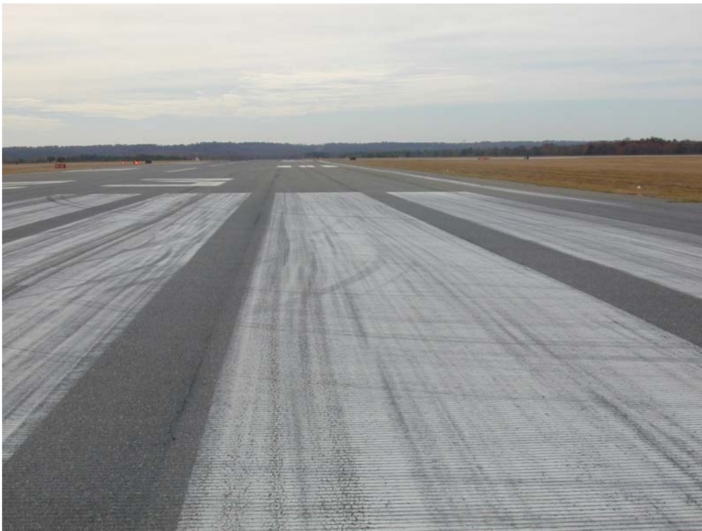
Overview of section R523MGRA-10N.
