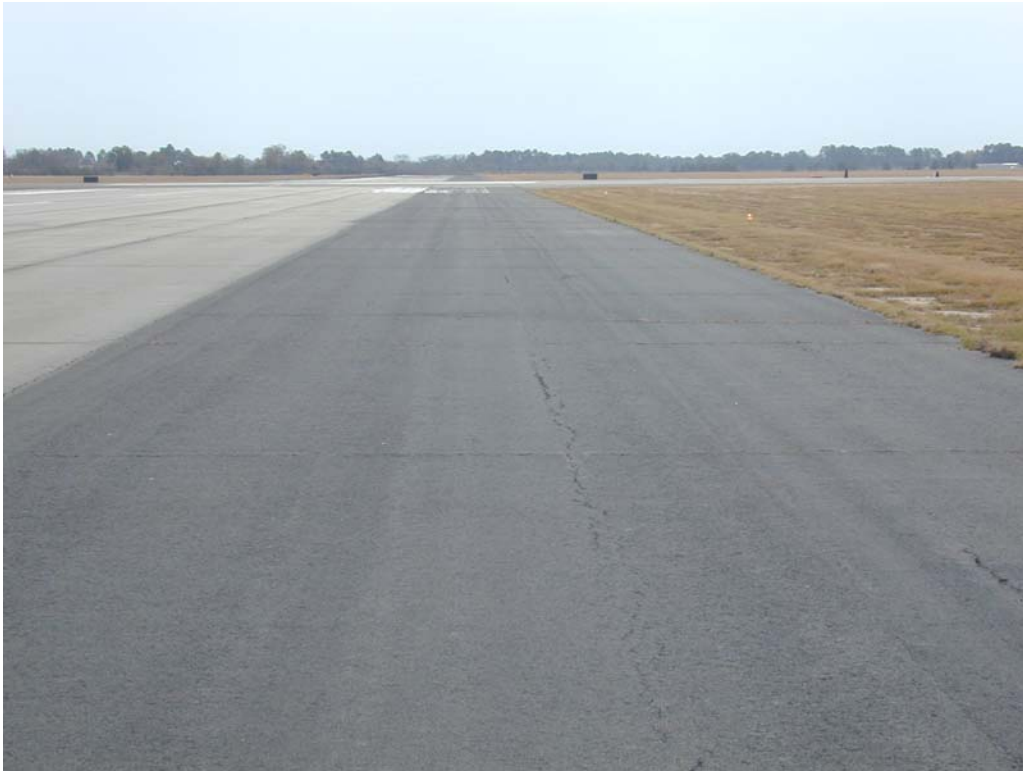
Overview of section R1331MGRA-10S.
