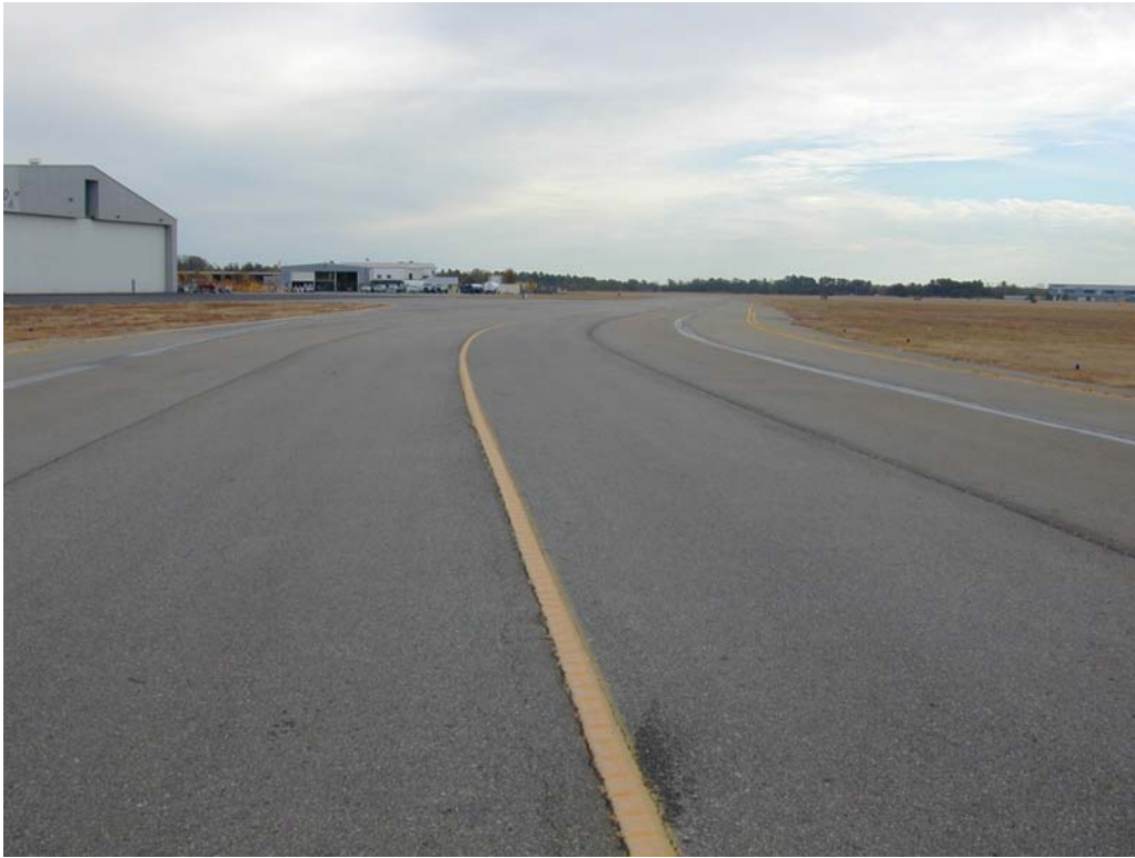
Overview of section TCMGRA-20.
