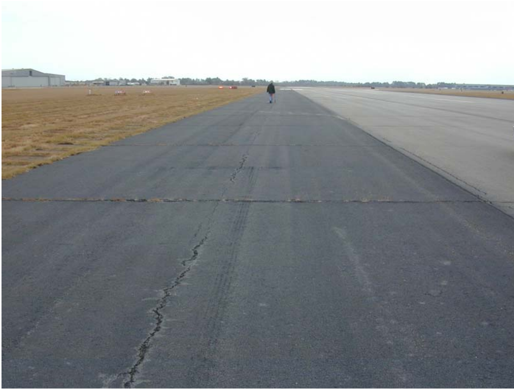
Overview of section R1331MGRA-10N.
