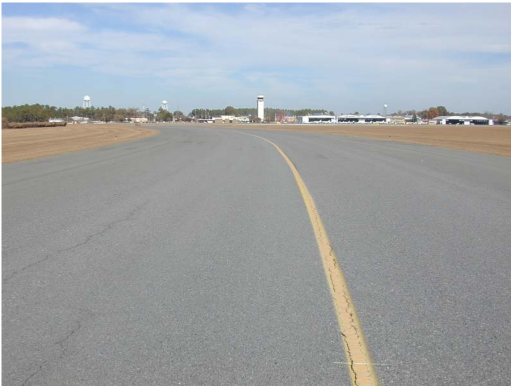
Overview of section TBMGRA-20.
