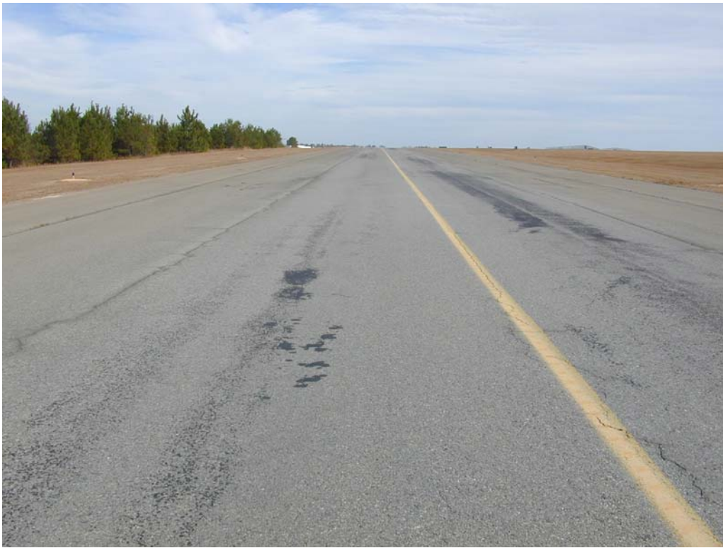
Overview of section TBMGRA-30.
