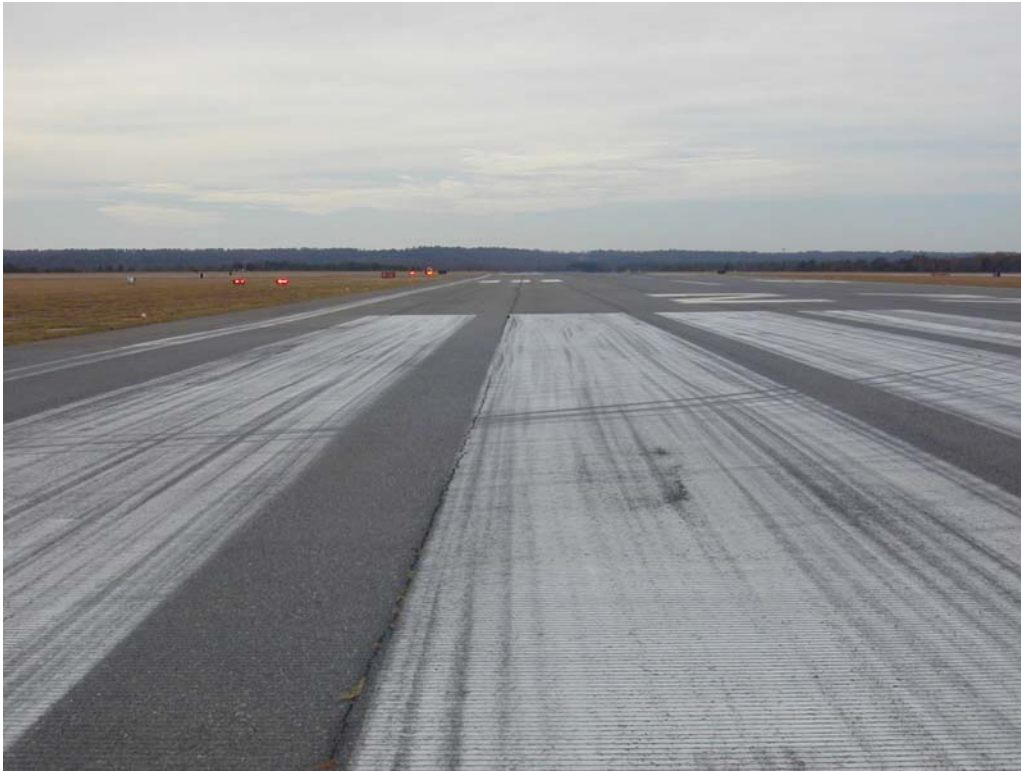
Overview of section R523MGRA-10S.
