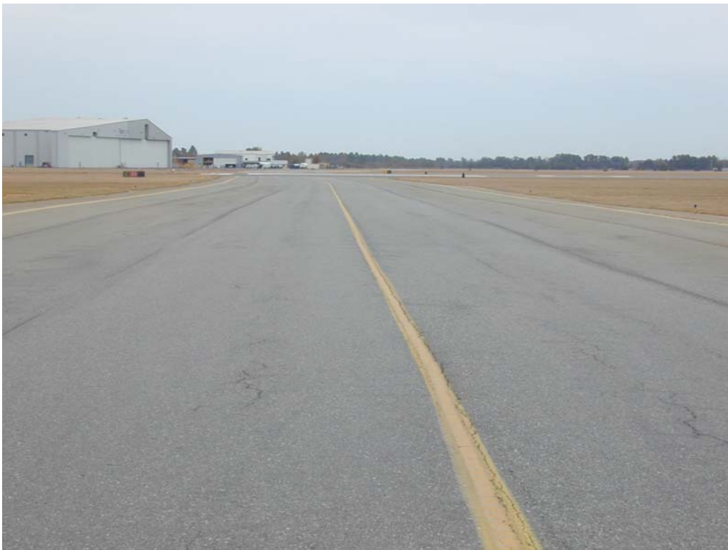
Overview of section TCMGRA-10.
