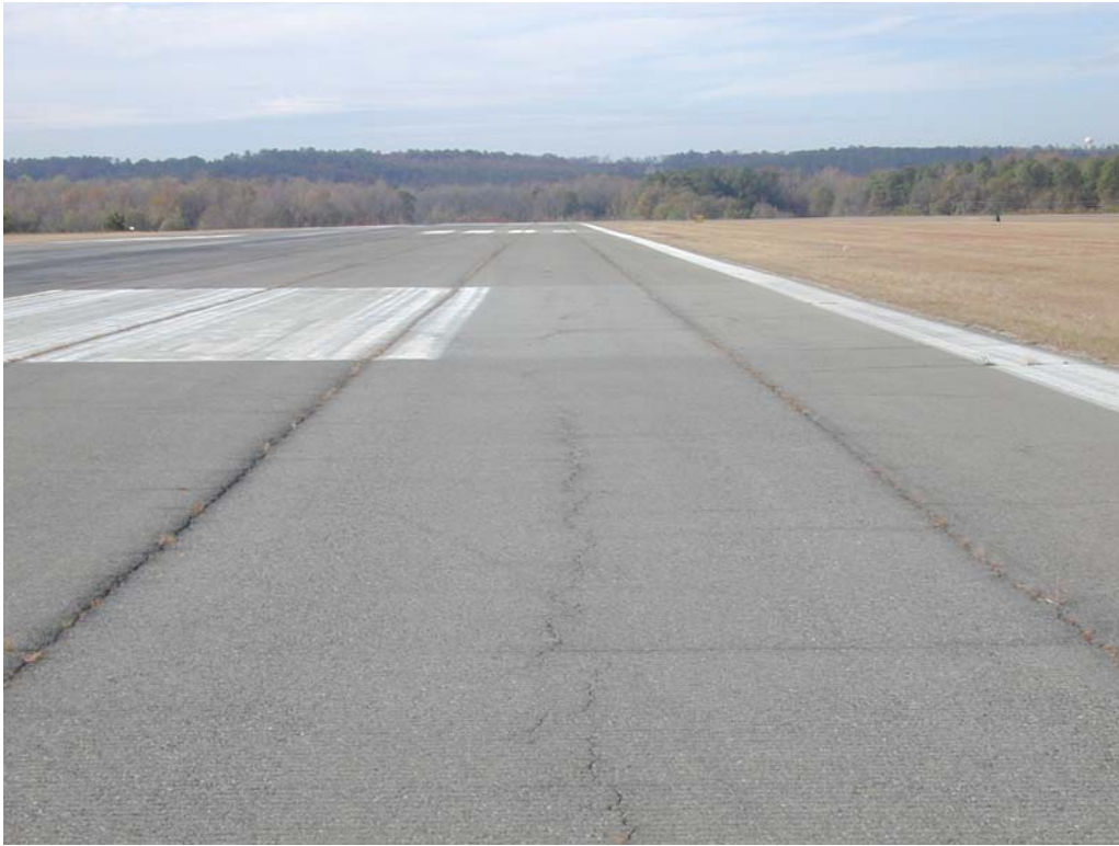
Overview of section R523MGRA-20N.
