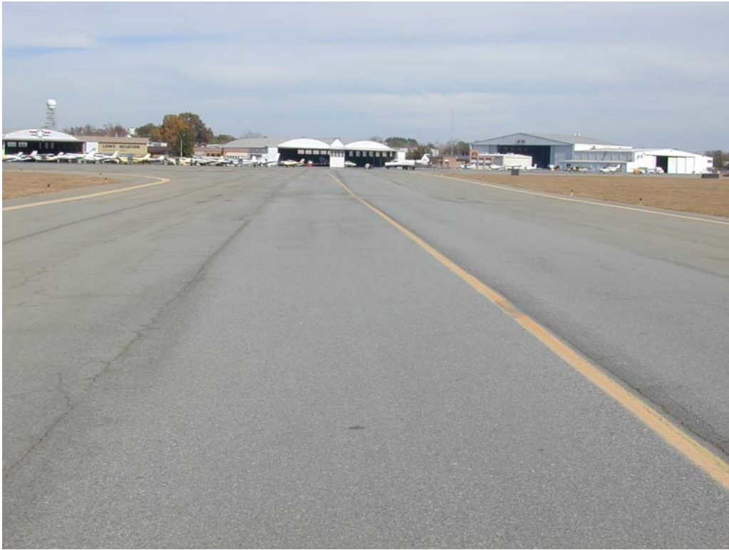
Overview of section TBMGRA-10.
