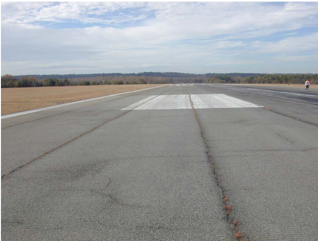
Overview of section R523MGRA-20S.
