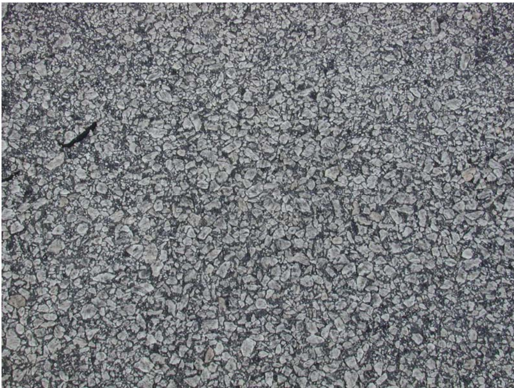
Raveling and weathering in section T927AB-10.
