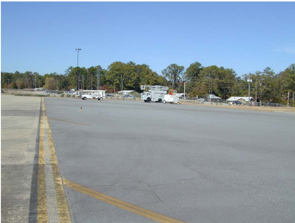
Overview of shoulder in section ATERMCL-10.
