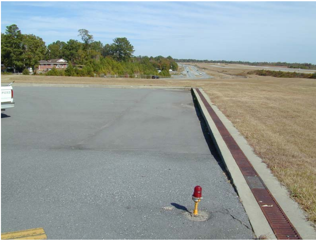
Overview of shoulder and edge drains in section ATERMCL-10.
