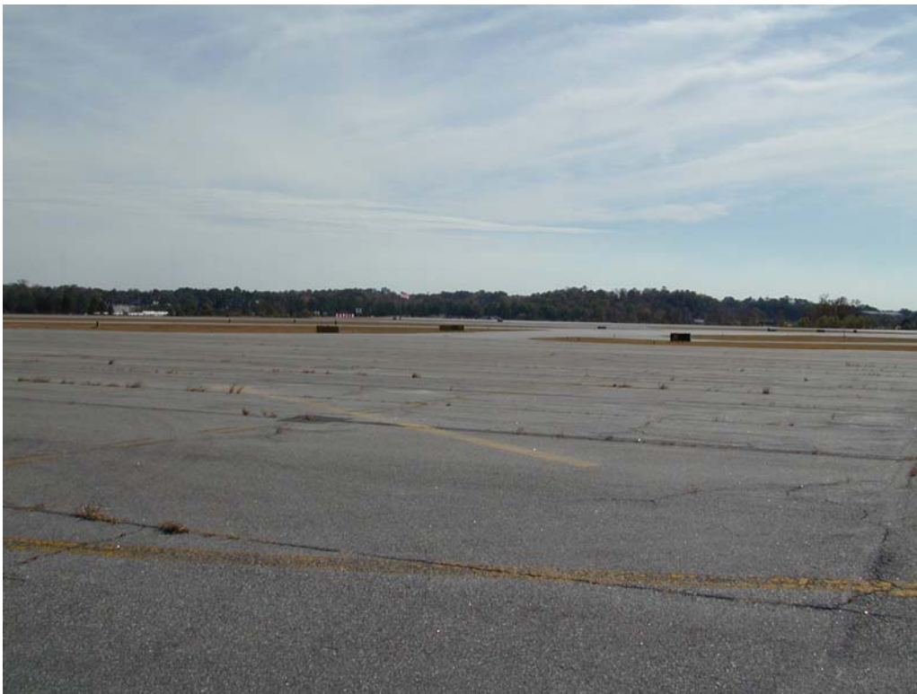
Overview of section A01CL-20 prior to rehabilitation.
