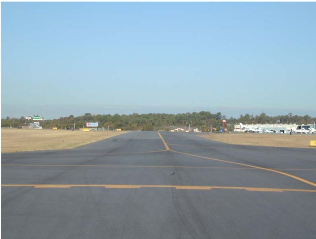
Overview of section TDCL-10.
