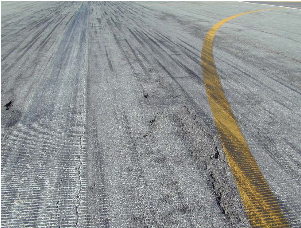
Overview of spring 2002 rehabilitation in section R523CL-10C.
