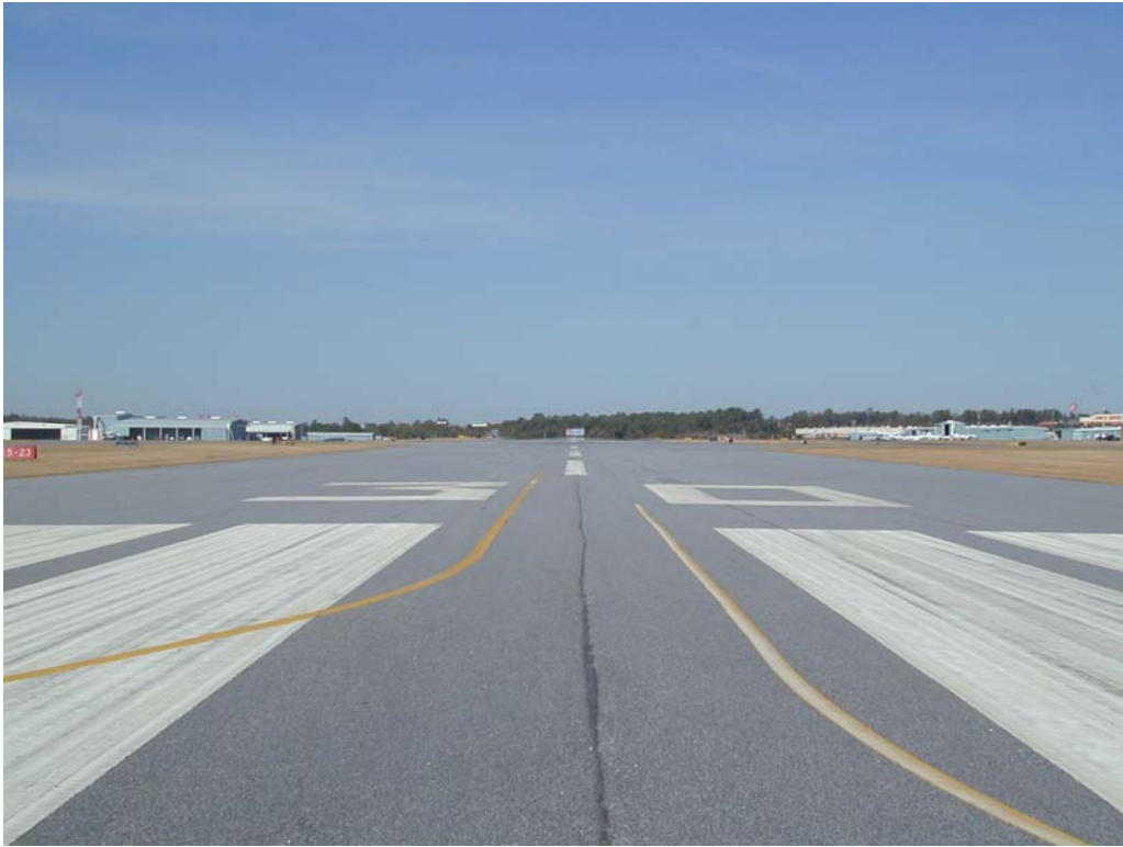
Overview of section R1230CL-10C.
