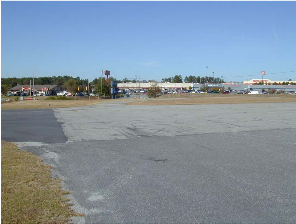
Overview of end of section A01CL-10.
