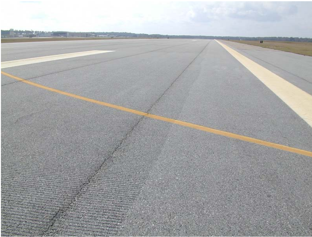
Overview of section R725GJP-20N.
