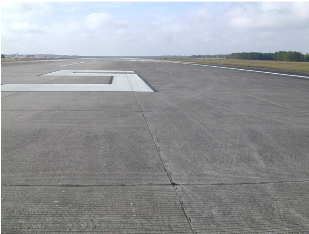
Overview of section R725GJP-30N.
