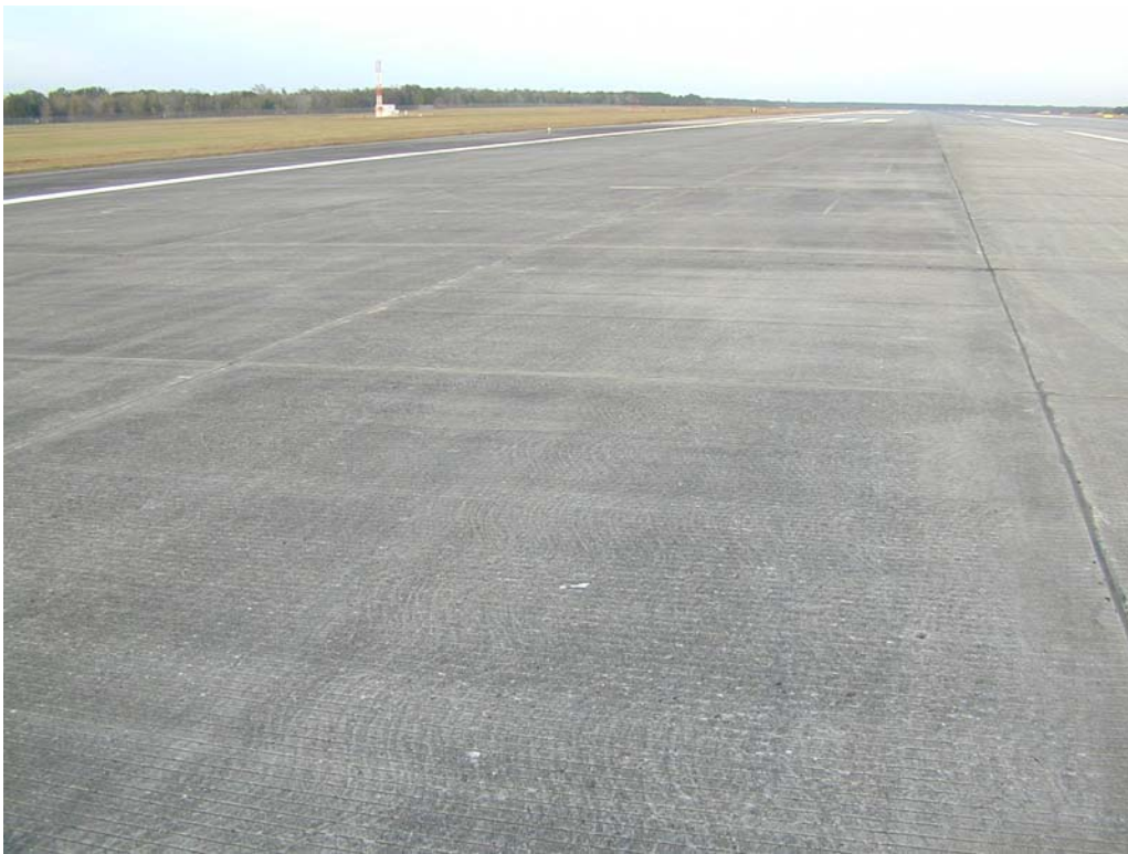
Overview of section R725GJP-10N.
