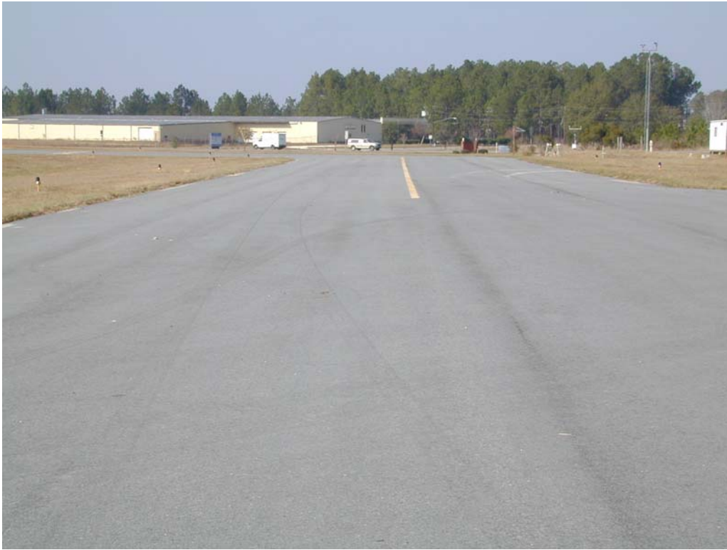
Overview of section TBAL-10.
