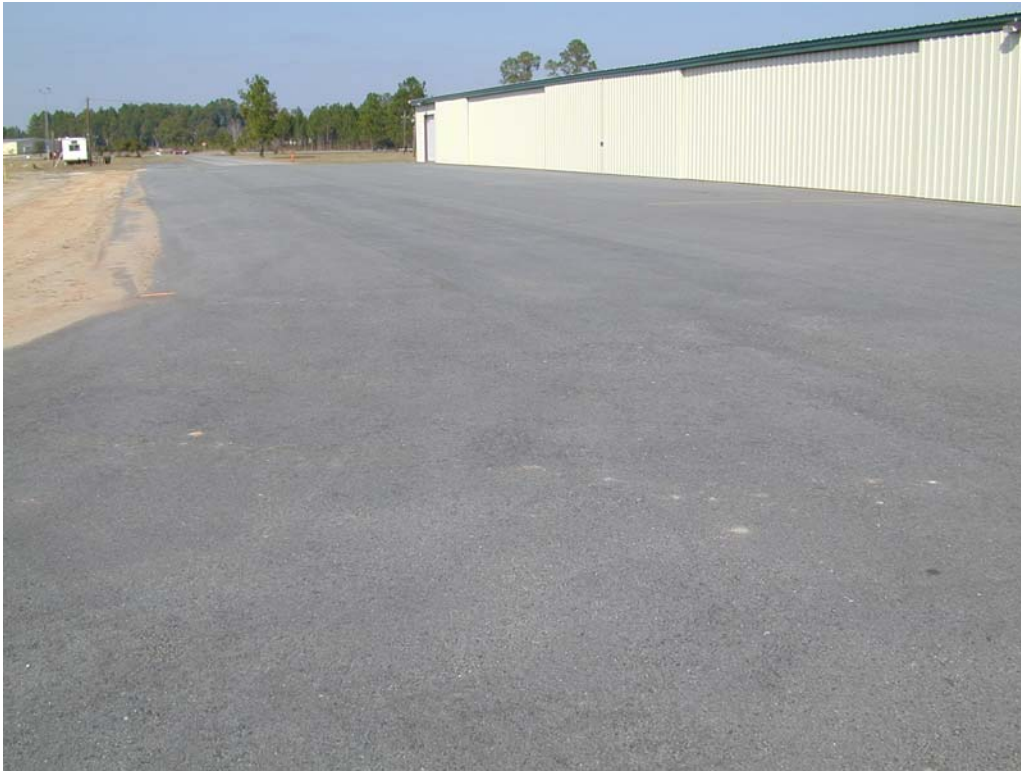
Overview of section TH01AL-10.
