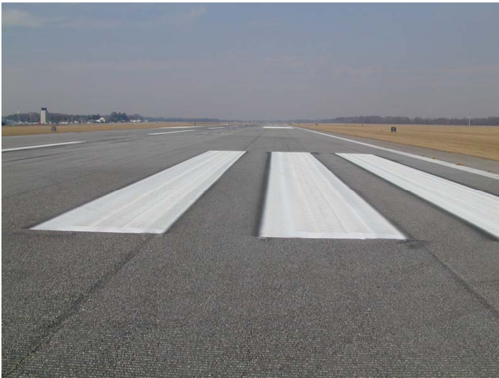
Overview of section R1735AGR-10E.
