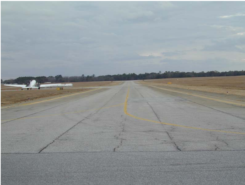
Overview of section TEAB-20.
