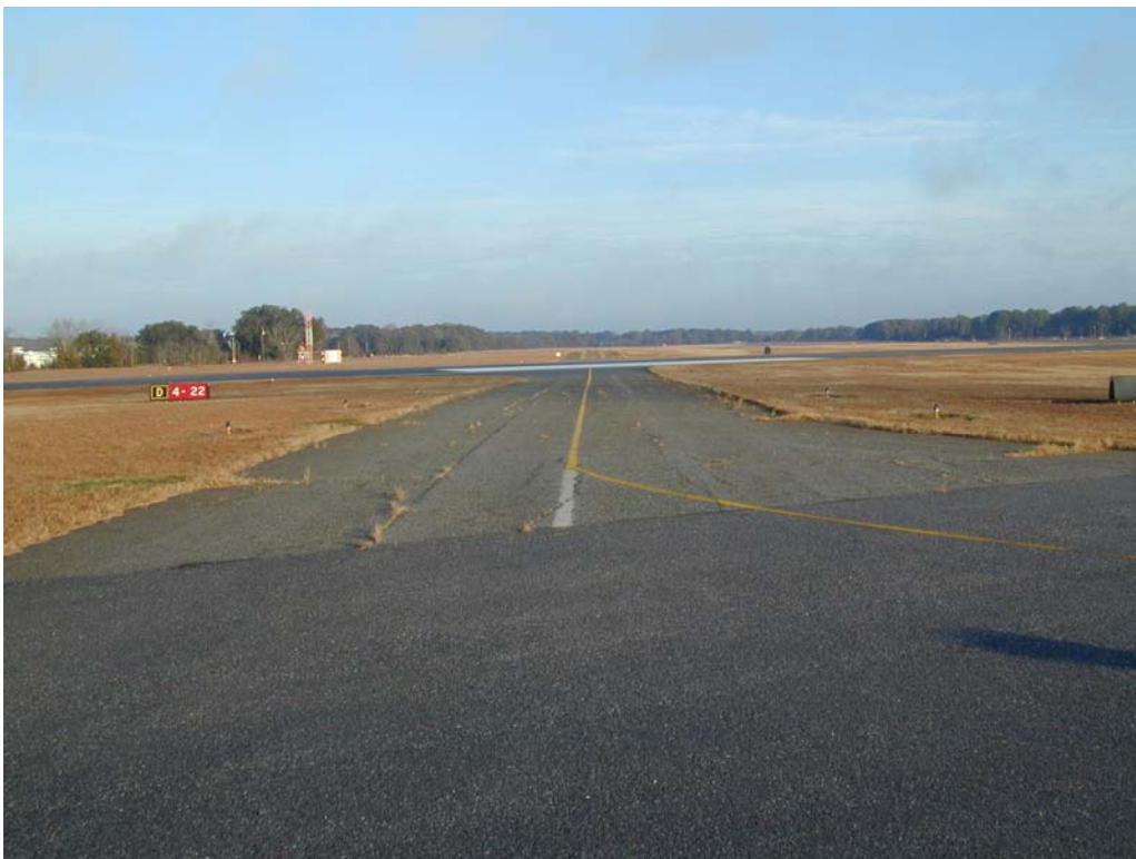
Overview of section TDAB-10.
