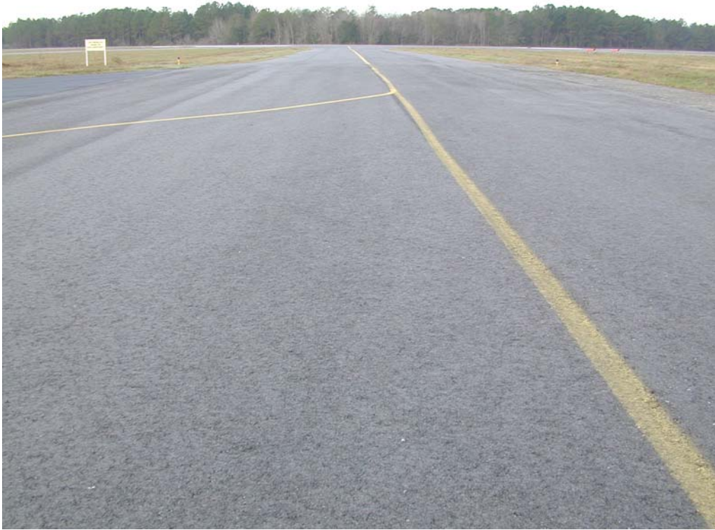
Taxiway A overview.
