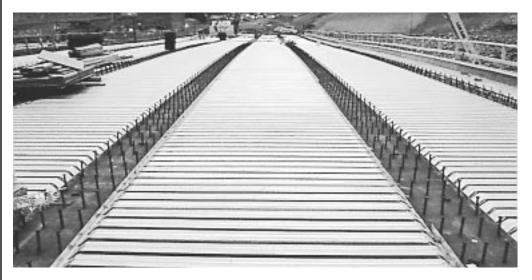
Another type of deck form that remains in place after the poured concrete has set is made of corrugated steel.
