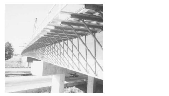
The pressure of the screed equipment and the weight of the concrete on the overhang pushes it against the bottom of the girder and out against its top flange at the same time. This could cause the girder to deform and the grade of the deck to be other than planned.
