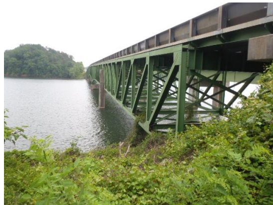
Truss system that will be repaired
