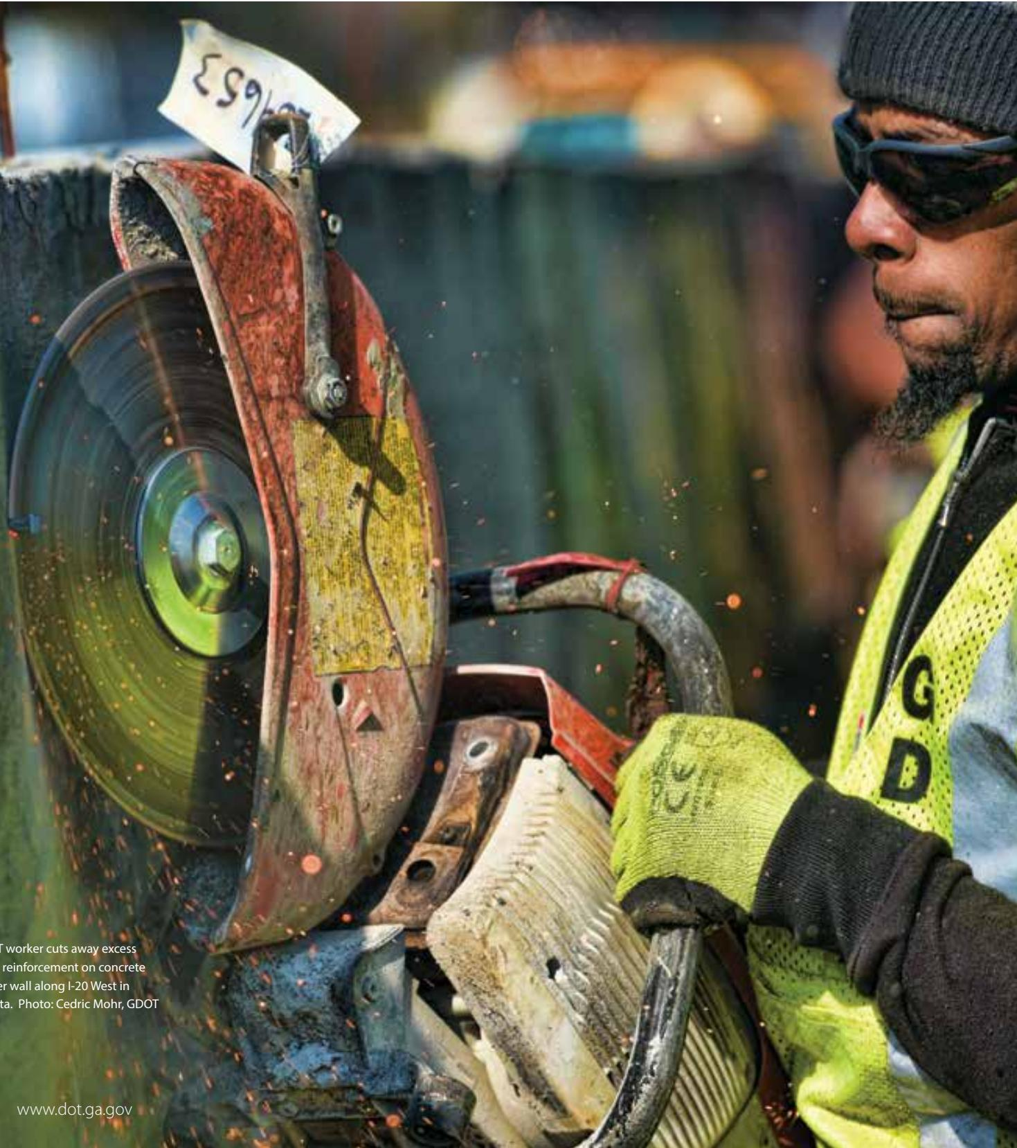
GDOT worker cuts away excess rebar reinforcement on concrete barrier wall along I-20 West in Atlanta. Photo: Cedric Mohr, GDOT
