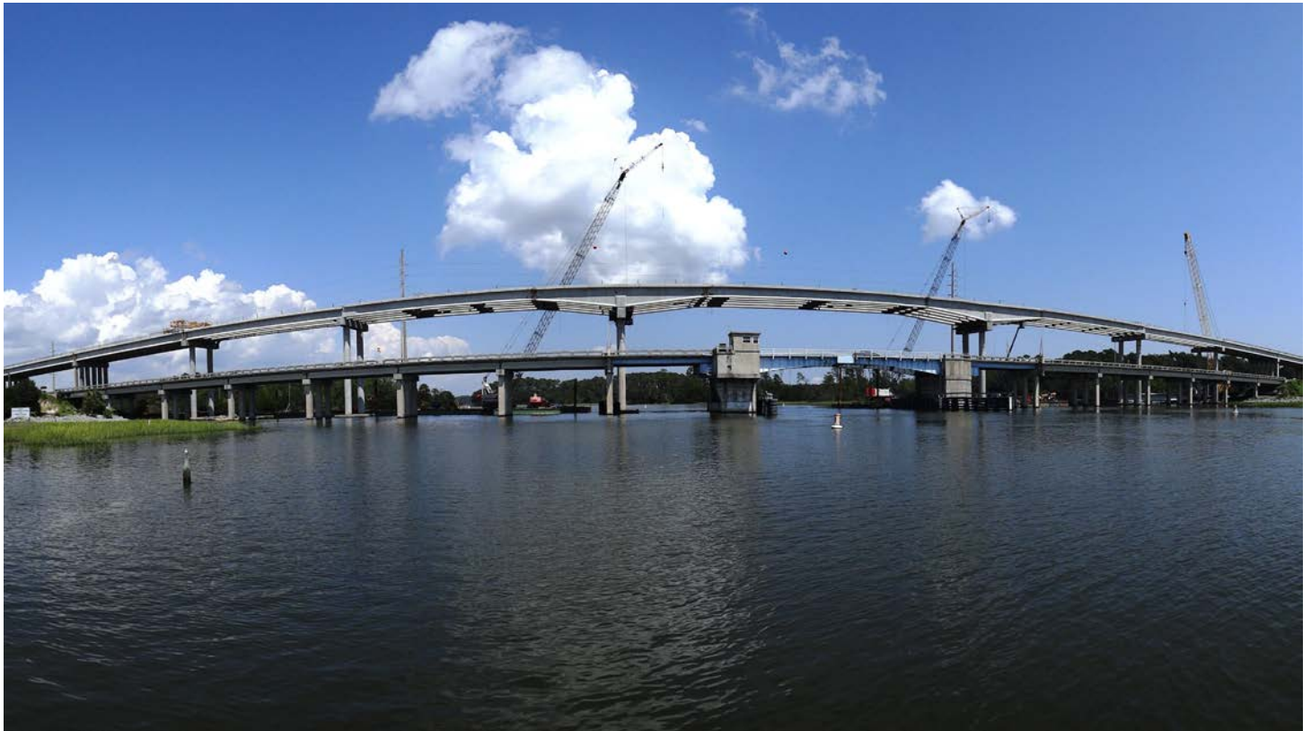
Skidaway Narrows bridge under construction with existing bridge in foreground
