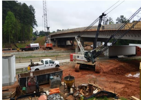
SR 316 at Walther Boulevard Grade Separation
