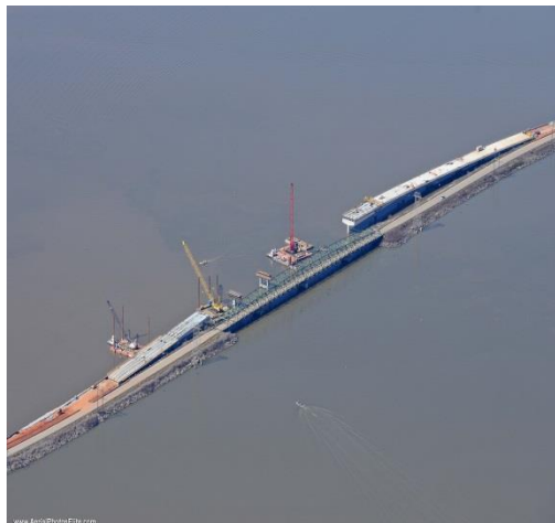
SR 47 at Little River Bridge Replacement
