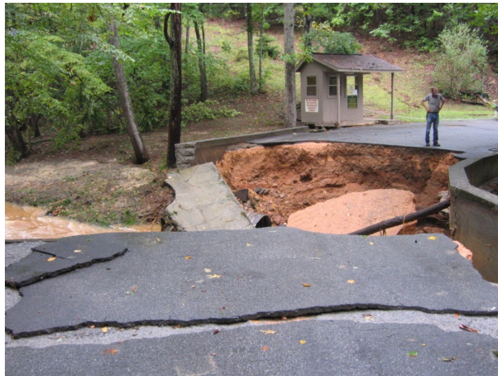
Tributary to Snake Creek, near Whitesburg, Georgia, showing a washed out bridge. Heavy rain caused flooding in and around the Atlanta area. (Photo from USGS)
