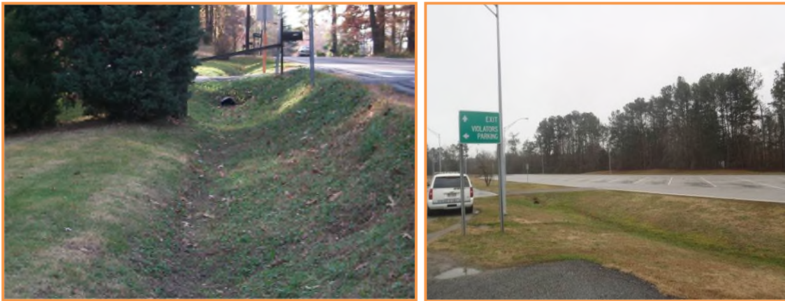
Figure 5.2-1 Two Examples of a Roadside Grass Channel
