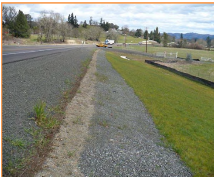
Figure 5.9-1 Bioslope with Gravel Diaphragm (photo courtesy of Oregon DOT)
