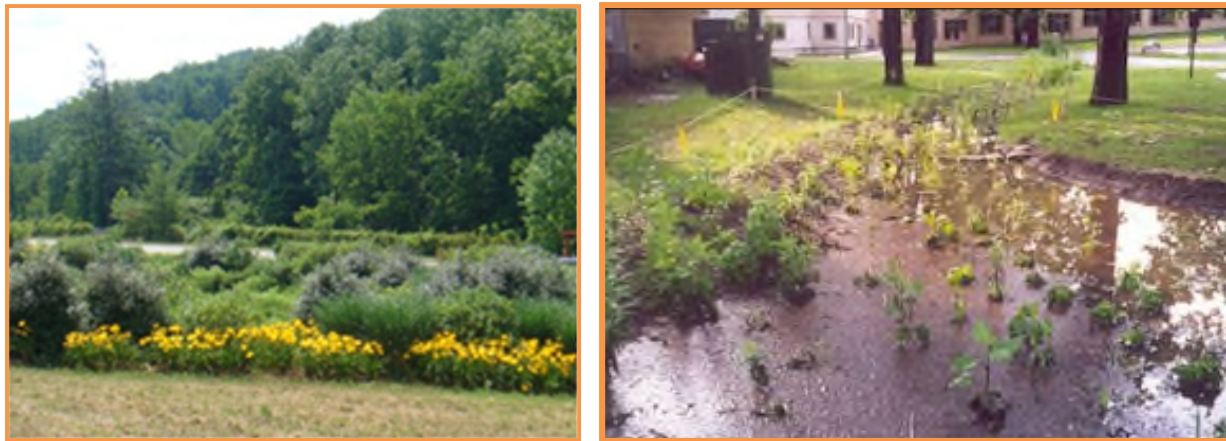
Figure 5.10-1 Landscaped Bioretention Basin (left) and Newly Planted Bioretention Basin after Storm Event (right) (photos courtesy of NCDOT and GSMM)
