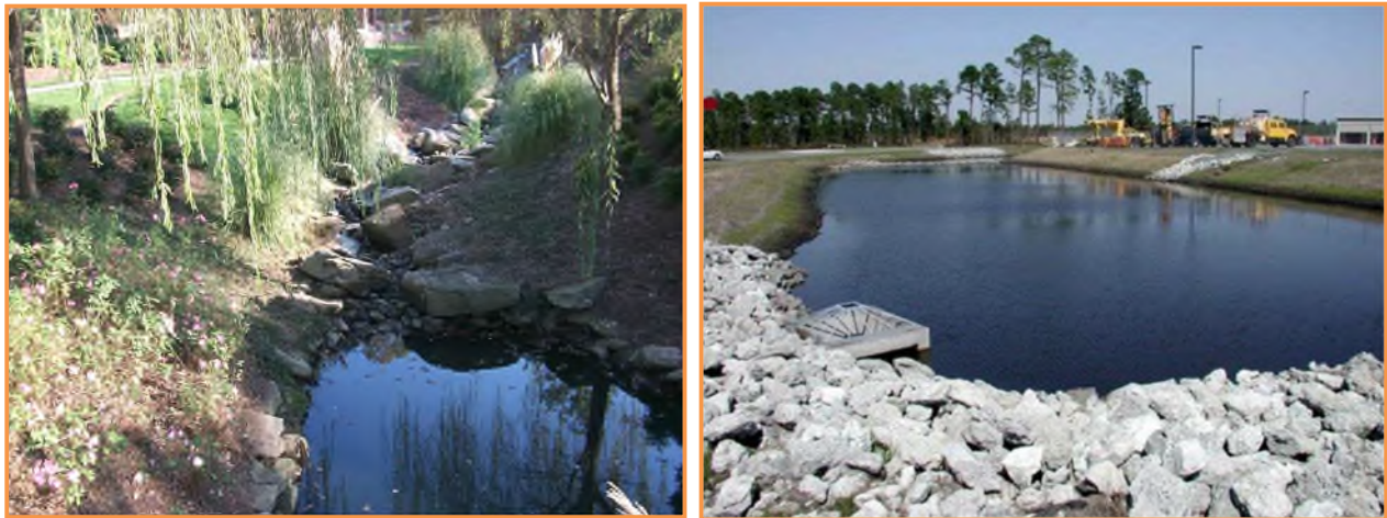
Figure 5.7-1 Wet Detention Pond as Part of a Conveyance Channel (left) and Wet Detention Pond at a DOT Maintenance Facility (right) (photos courtesy of GSMM and NCDOT)
