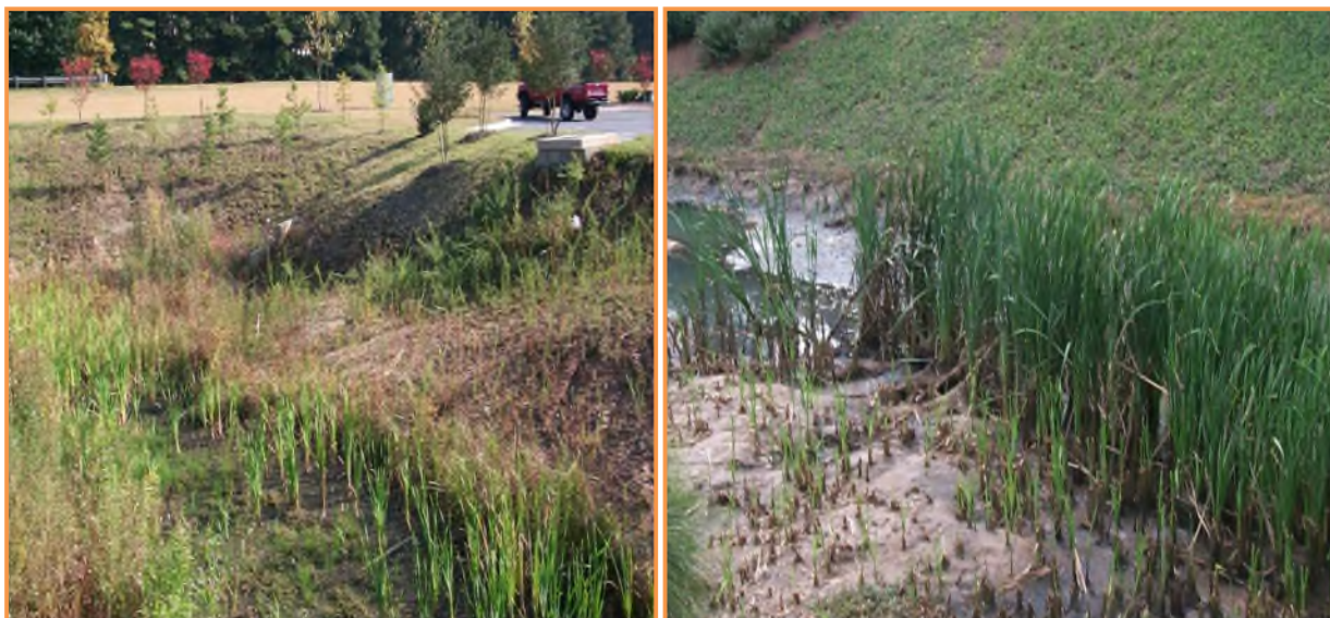
Figure 5.8-1 Shallow Stormwater Wetland (left) and Pocket Stormwater Wetland (right) (photos courtesy of GSMM)
