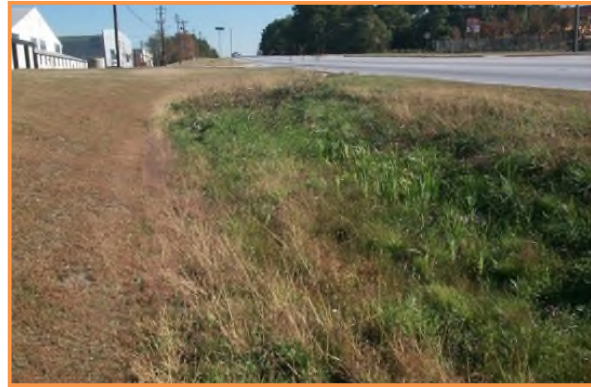
Figure 5.3-1 Examples of a Dry (left) and a Wet Swale (right) (source: Georgia Stormwater Management Manual [GSMM], Volume 2)
