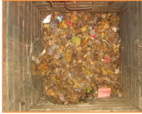
Figure 4.3-4 Sediment/Debris Buildup
