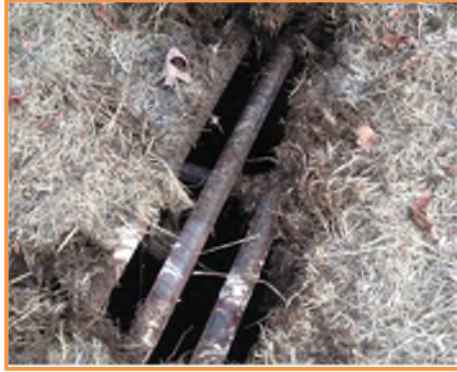
Figure 4.3-3 Grate Blockage
