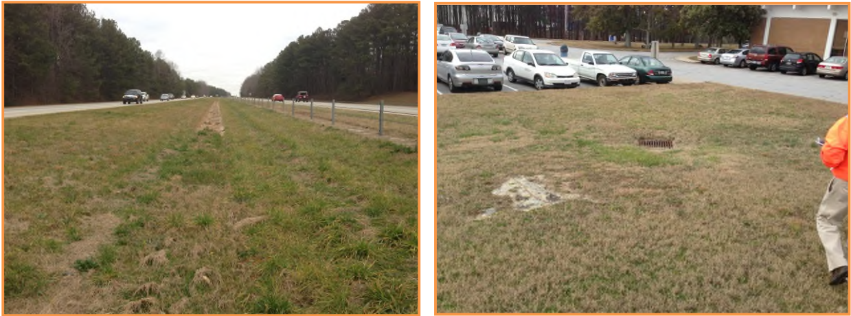
Figure 5.1-1 Channel between Filter Strip (left), Filter Strip around Drop Inlet (right),
