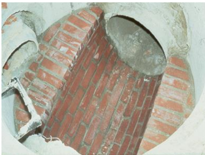
Figure 7.12 - Example of a bench in an access hole
