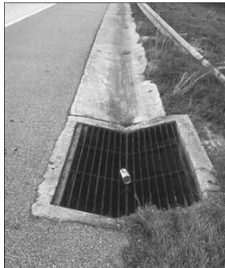
Figure 6.4 - Photograph of typical v-section gutter and inlet
