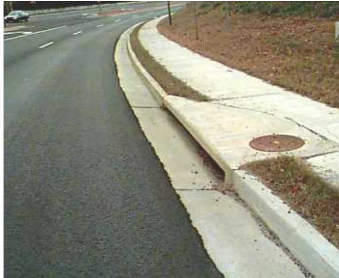
Figure 6.7 - Curb inlet placed on continuous roadway grade
