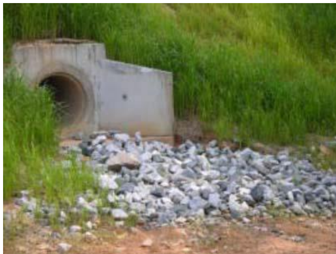
Figure 3.2 - Typical riprap energy dissipator (3-5)
