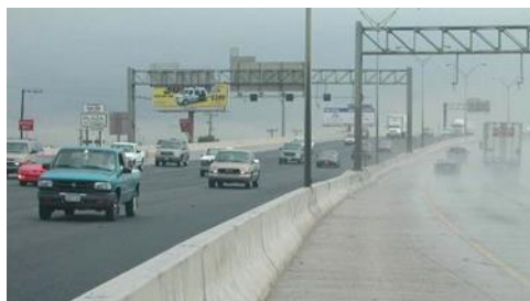
Photo Description: OGFC on Left, Portland Cement Concrete on Right
