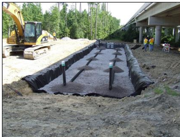
Figure 10.8-4 - Typical underdrain installation (photo courtesy of NCDOT)
