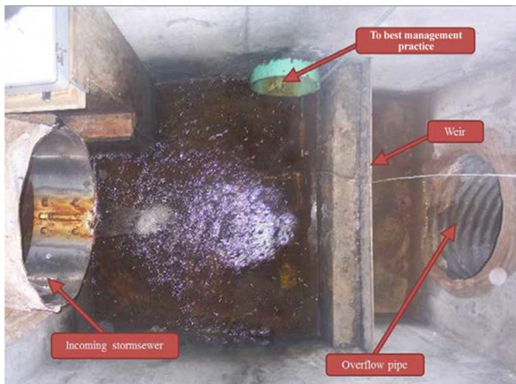
Figure 10.8-3 - A commonly used flow bypass structure configuration that bypasses flow when the capacity of the outlet pipe supplying the BMP is exceeded (photo courtesy of NCSU-BAE)
