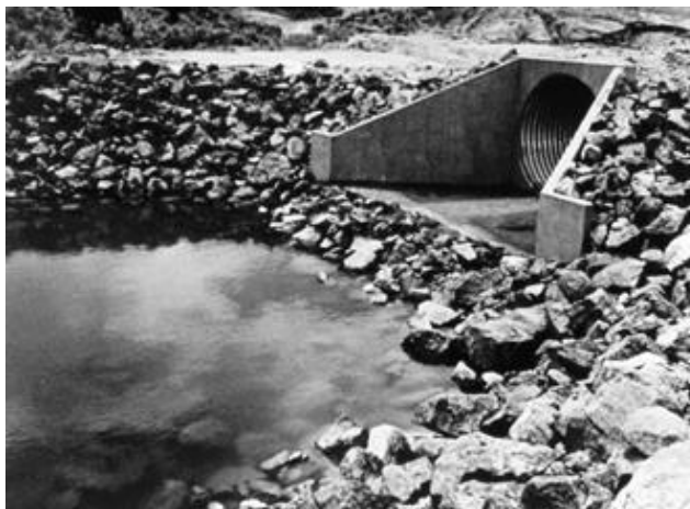
Figure 8.24 - Riprapped culvert energy basin
