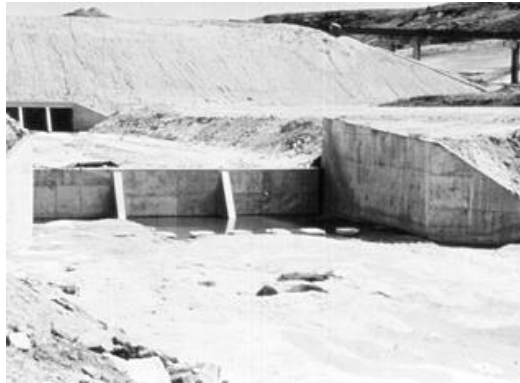
Figure 8.22 - Straight drop spillway stilling basin
