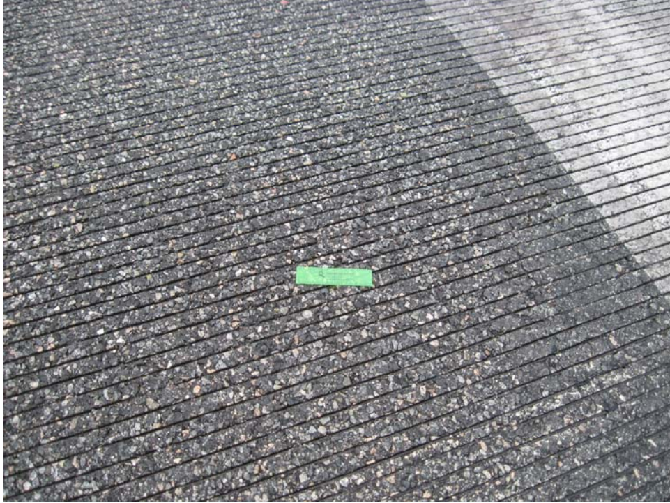
R422VL-10. Weathering (sample unit #55).
