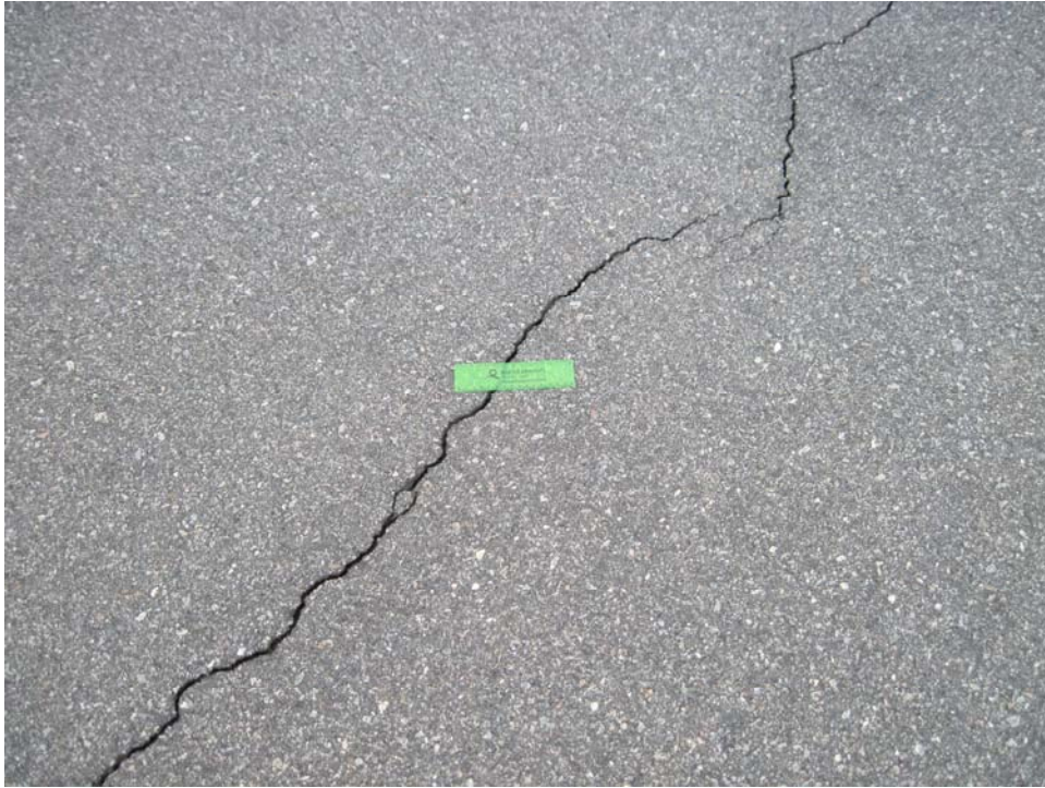
A01VL-20. Longitudinal and Transverse Cracking (Sample Unit #16).
