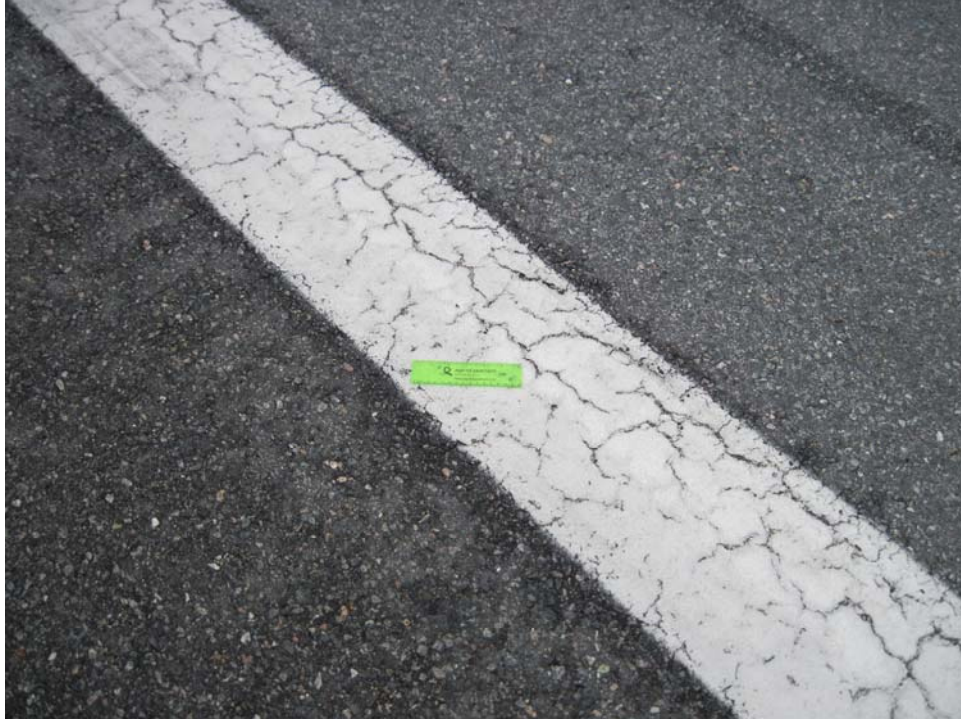
R1331VL-20. Satisfactory Paint.
