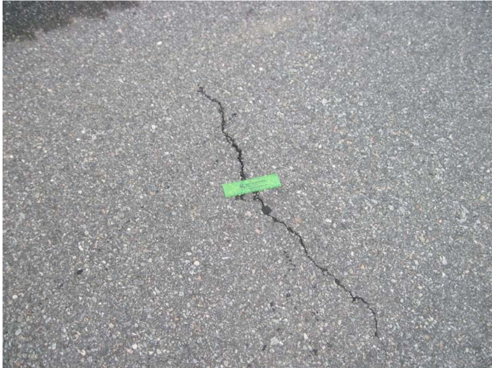
TLVL-10. Longitudinal and Transverse Cracking.
