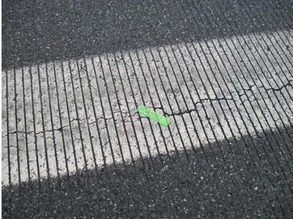
R422VL-10. Longitudinal and Transverse Cracking.
