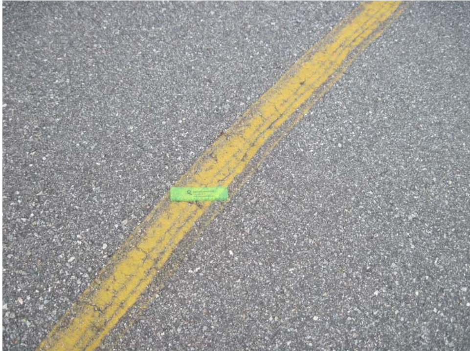
THANG02VL-20. Unsatisfactory Paint.
