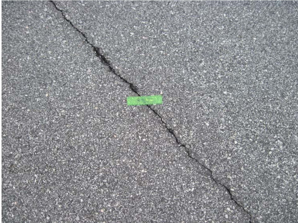
TAVL-20. Longitudinal and Transverse Cracking (Sample Unit #2).
