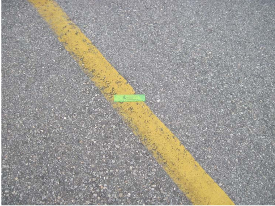
THANG01VL-30. Satisfactory Paint.
