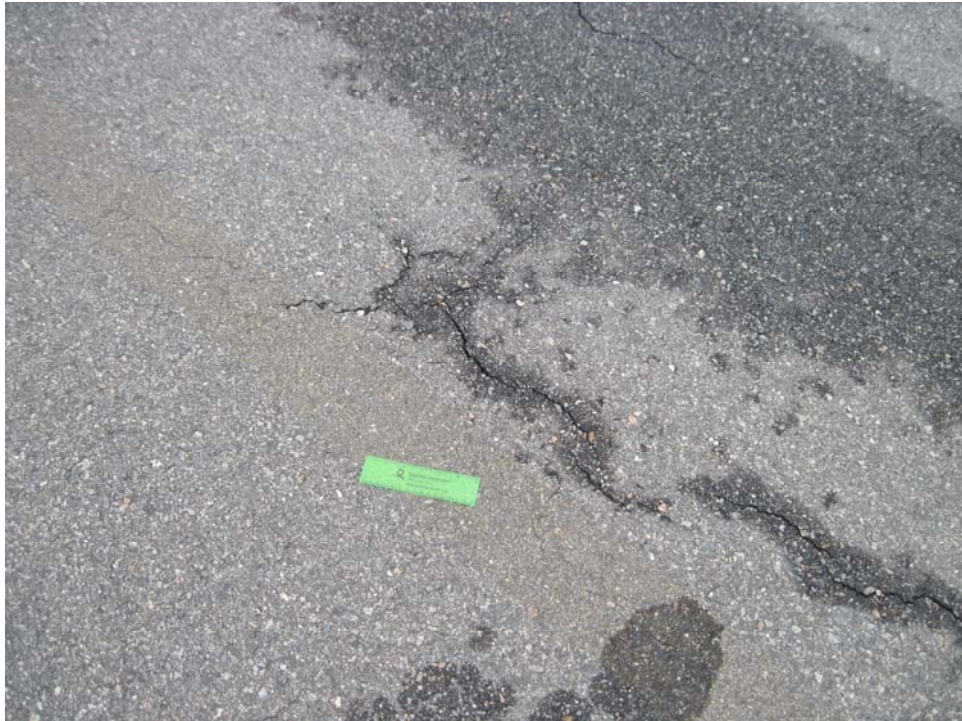
A01VL-10. Longitudinal and Transverse Cracking (Sample Unit #13).
