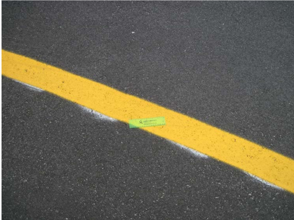
THANG02VL-40. Satisfactory Paint.
