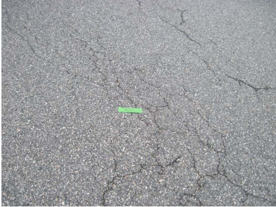
TMVL-10. Alligator Cracking (sample unit #2).
