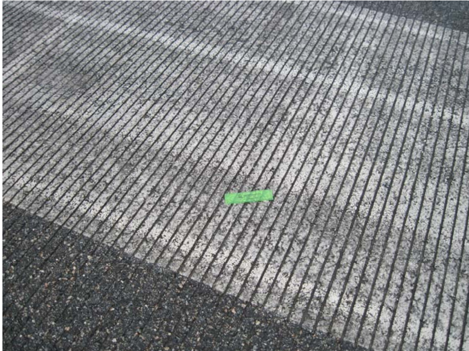
R422VL-10. Unsatisfactory Paint.
