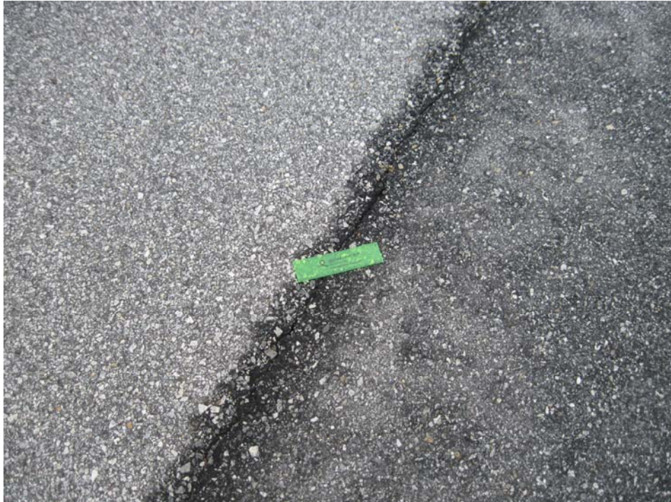
TCVL-10. Longitudinal and Transverse Cracking (sample unit #30).
