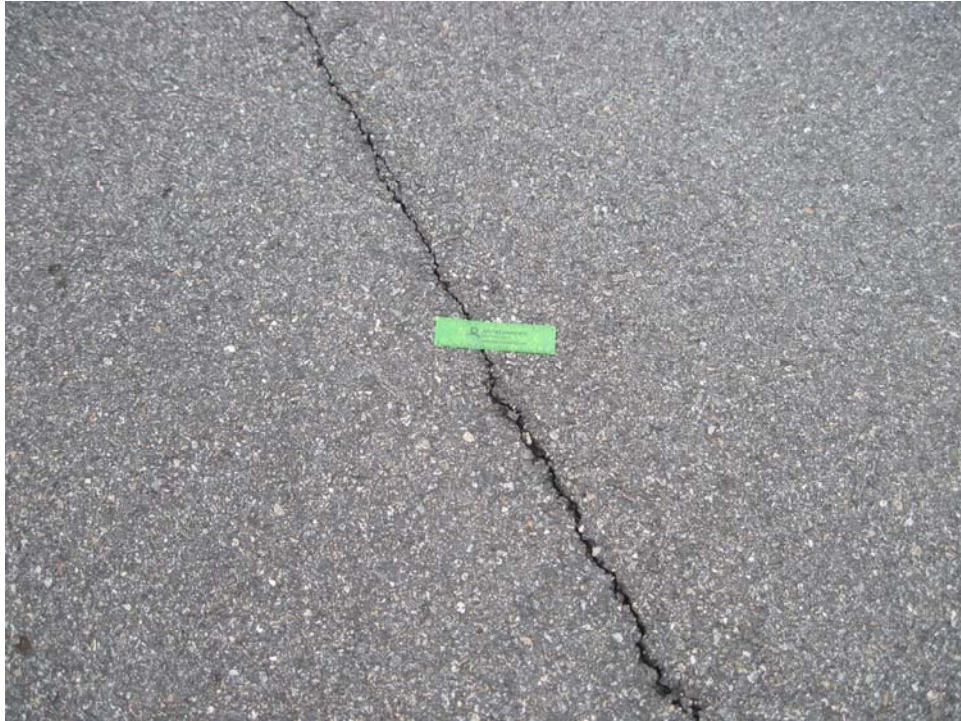
TAVL-10. Longitudinal and Transverse Cracking (Sample Unit #20).
