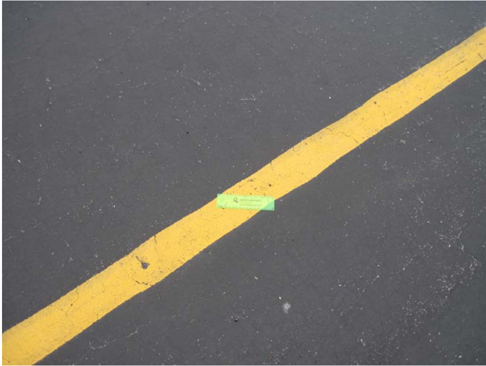
A01VL-10. Satisfactory Paint.
