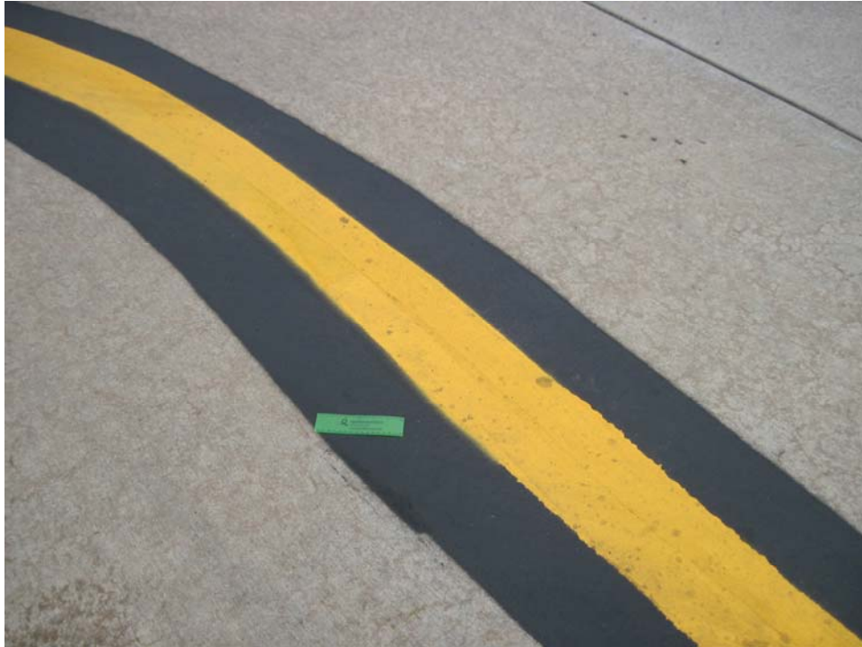
ATERMVL-10. Satisfactory Paint.
