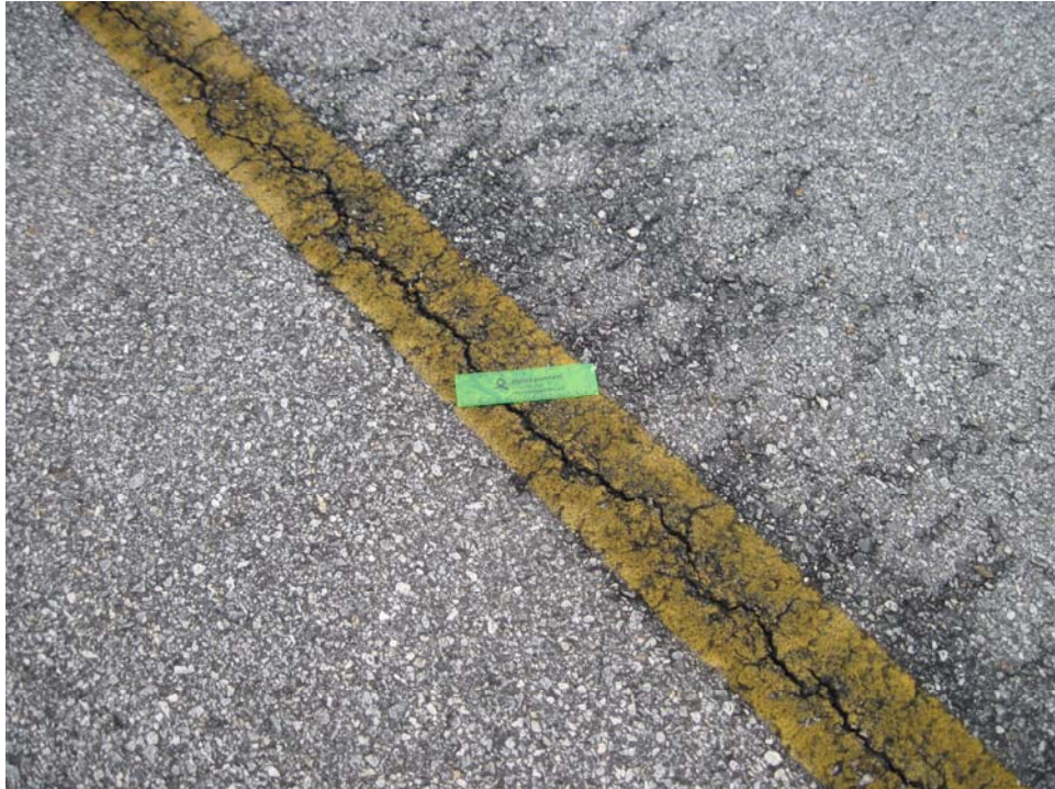
TFVL-10. Unsatisfactory Paint and Longitudinal and Transverse Cracking (Sample Unit #3).
