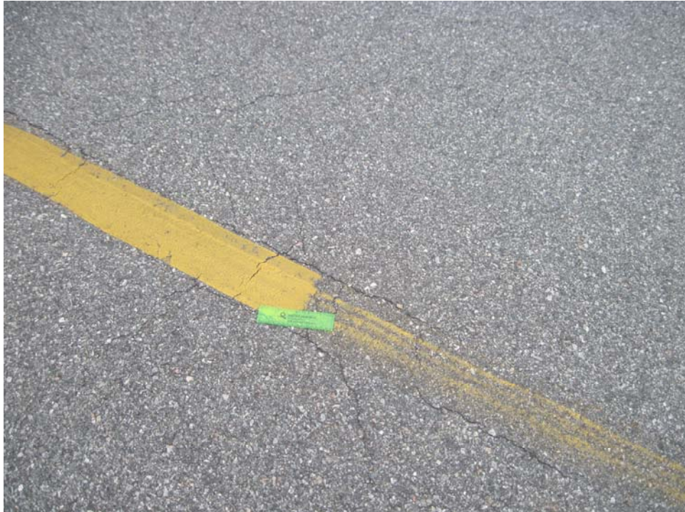
A01VL-40. Satisfactory Paint.
