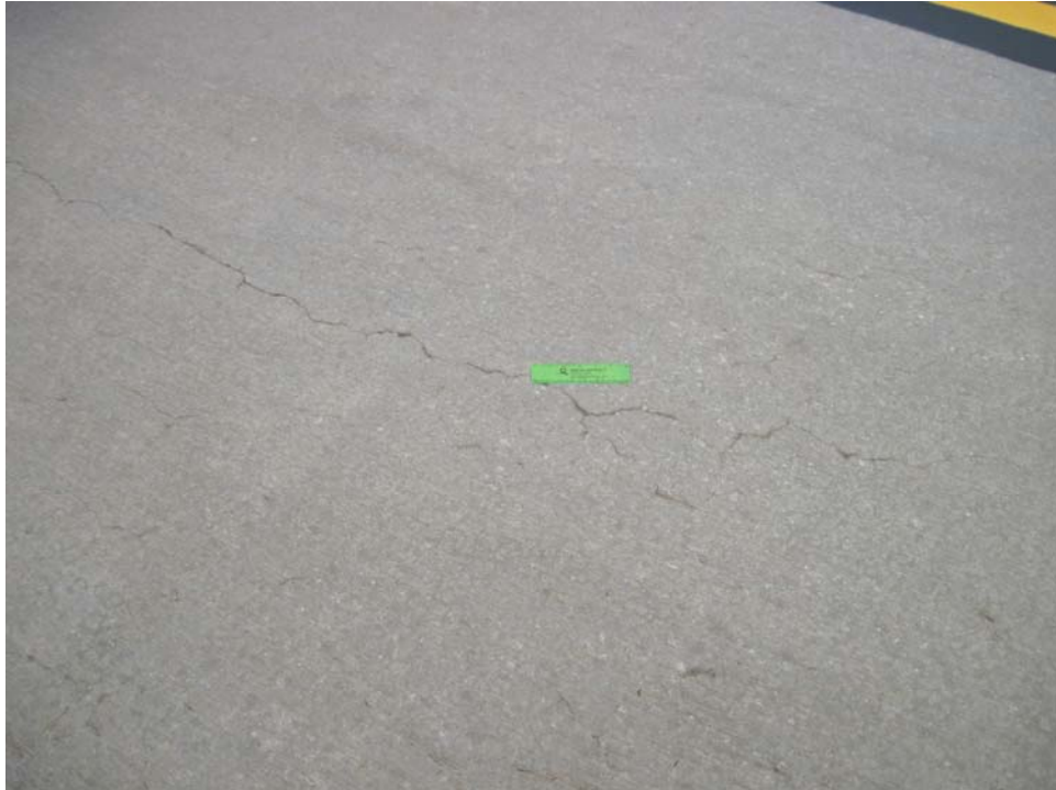
ATERMVL-10. Shrinkage Cracking (Sample Unit #5).
