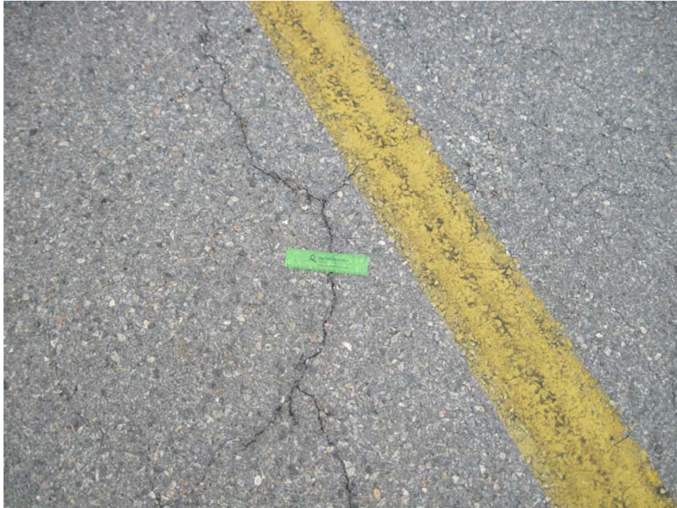
THANG02VL-10. Longitudinal and Transverse Cracking (Sample Unit #02).
