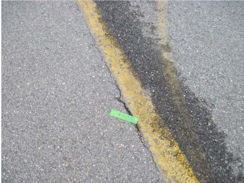
THANG01VL-30. Longitudinal and Transverse Cracking (Sample Unit #01).
