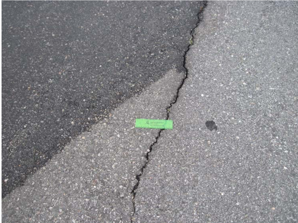
A01VL-30. Longitudinal and Transverse Cracking (Sample Unit #01).
