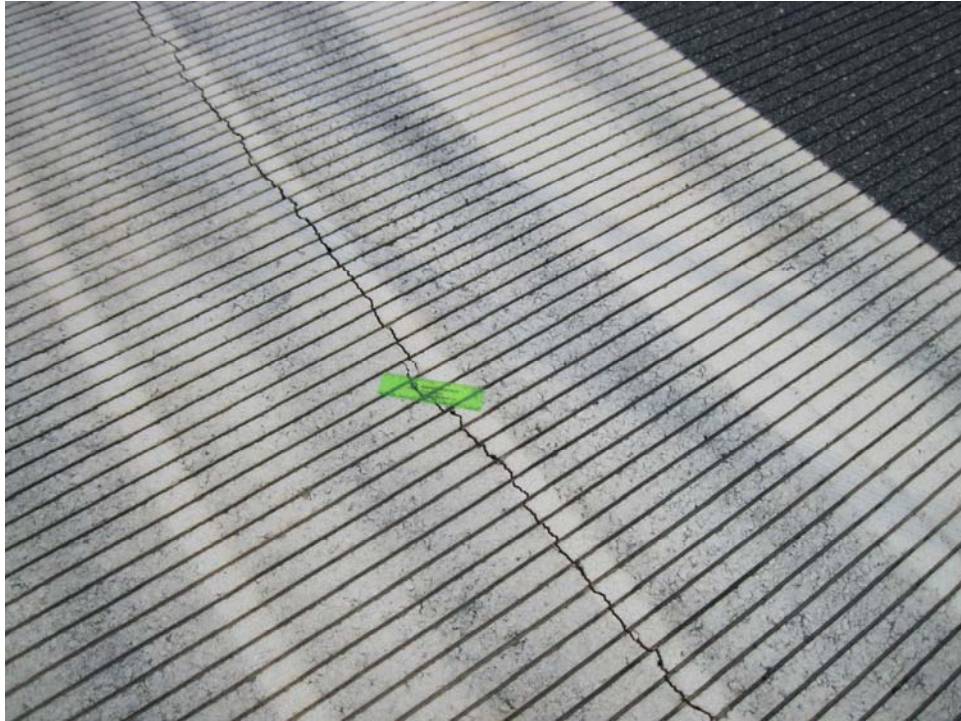
R1735VL-10. Longitudinal and Transverse Cracking and Satisfactory Paint (Sample Unit #60).
