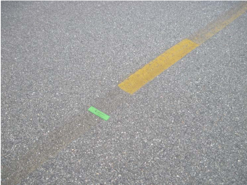
A01VL-20. Unsatisfactory Paint.
