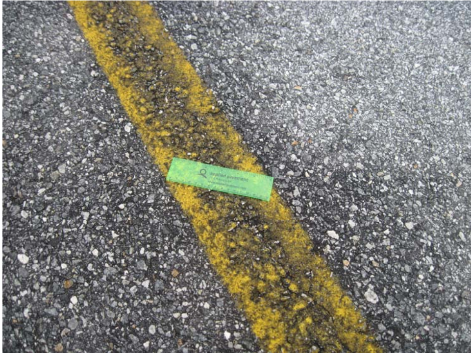
TCVL-10. Unsatisfactory Paint.
