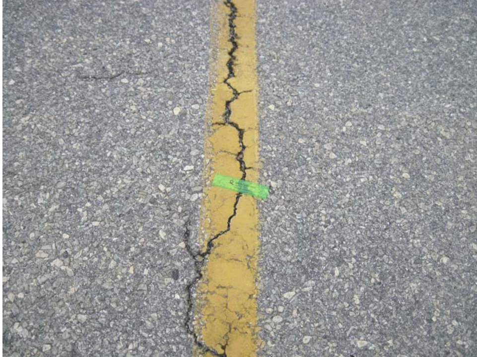
THANG01VL-10. Longitudinal and Transverse Cracking and Satisfactory Paint (Sample Unit #1).
