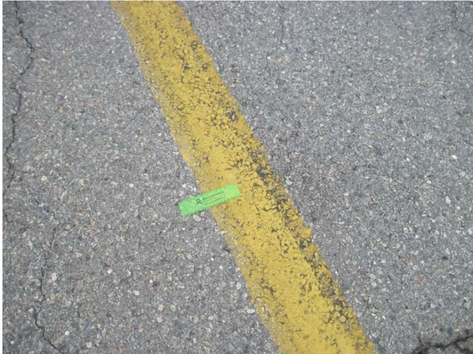
THANG02VL-10. Satisfactory Paint.
