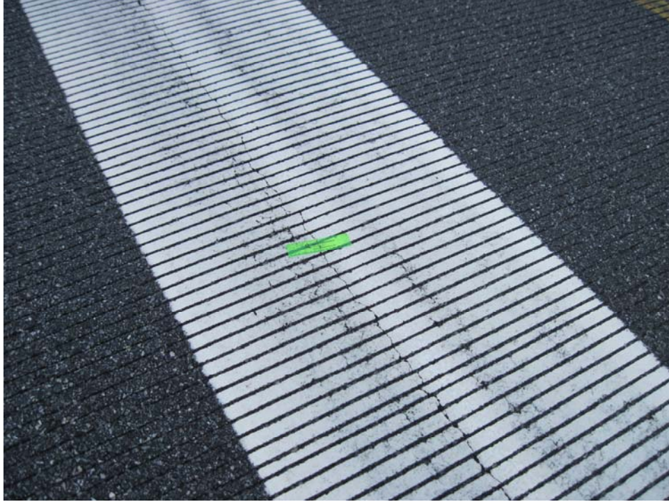
R1735VL-20. Longitudinal and Transverse Cracking and Satisfactory Paint (Sample Unit #31).
