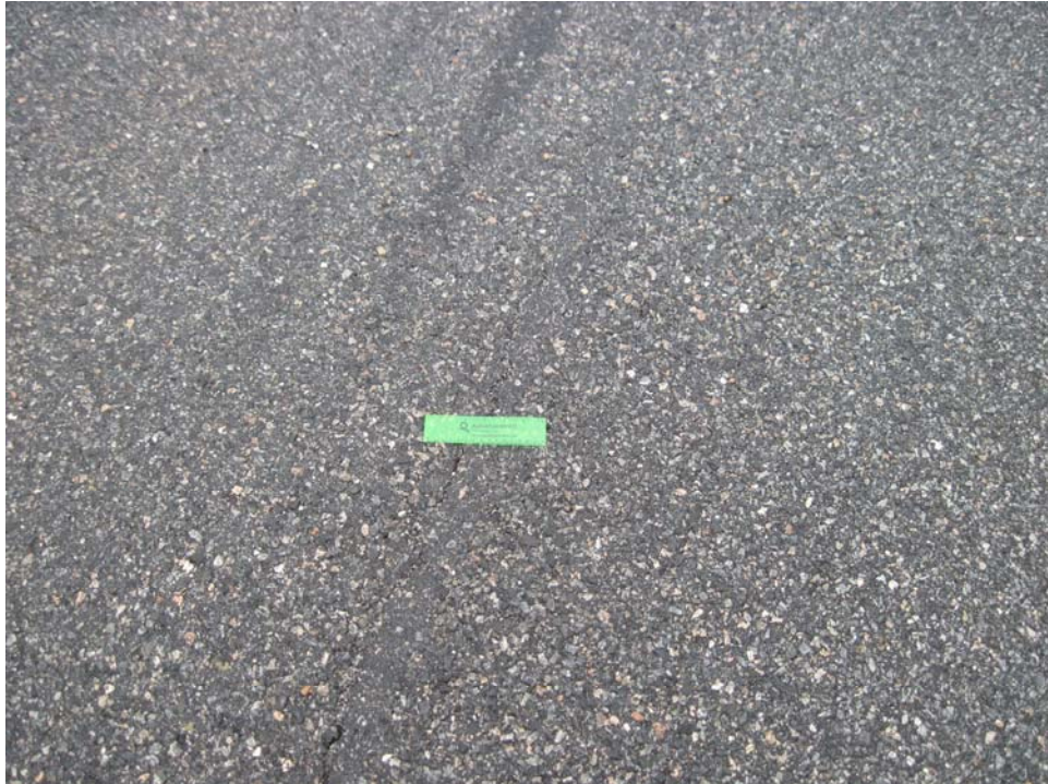
R1331VL-20. Longitudinal and Transverse Cracking.
