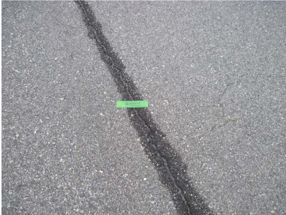
A01VL-40. Longitudinal and Transverse Cracking (Sample Unit #2).
