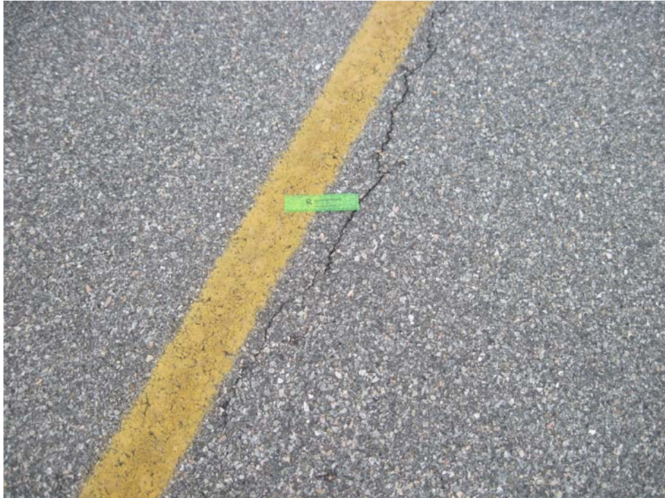
TMVL-10. Longitudinal and Transverse Cracking and Satisfactory Paint (Sample Unit #9).
