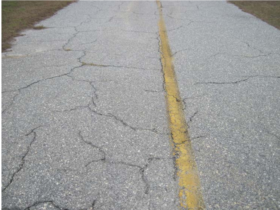
THANG01VL-10. Block Cracking (Sample Unit #02).
