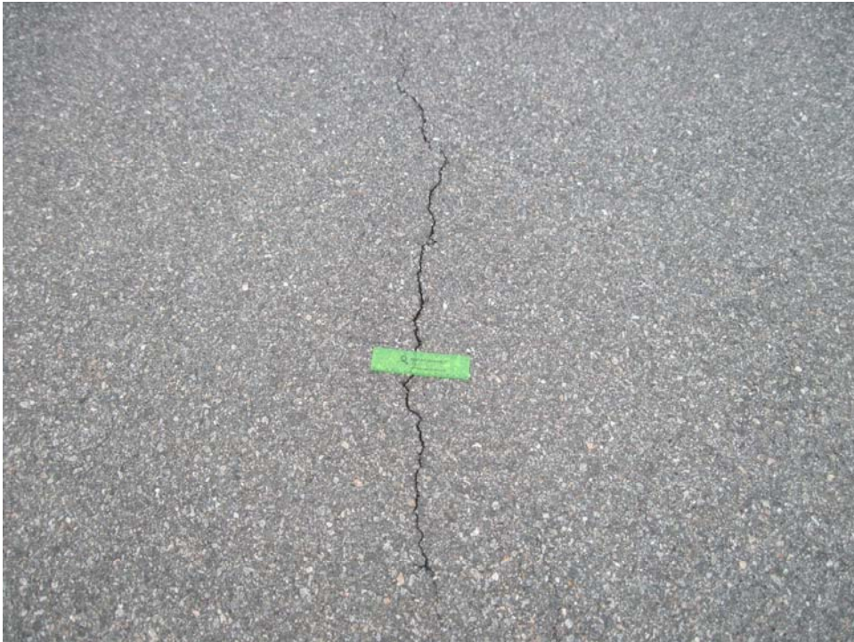
A01VL-25. Longitudinal and Transverse Cracking (Sample Unit #02).
