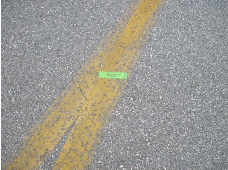
THANG01VL-20. Satisfactory Paint.
