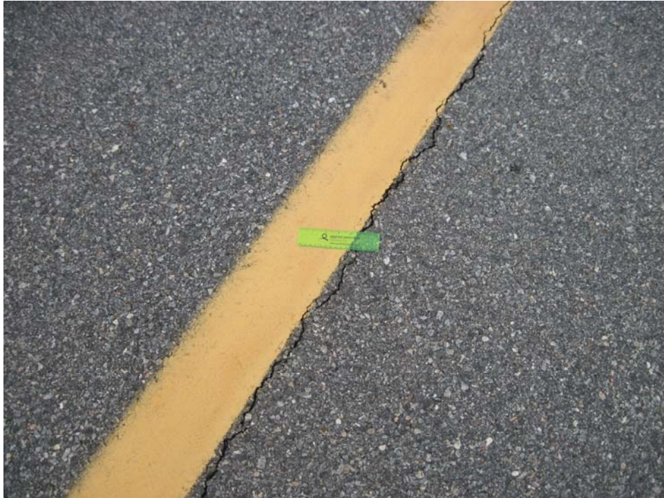
TNVL-10. Longitudinal and Transverse Cracking and Satisfactory Paint.
