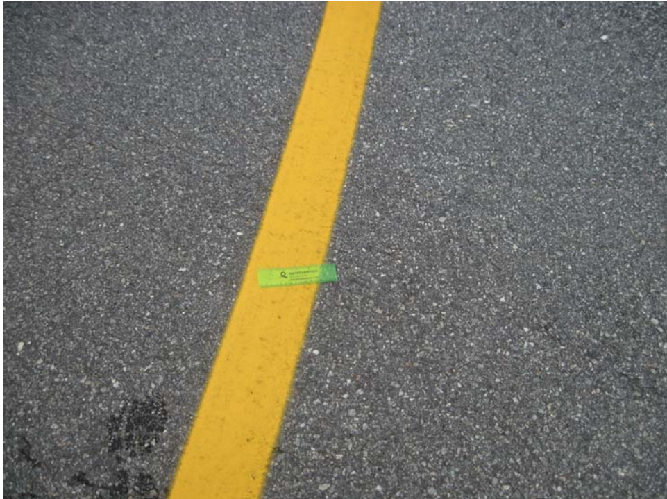
THANG02VL-30. Satisfactory Paint.
