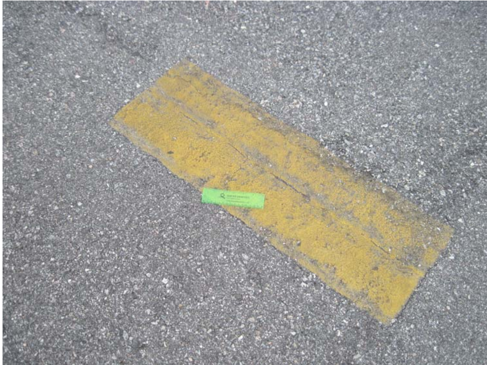
A01VL-30. Unsatisfactory Paint.
