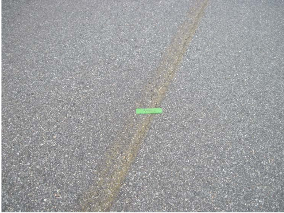
TLVL-20. Longitudinal and Transverse Cracking and Unsatisfactory Paint (Sample Unit #2).
