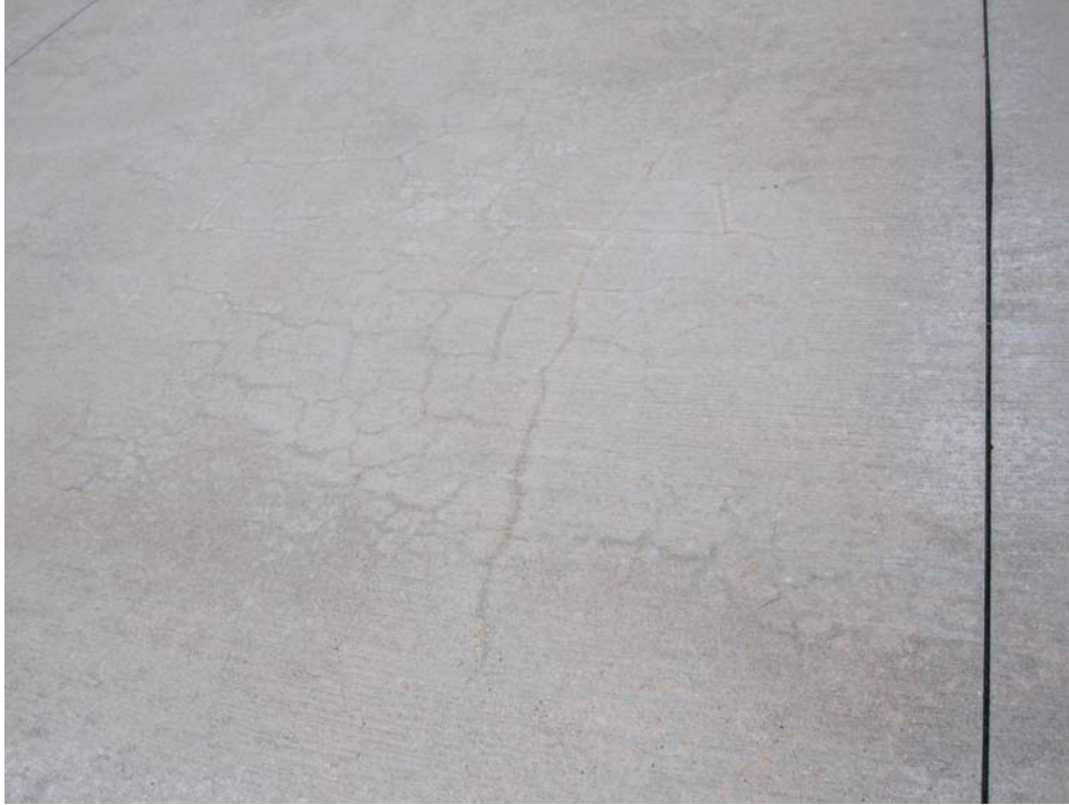
TESV-10. Shrinkage Cracking (Sample Unit #09).
