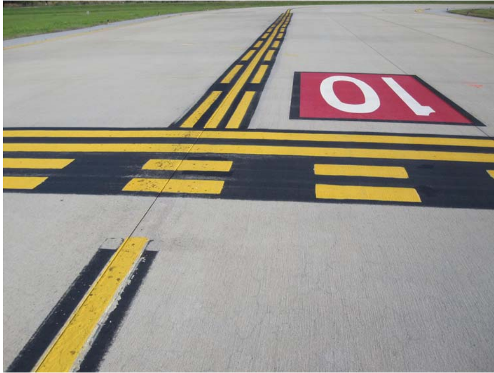
TESV-10. Satisfactory Paint (2).
