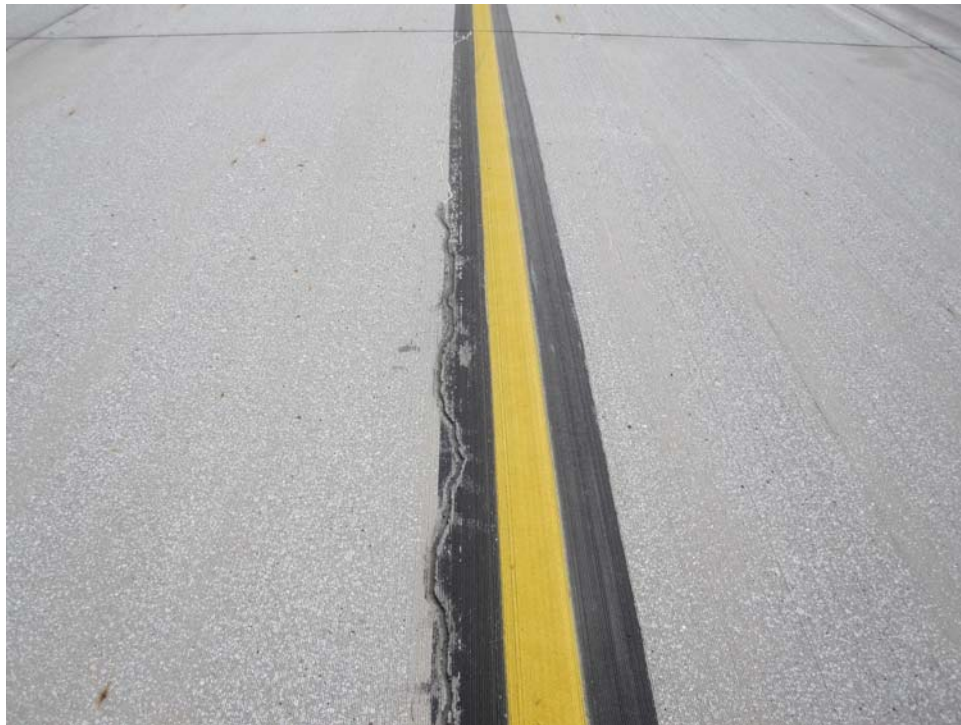
TESV-40. LTD Cracking (Sample Unit #16).
