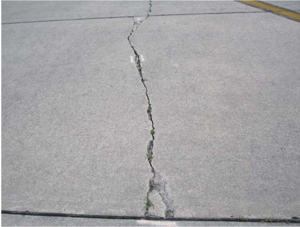
ASIGSTHSV-10. LTD Cracking (Sample Unit #02).
