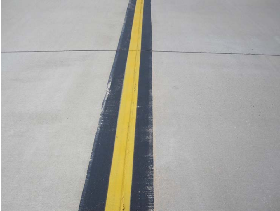
TGA5SV-10. Satisfactory Paint.
