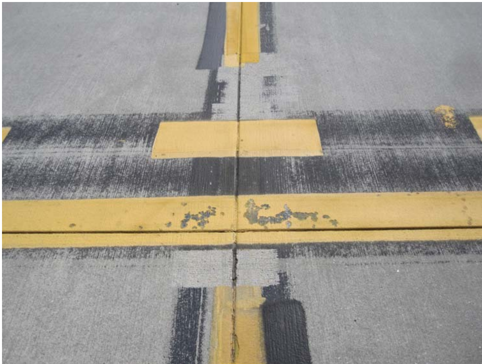
TA1SV-10. Satisfactory Paint.
