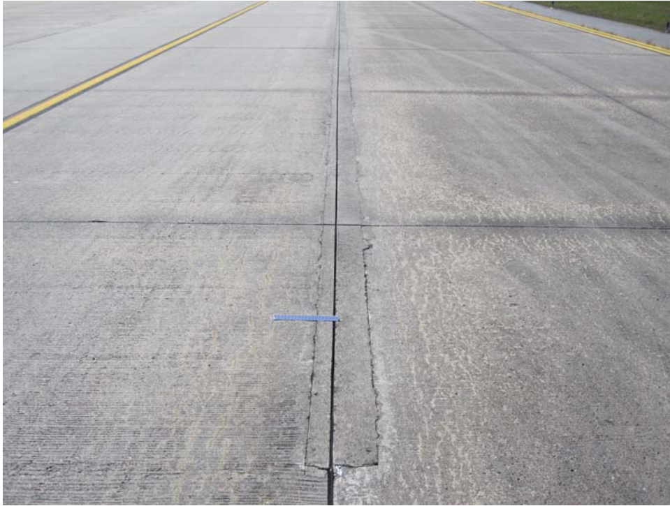
TBSV-20. Large Patching (Sample Unit #71).
