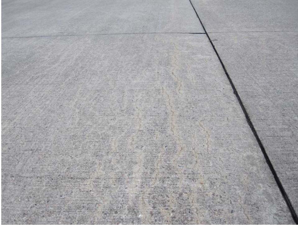
TCSV-40. ASR (Sample Unit #15).
