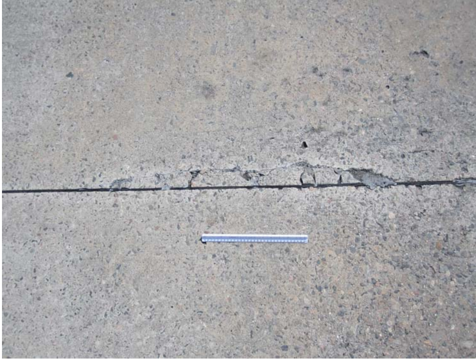
ATERMSV-10. Joint Spalling (Sample Unit #33).
