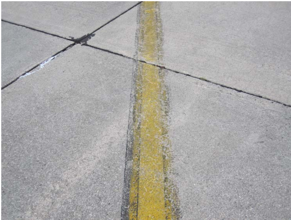
ASIGSTHSV-10. Unsatisfactory Paint.
