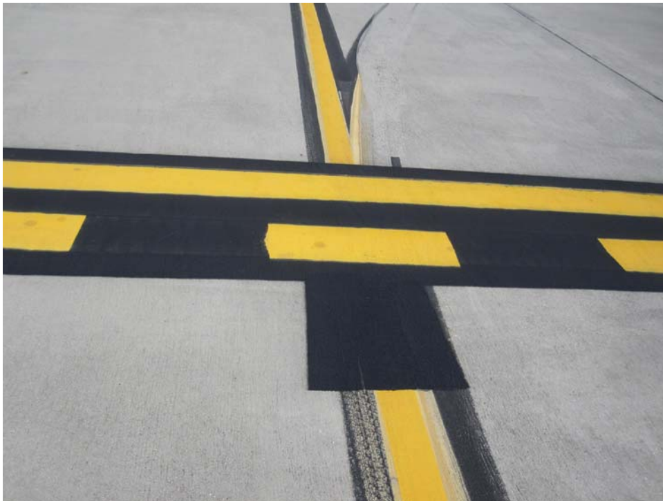
TGA1SV-10. Satisfactory Paint.
