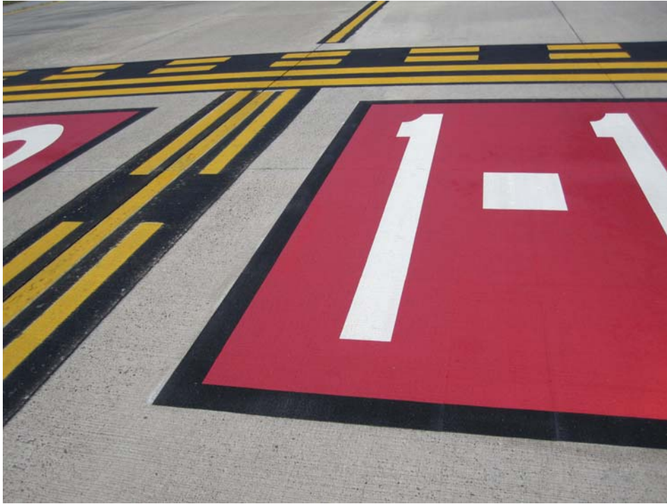
TESV-30. Satisfactory Paint.
