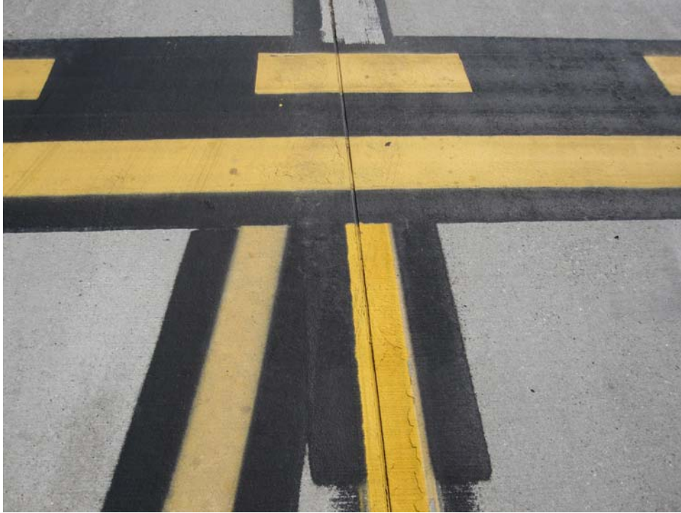
TA3SV-10. Satisfactory Paint.
