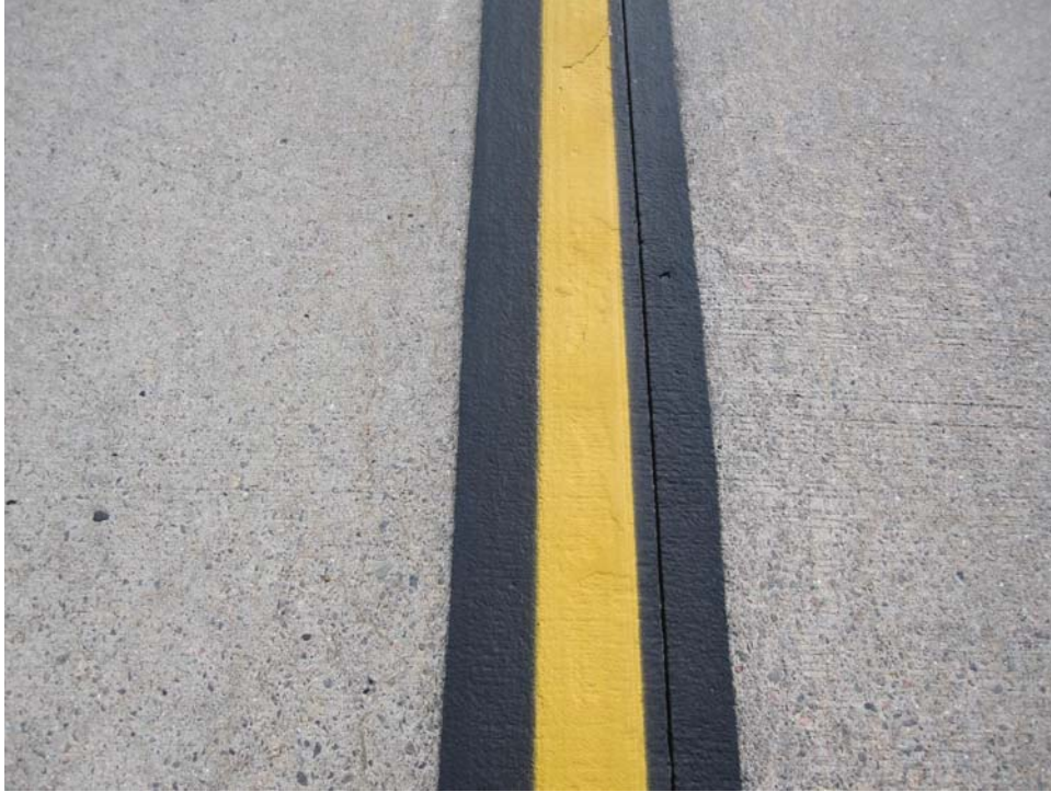
TCSV-40. Satisfactory Paint.
