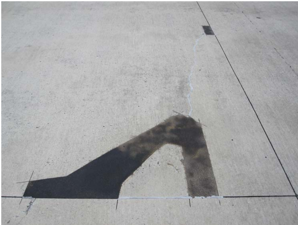
TC1SV-10. Longitudinal and Transverse Cracking (Sample Unit #25).
