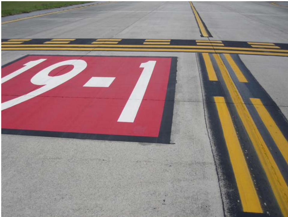
TCSV-20. Satisfactory Paint.
