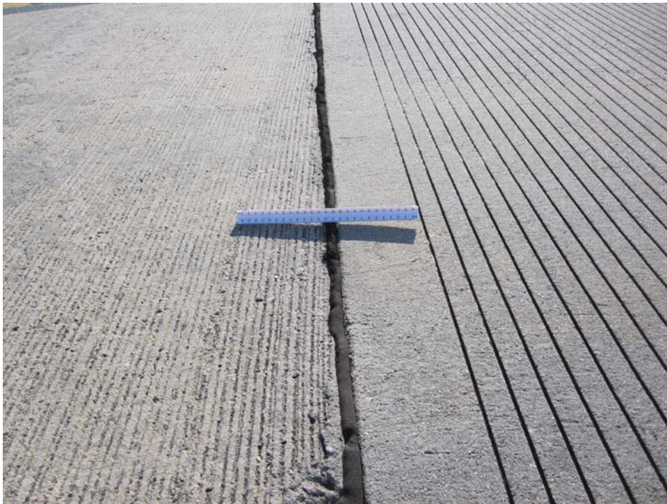
R119SV-20W. Joint Seal Damage (Sample Unit #01).
