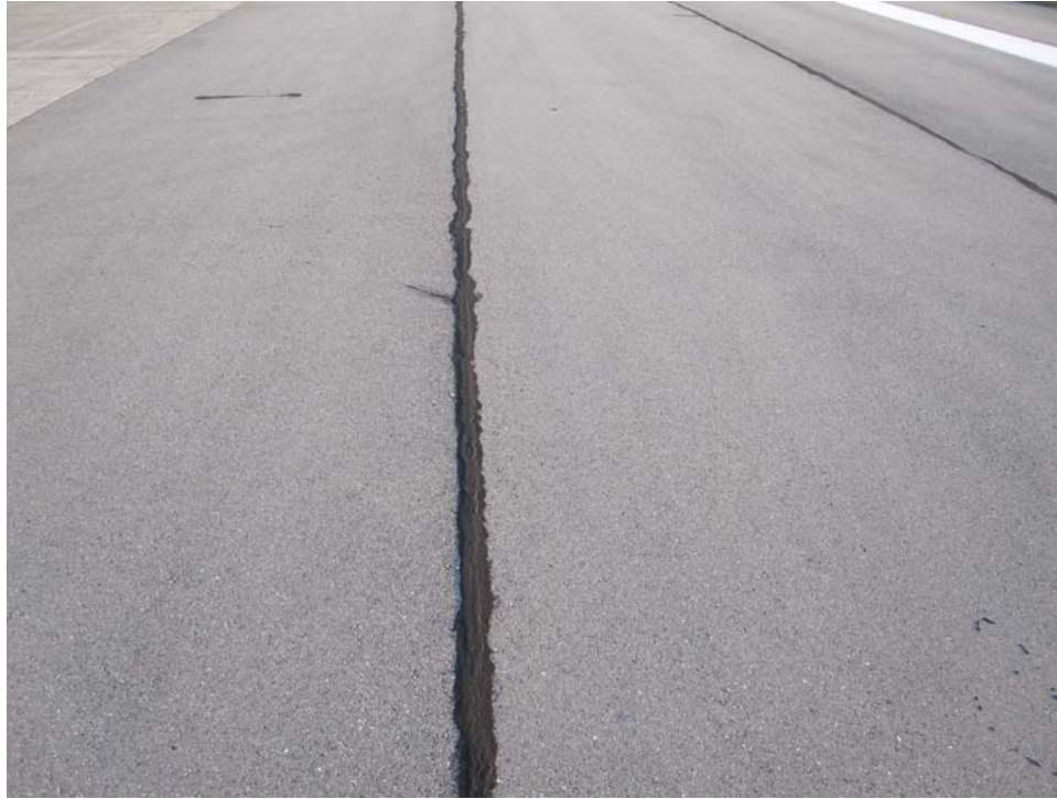
R119SV-10E. Longitudinal and Transverse Cracking (Sample Unit #24).
