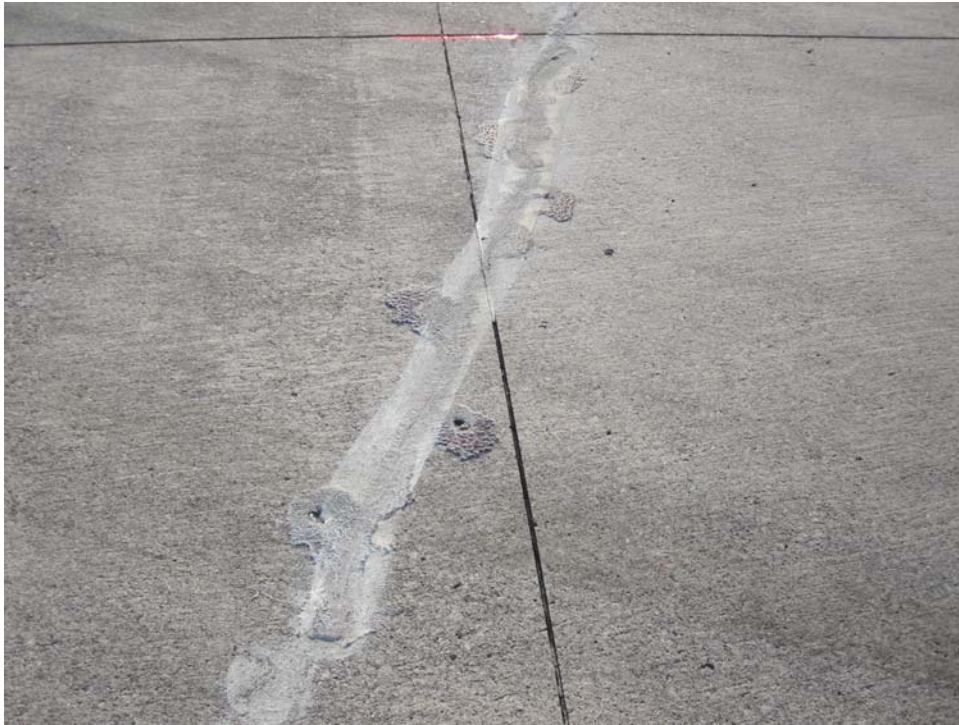
TC1SV-10. Corner Break (Sample Unit #06).
