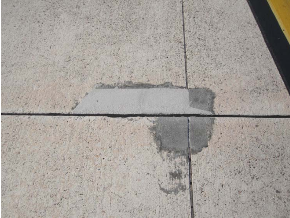
TE1SV-10. Small Patching (Sample Unit #09).
