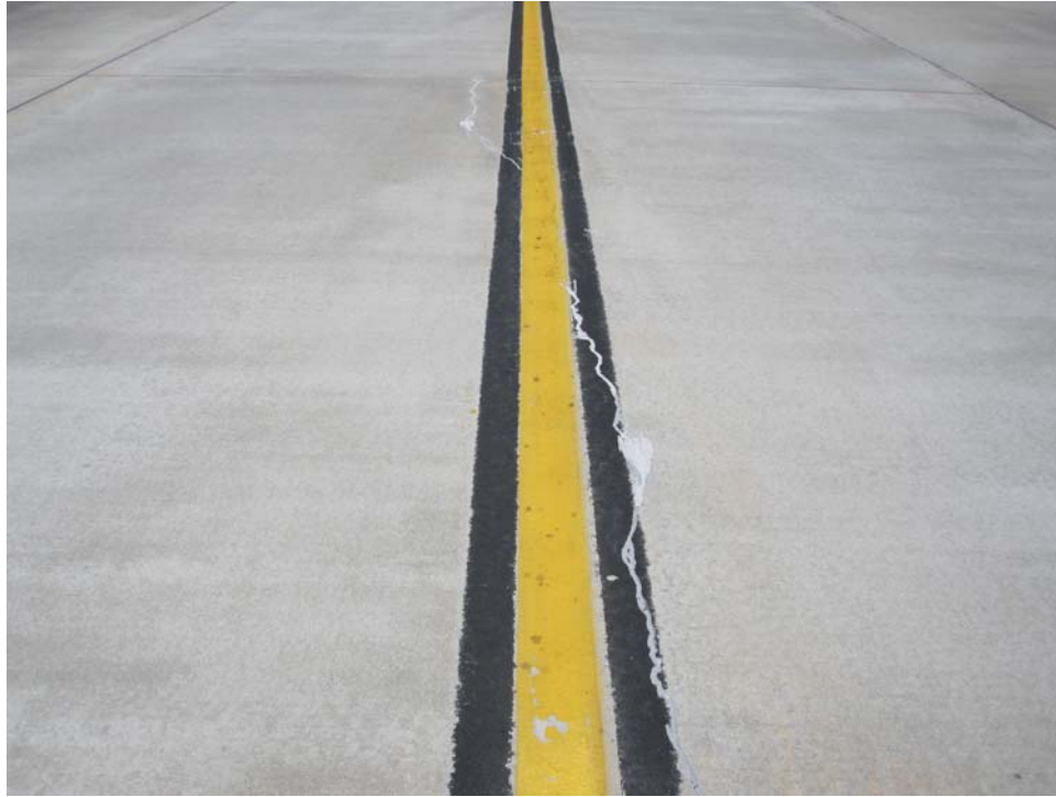
TFSV-10. LTD Cracking (Sample Unit #13).
