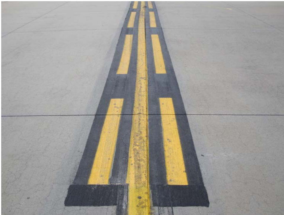
TESV-10. Satisfactory Paint (1).
