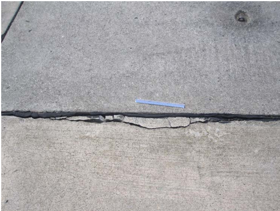
ASIGSTHSV-10. Joint Spalling (Sample Unit #16).
