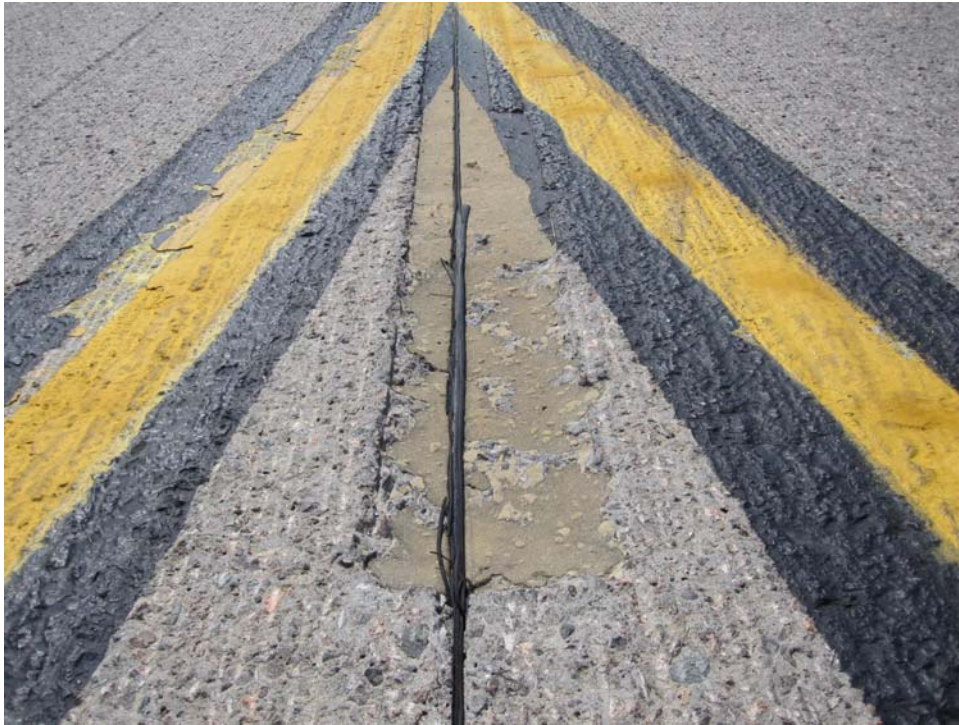
TE1SV-10. Large Patching (Sample Unit #03).
