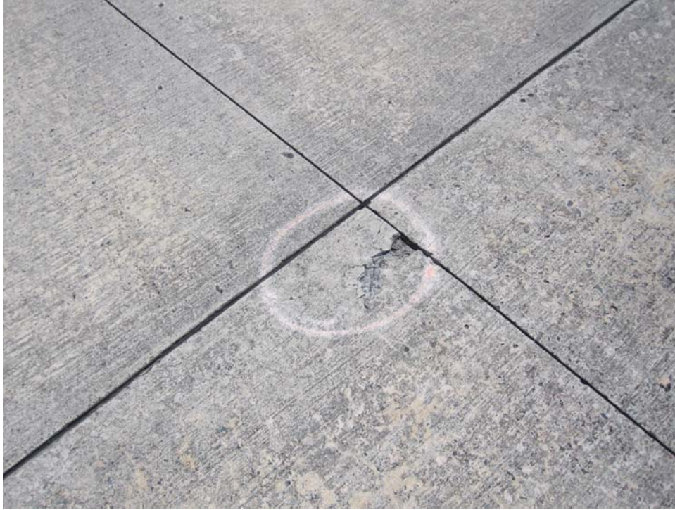
AOLDTERMSV-10 . Corner Spalling (Sample Unit #72).
