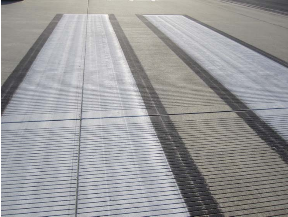
R1028SV-10C. Satisfactory Paint.
