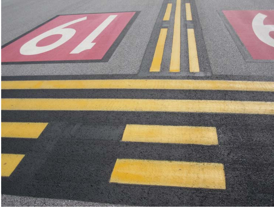
TBSV-10. Satisfactory Paint.
