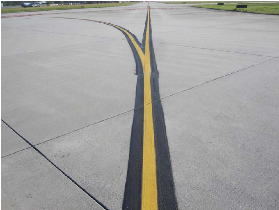
TE2SV-10. Satisfactory Paint.
