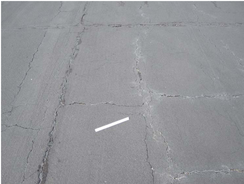
ASIGSTHSV-20. Block Cracking (Sample Unit #15).
