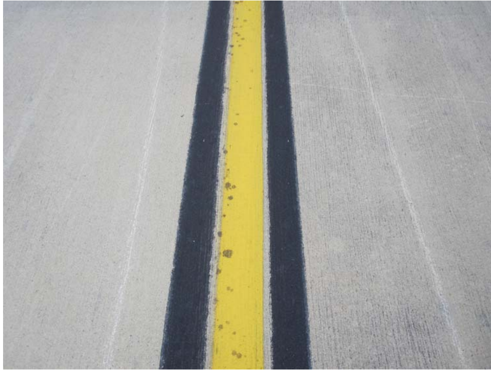
TASV-50. Satisfactory Paint.
