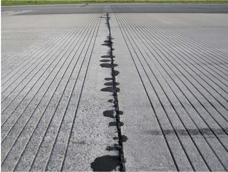
R1028SV-10C. Joint Seal Damage (Additional Sample Unit #26).
