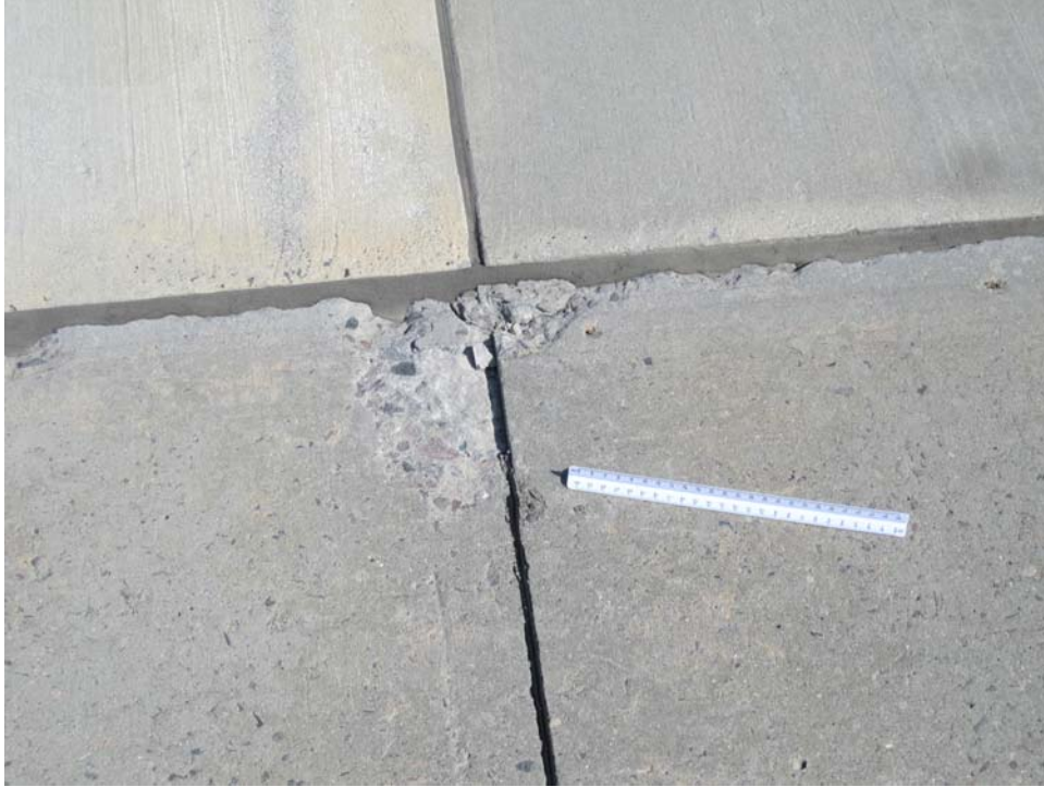
TA2SV-10. Corner Spalling (Sample Unit #04).
