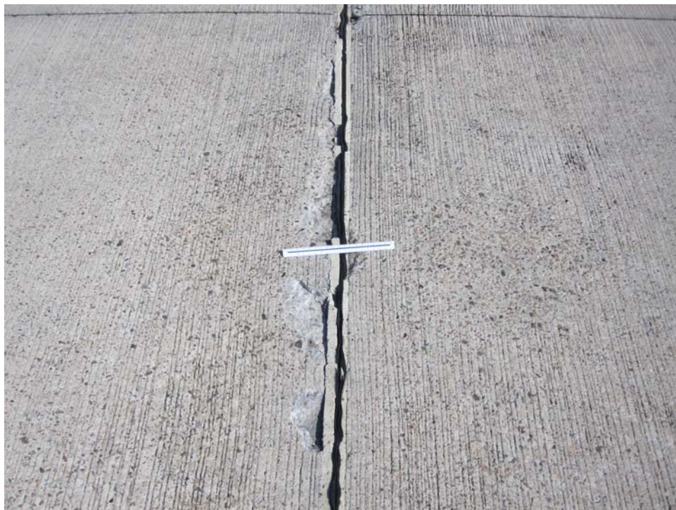
TESV-30. Joint Spalling (Sample Unit #26).
