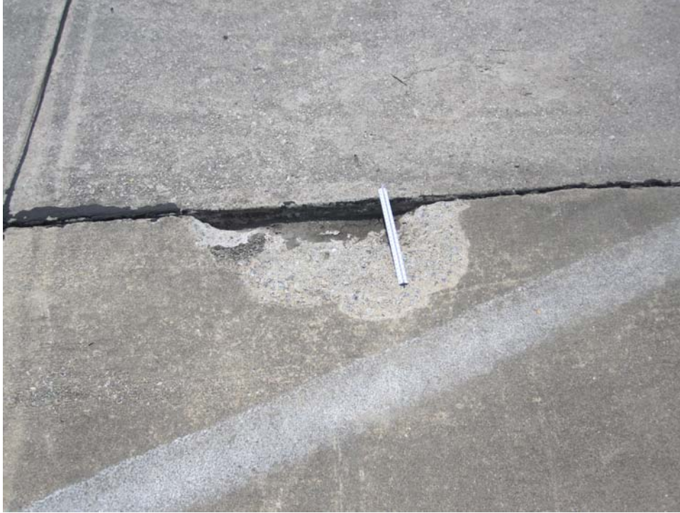
ASIGNORSV-20. Joint Spalling (Sample Unit #12).
