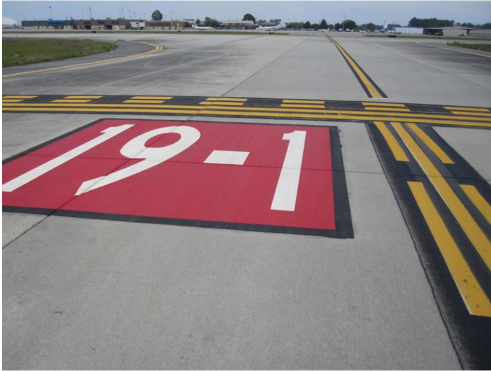
TA4SV-10. Satisfactory Paint.
