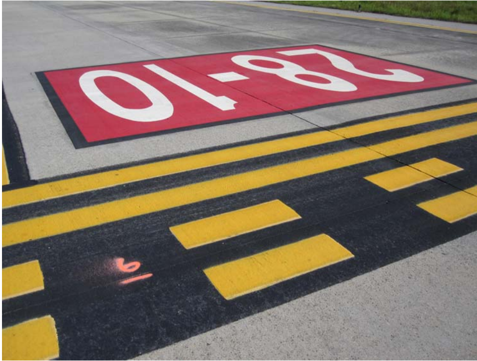
TASV-30. Satisfactory Paint.
