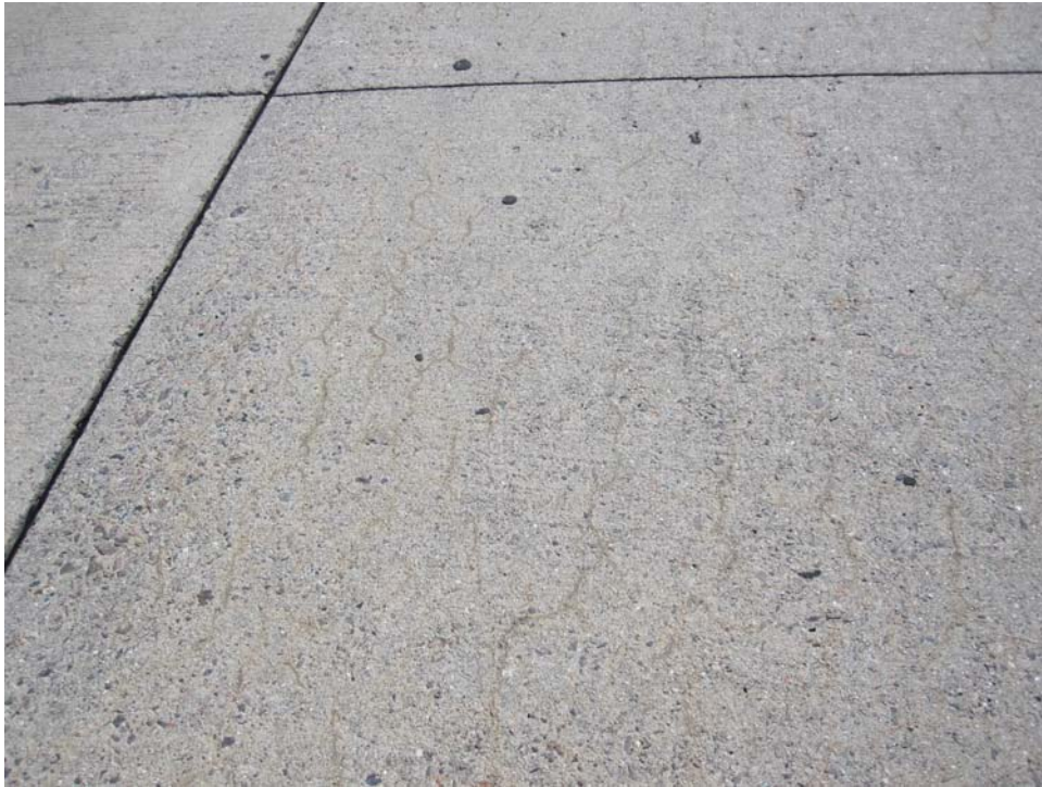
TCSV-40. ASR (Sample Unit #32).
