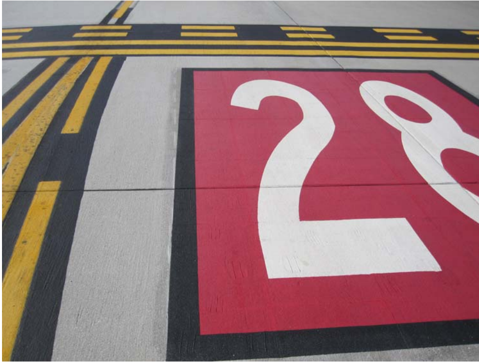
TESV-40. Satisfactory Paint.
