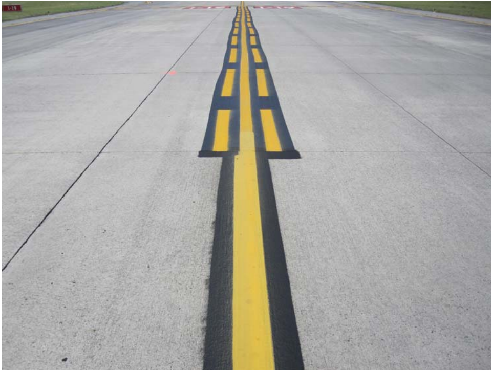
TCSV-30. Satisfactory Paint (2).
