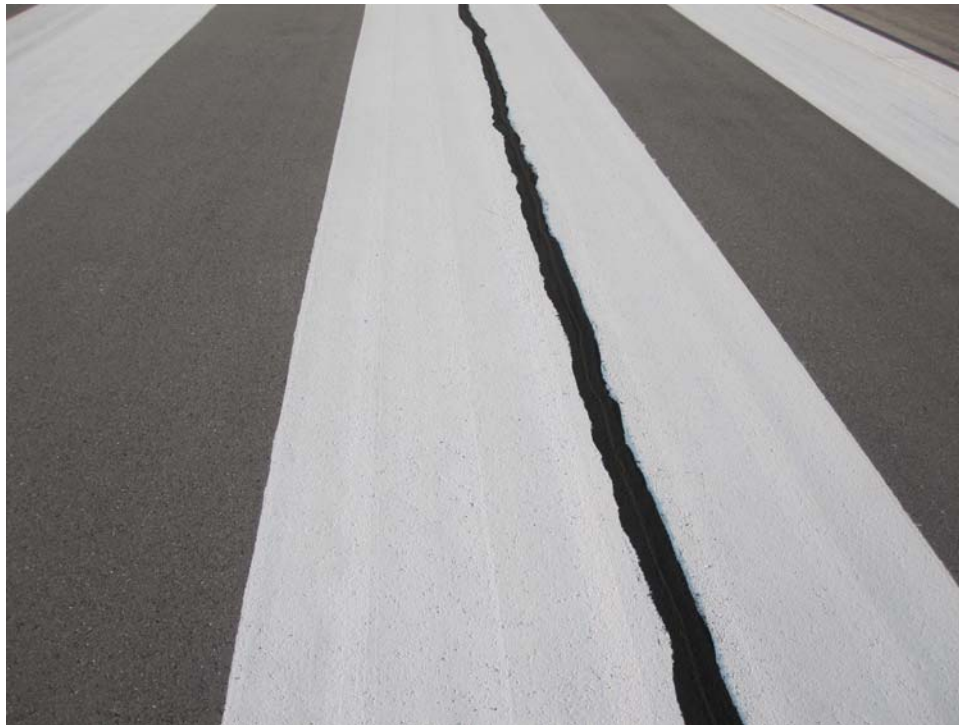
R119SV-10E. Satisfactory Paint.
