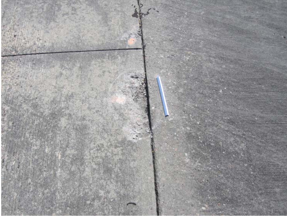
TESV-20. Joint Spalling (Sample Unit #38).
