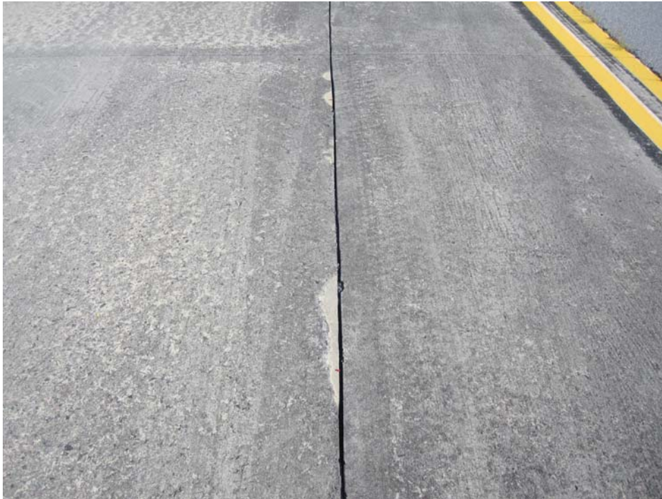
TASV-30. Small Patching (Sample Unit #08).
