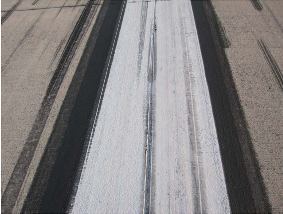
R119SV-10C. Satisfactory Paint.
