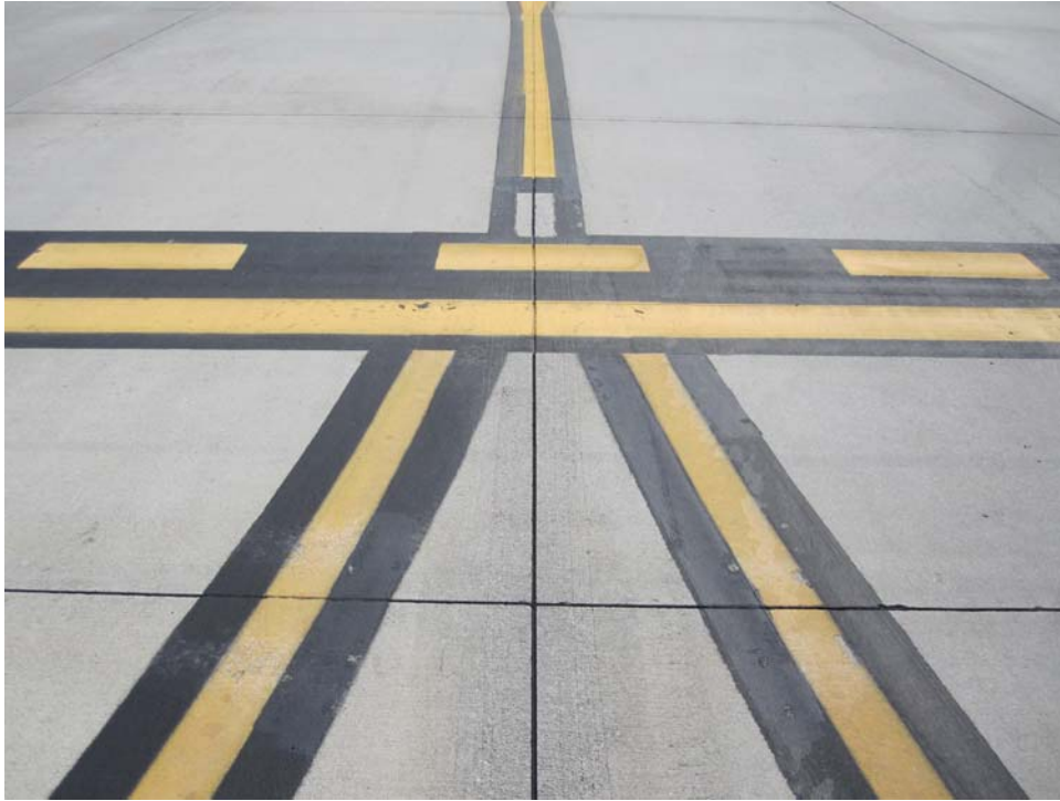
TA2SV-10. Satisfactory Paint.
