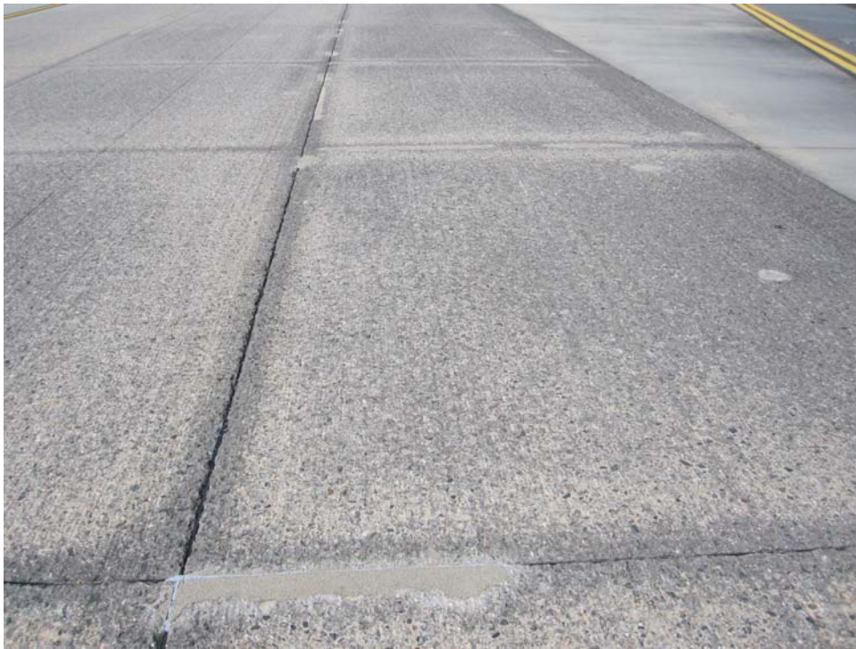
TESV-20. Small Patching (Sample Unit #18).
