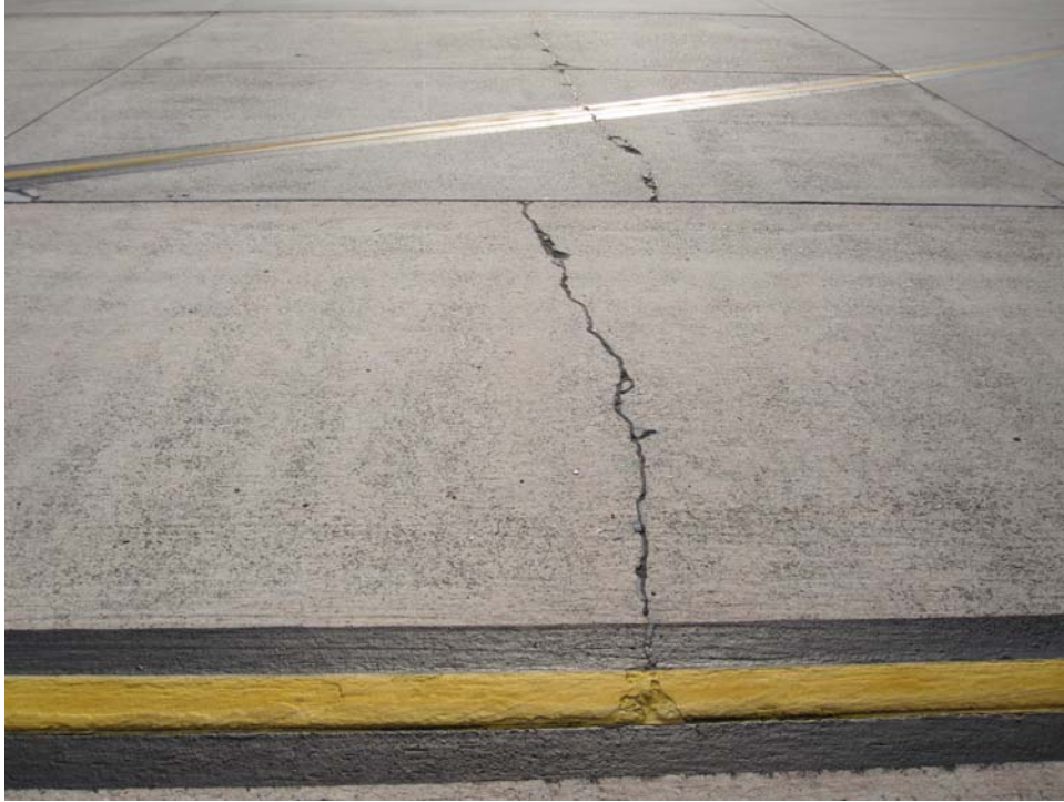
TE1SV-10. LTD Cracking (Sample Unit #10).
