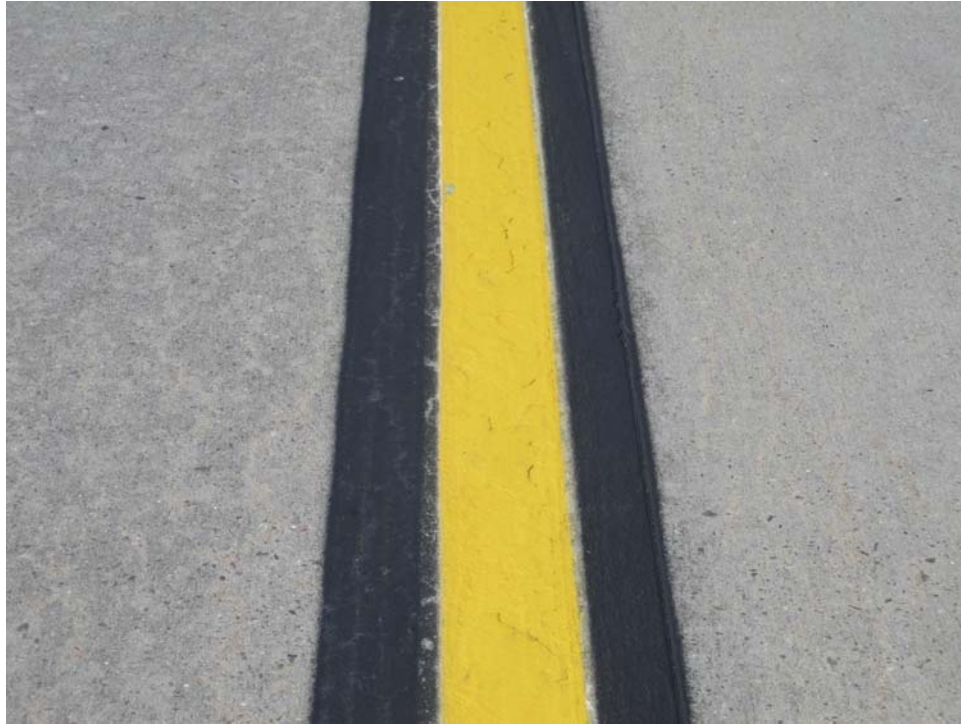
TESV-20. Satisfactory Paint.
