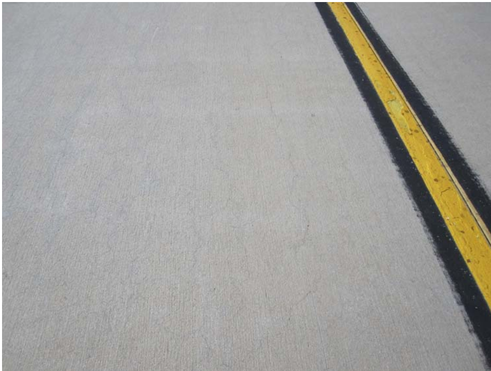
TESV-10. Shrinkage Cracking (Sample Unit #03).
