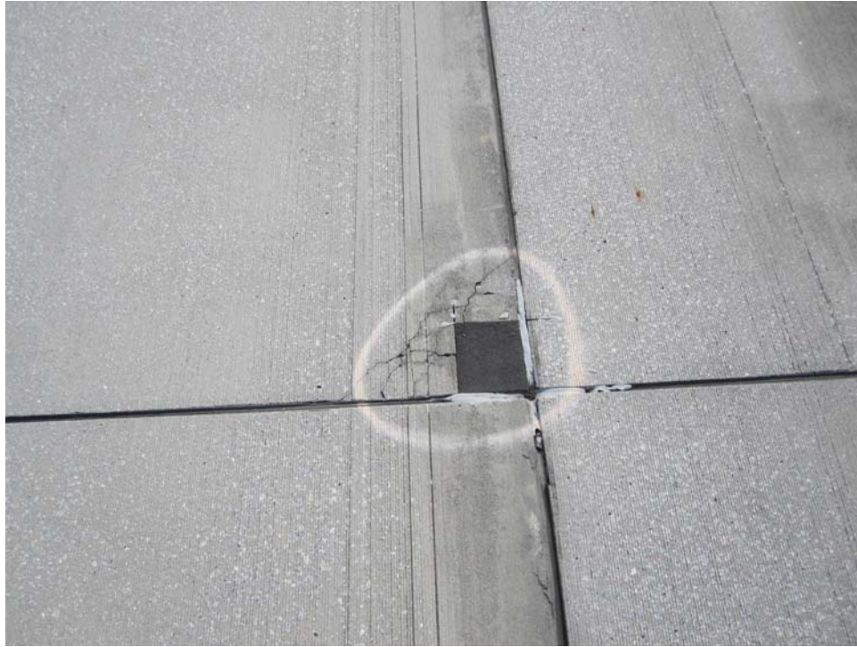
TESV-40. Corner Spalling (Sample Unit #19).
