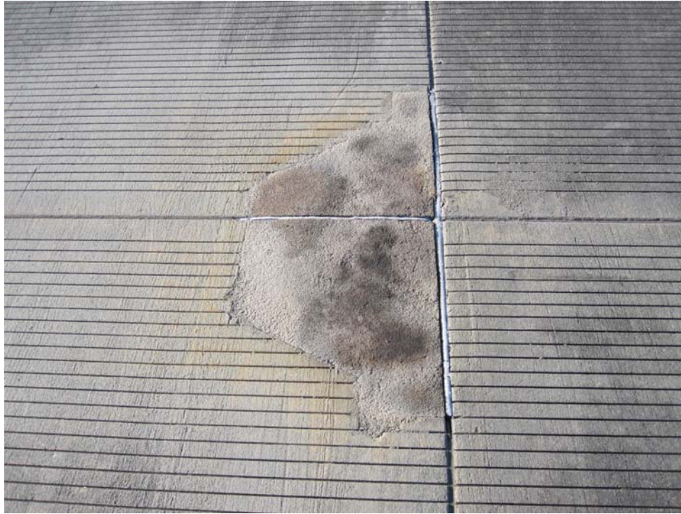
R119SV-20E. Small Patching (Sample Unit #04).
