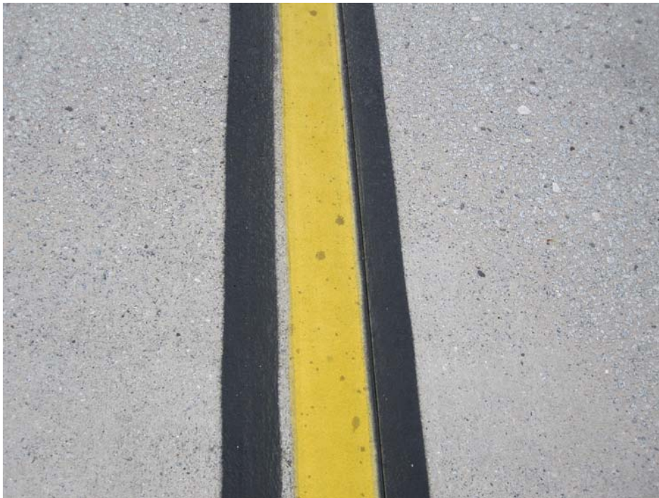
TASV-20. Satisfactory Paint.
