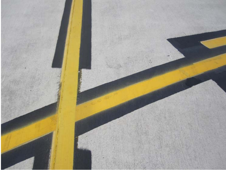
TCSV-10. Satisfactory Paint.
