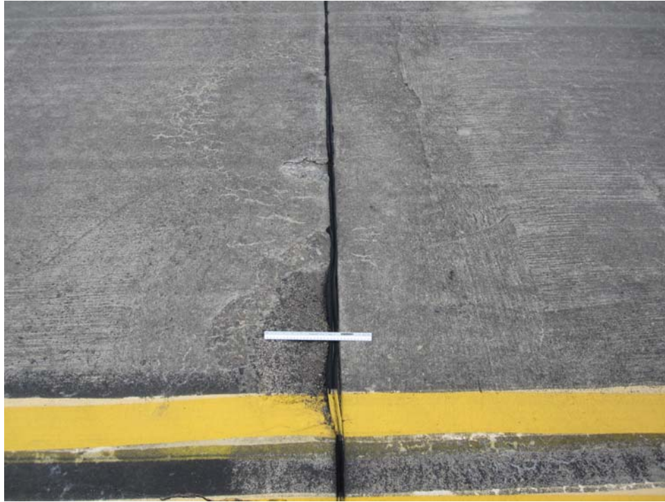
TCSV-30. Joint Spalling (Sample Unit #08).
