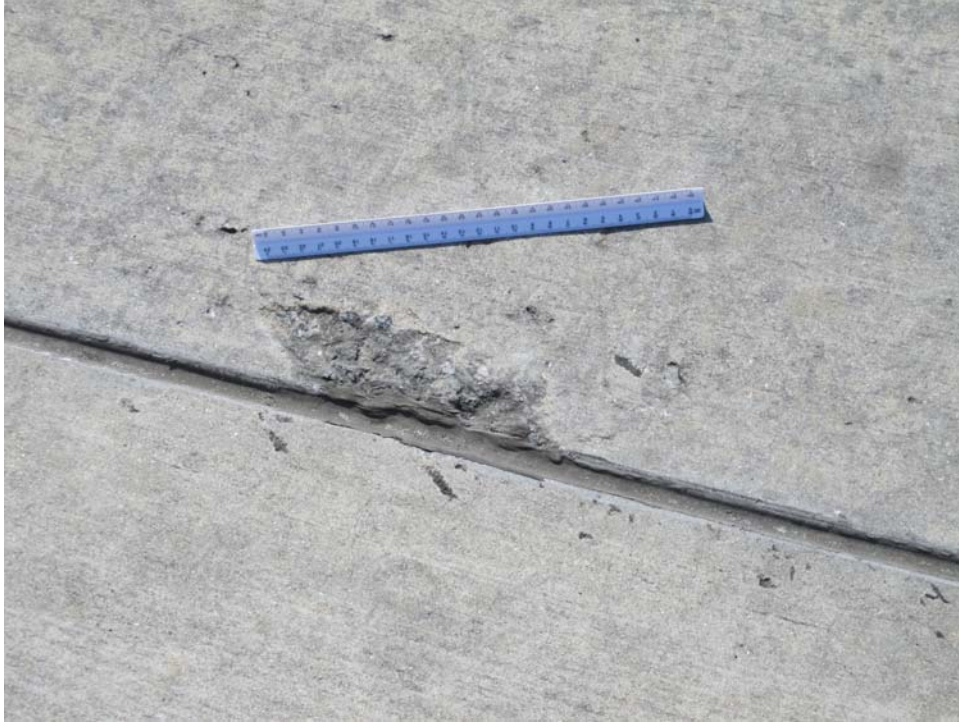
ATERMSV-20. Joint Spalling (Sample Unit #23).
