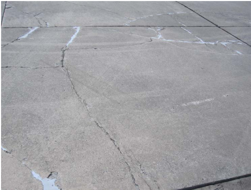
ASIGNORSV-20. Shattered Slab (Sample Unit #31).
