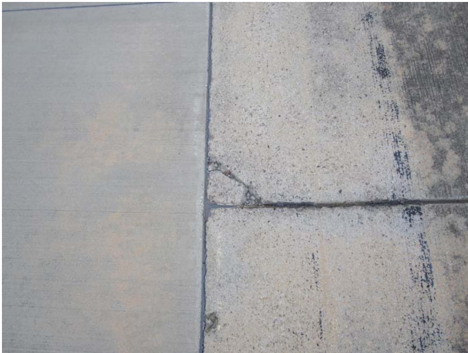
TASV-50. Corner Spalling (Sample Unit #29).
