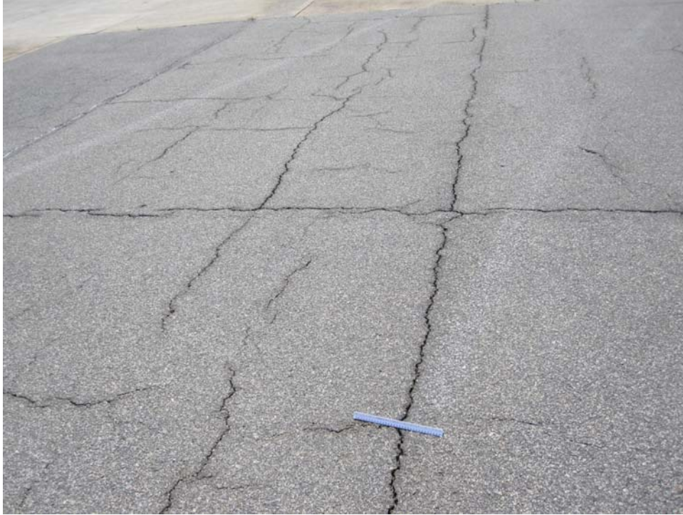
ASIGNORSV-10. Block Cracking (Sample Unit #15).
