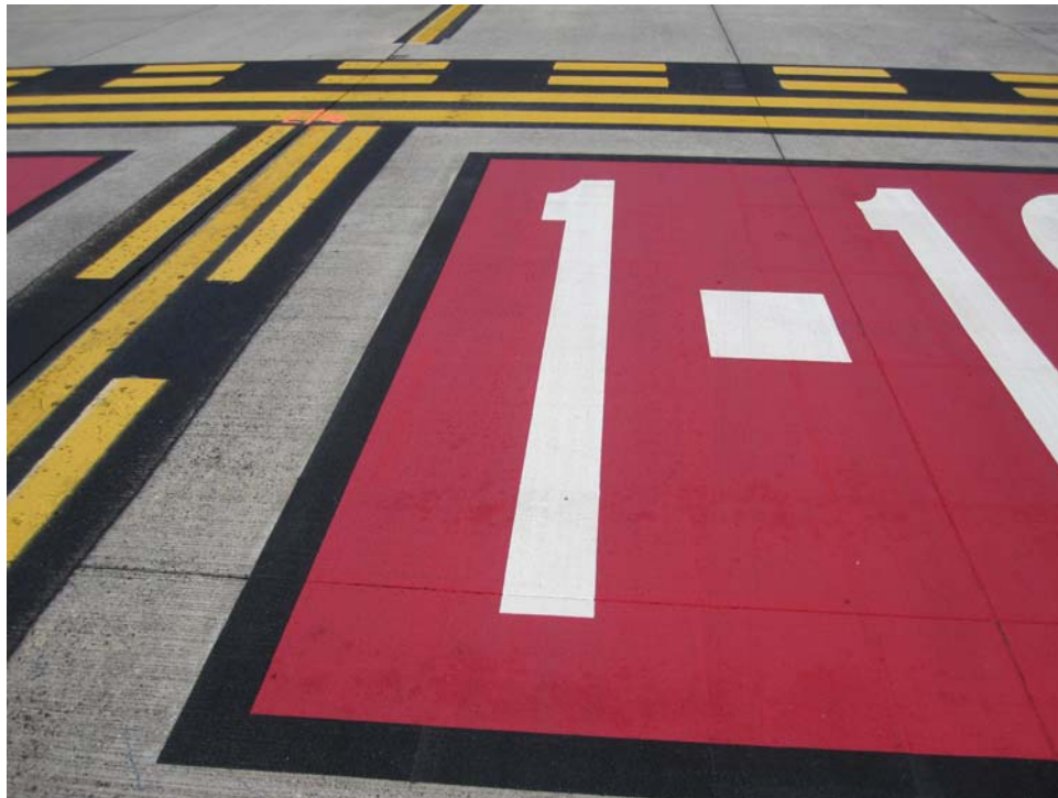
TB1SV-10. Satisfactory Paint.
