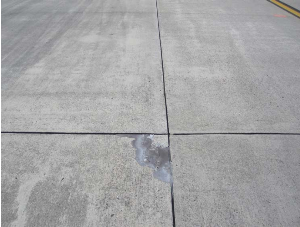
TCSV-20. Corner Spalling (Sample Unit #40).
