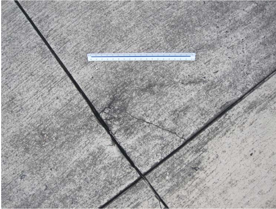
TC1SV-10. Corner Spalling (Sample Unit #20).
