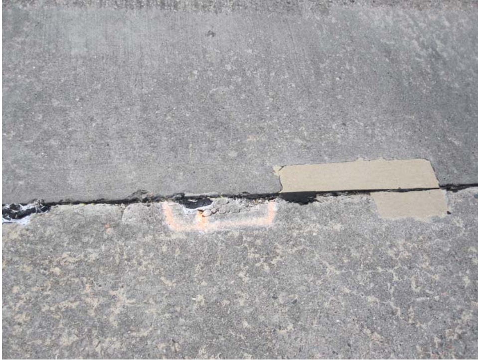
TE1SV-10. Joint Spalling (Sample Unit #01).
