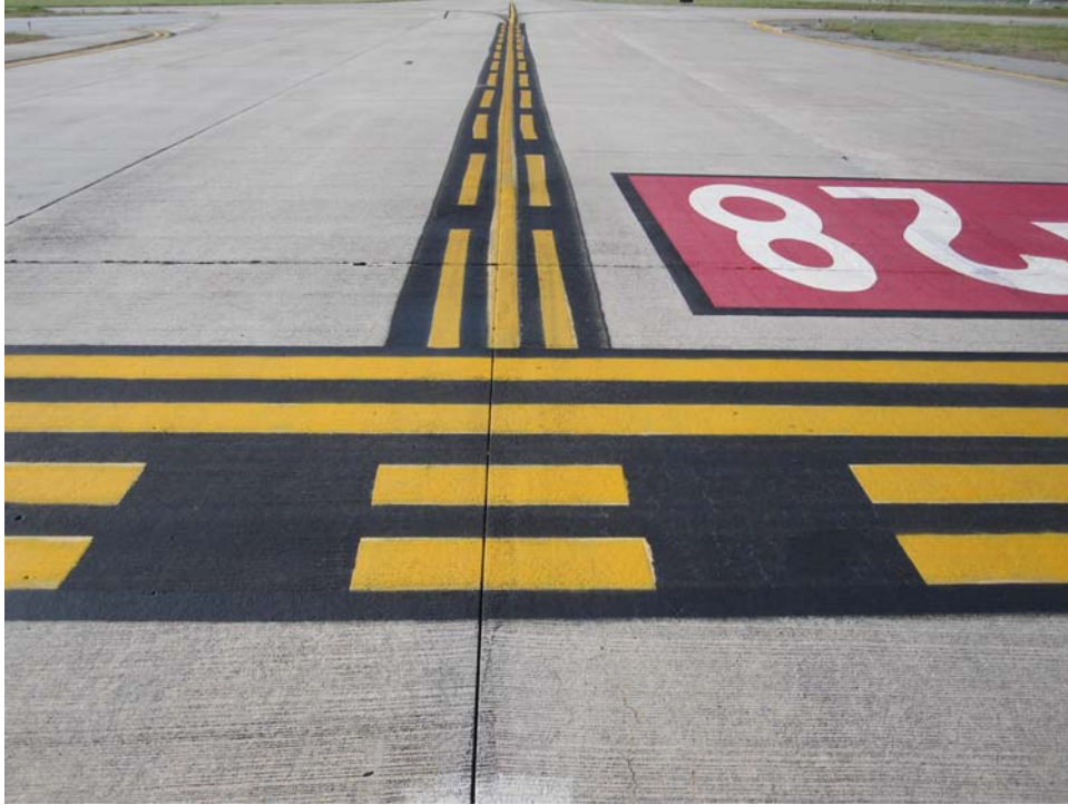
TBSV-20. Satisfactory Paint (2).
