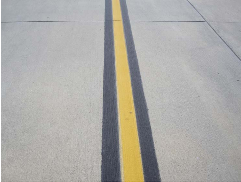
TCSV-50. Satisfactory Paint.
