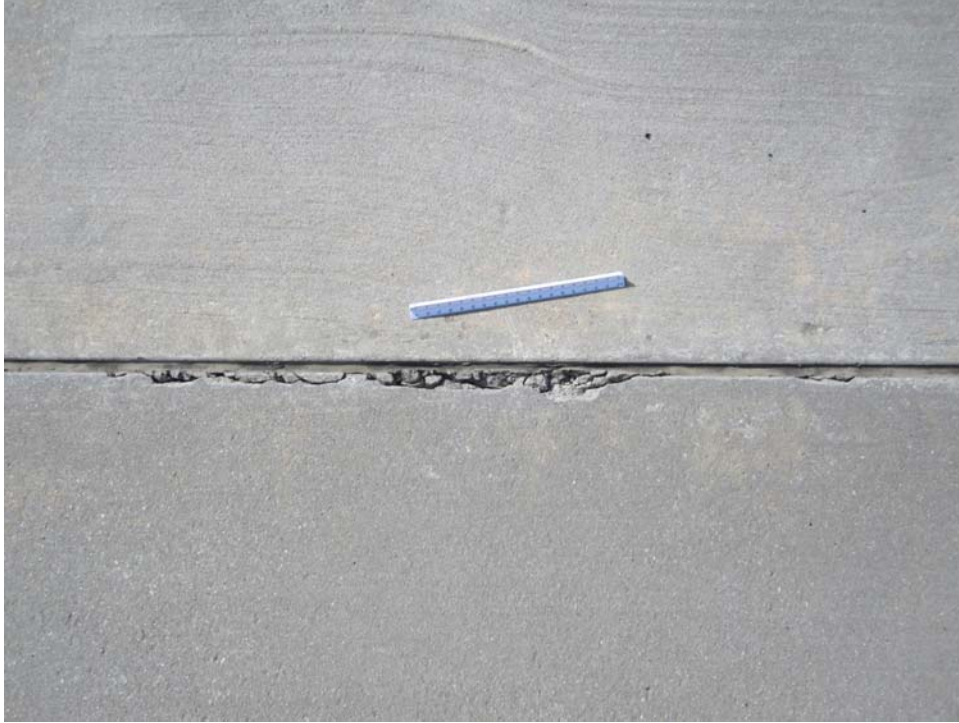
TA1SV-10. Joint Spalling (Sample Unit #04).
