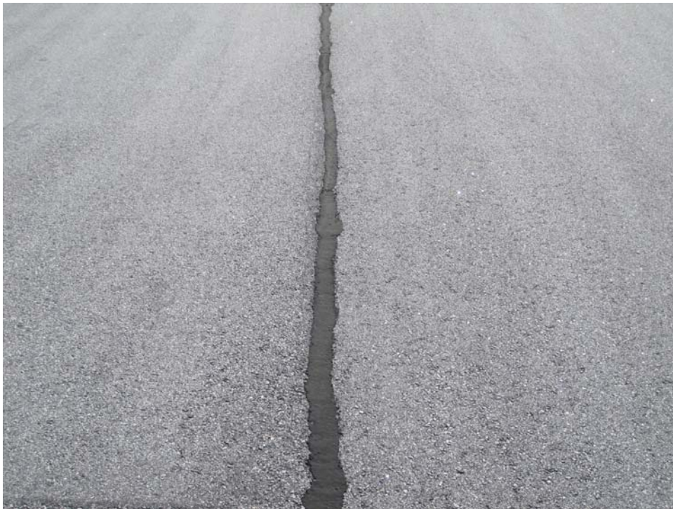
TBSV-10. Longitudinal and Transverse Cracking (Sample Unit #15).
