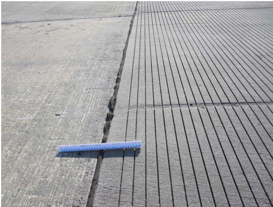
R119SV-20E. Joint Seal Damage (Sample Unit #01).
