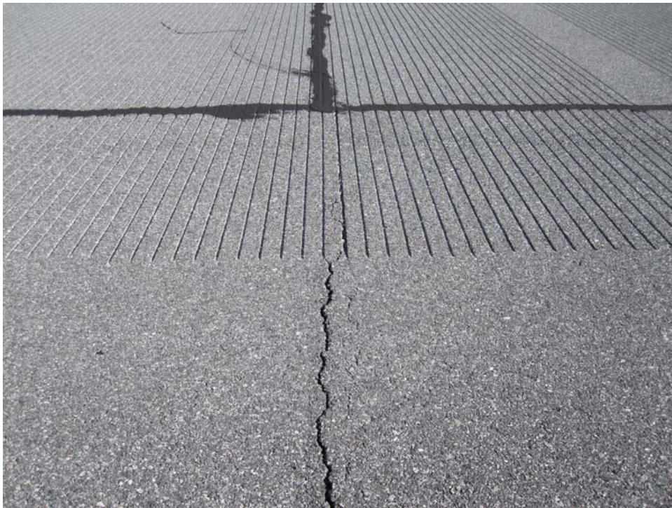
R1028SV-10S. Longitudinal and Transverse Cracking (Sample Unit #44).
