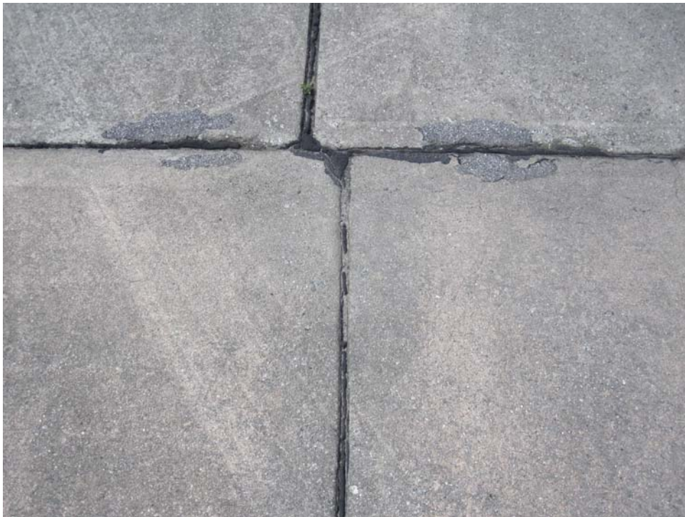
ASIGNORSV-20. Joint Seal Damage (Sample Unit #15).
