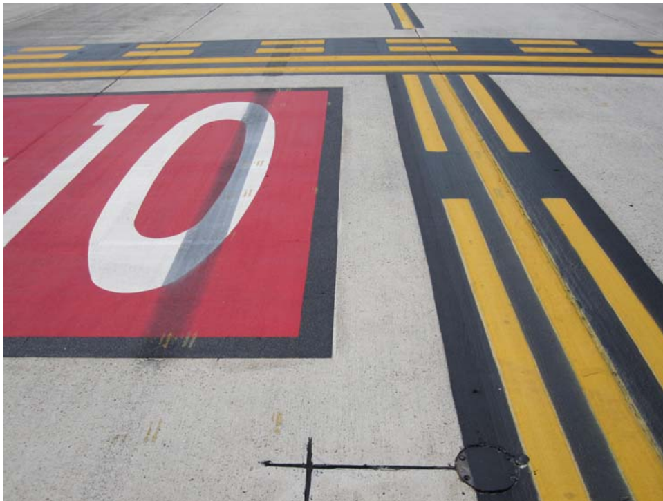
TE1SV-10. Satisfactory Paint (1).
