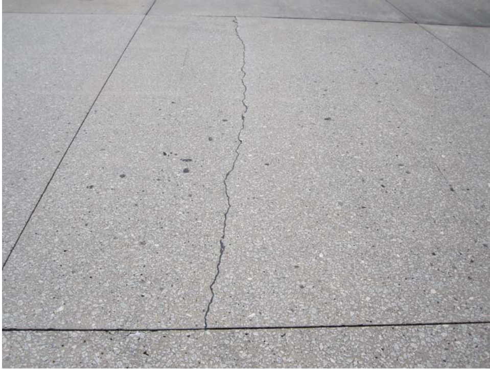
TASV-20. LTD Cracking (Sample Unit #26).
