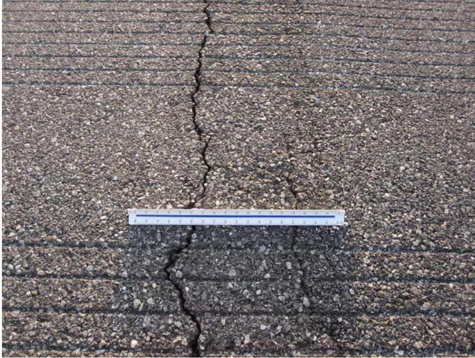
R1028SV-10S. Raveling (Sample Unit #23).
