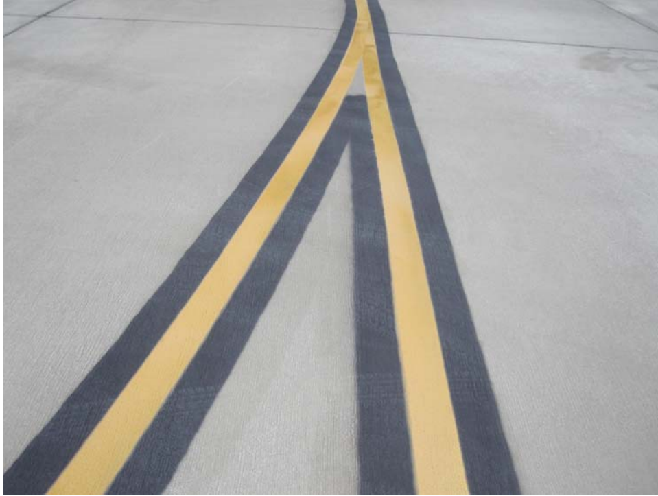
TASV-05. Satisfactory Paint.
