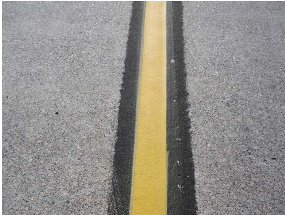
TCSV-30. Satisfactory Paint (1).
