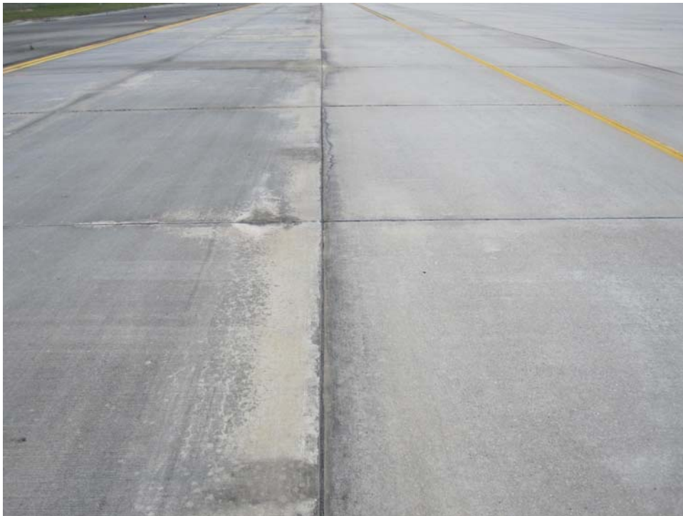
ATERMSV-10. Pumping (Sample Unit #01).
