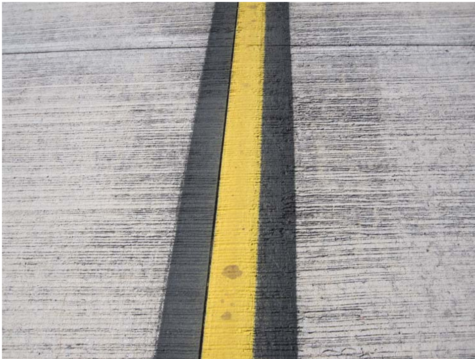
TBSV-20. Satisfactory Paint (1).
