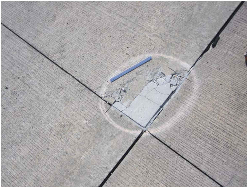
TBSV-20. Corner Spalling (Sample Unit #101).
