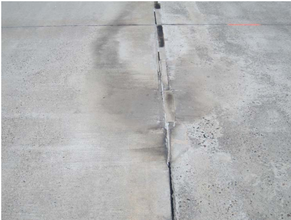
TA3SV-10. Pumping (Sample Unit #02).
