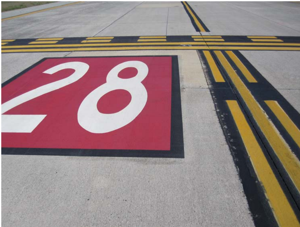
TCSV-60. Satisfactory Paint.
