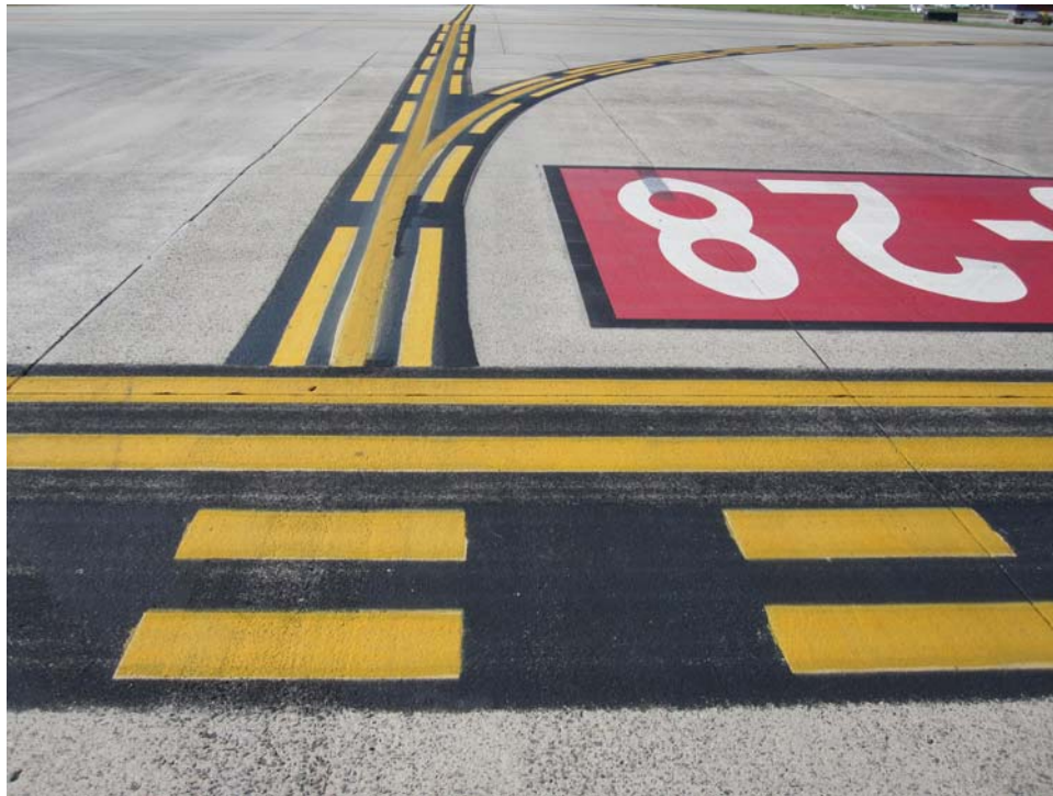
TASV-40. Satisfactory Paint.
