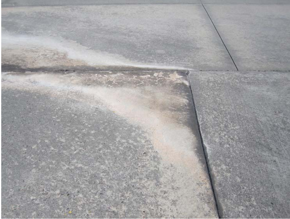
TASV-30. Pumping (Additional Sample Unit #01).
