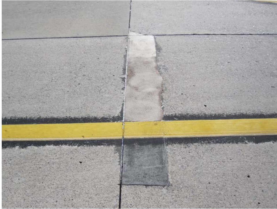
TASV-40. Large Patching (Sample Unit #09).
