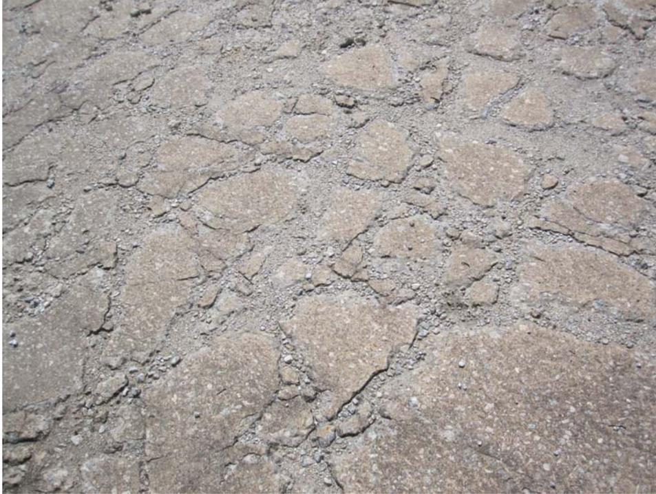
A01LW-40. Shattered Slab (Sample Unit #04).
