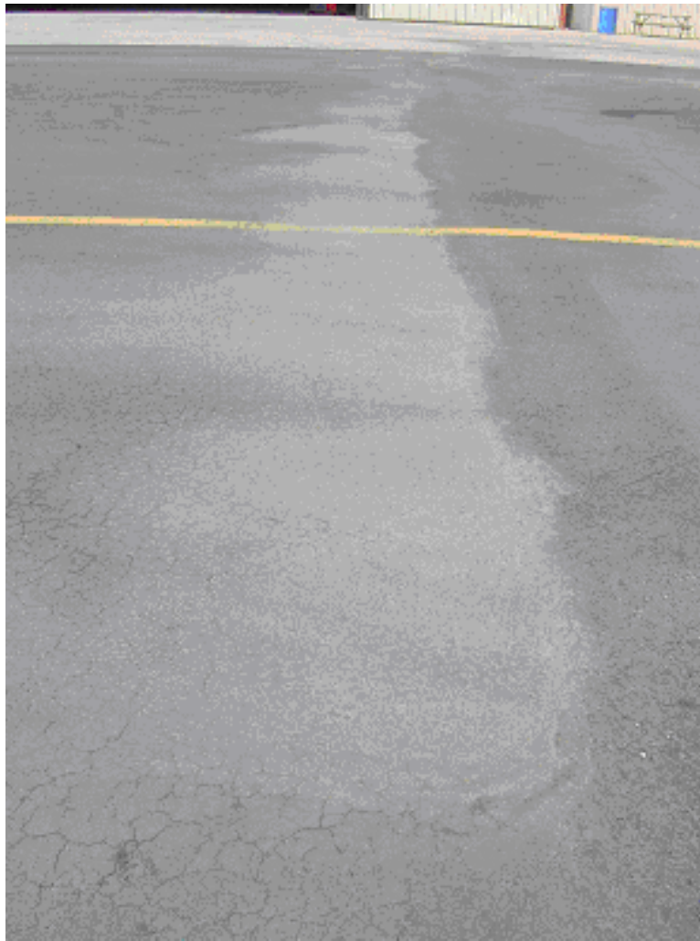
Depression in section A01WI-20.
