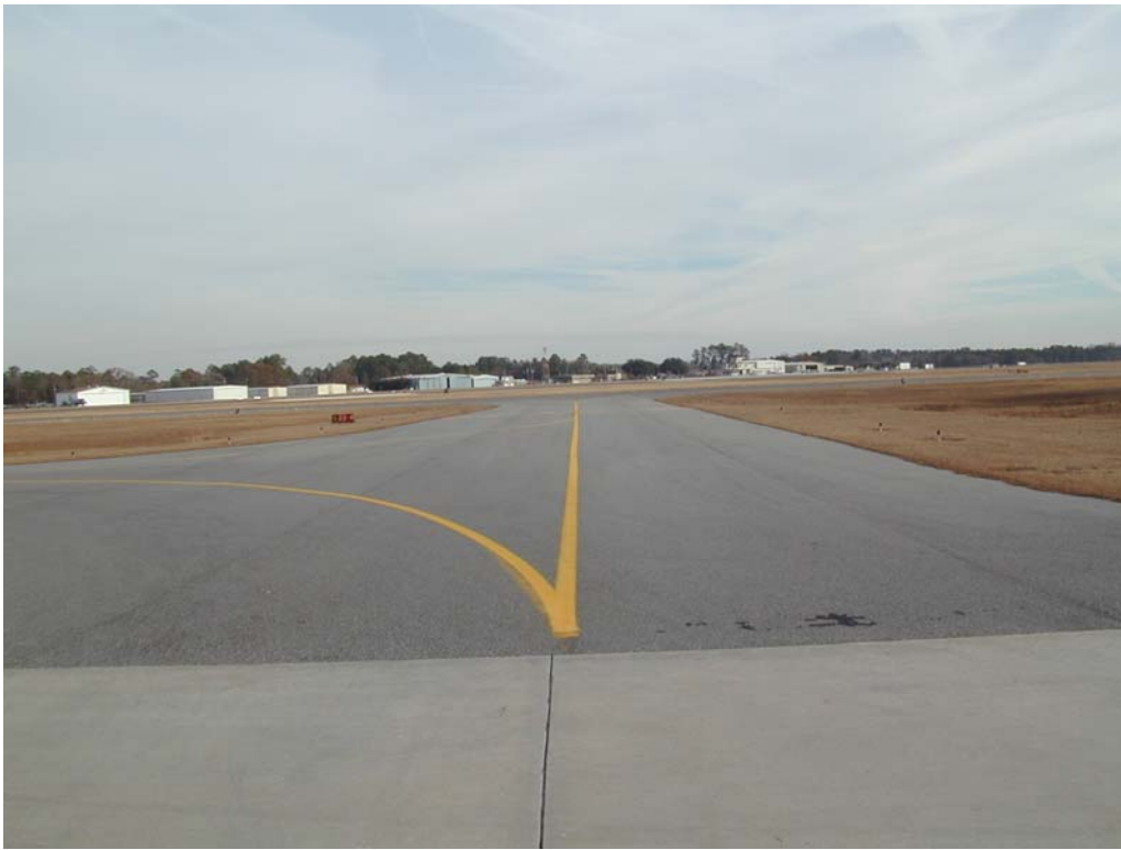
Overview of section TNVL-10.
