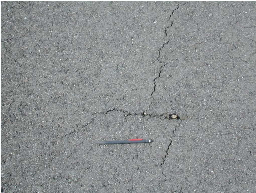
L&T cracking in section R1331VL-10.
