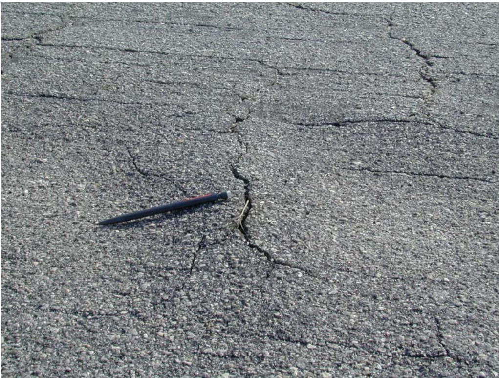
L&T cracking with swelling in section TFVL-10.
