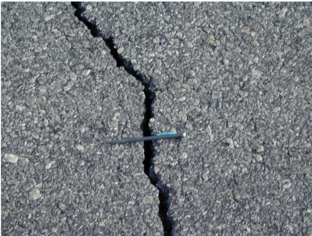
L&T cracking in section TAVL-10.
