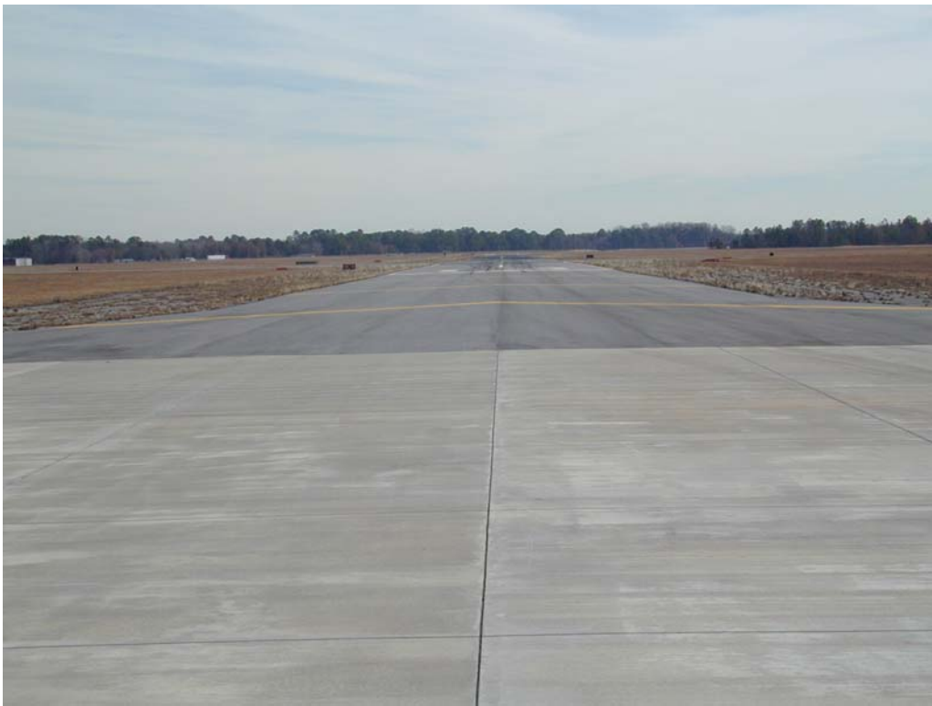
Overview of section R1331VL-10.
