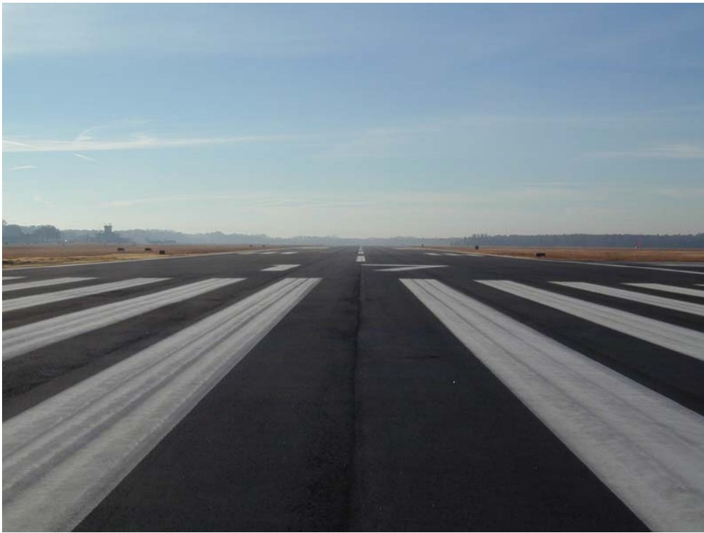
Overview of section R1735VL-10.
