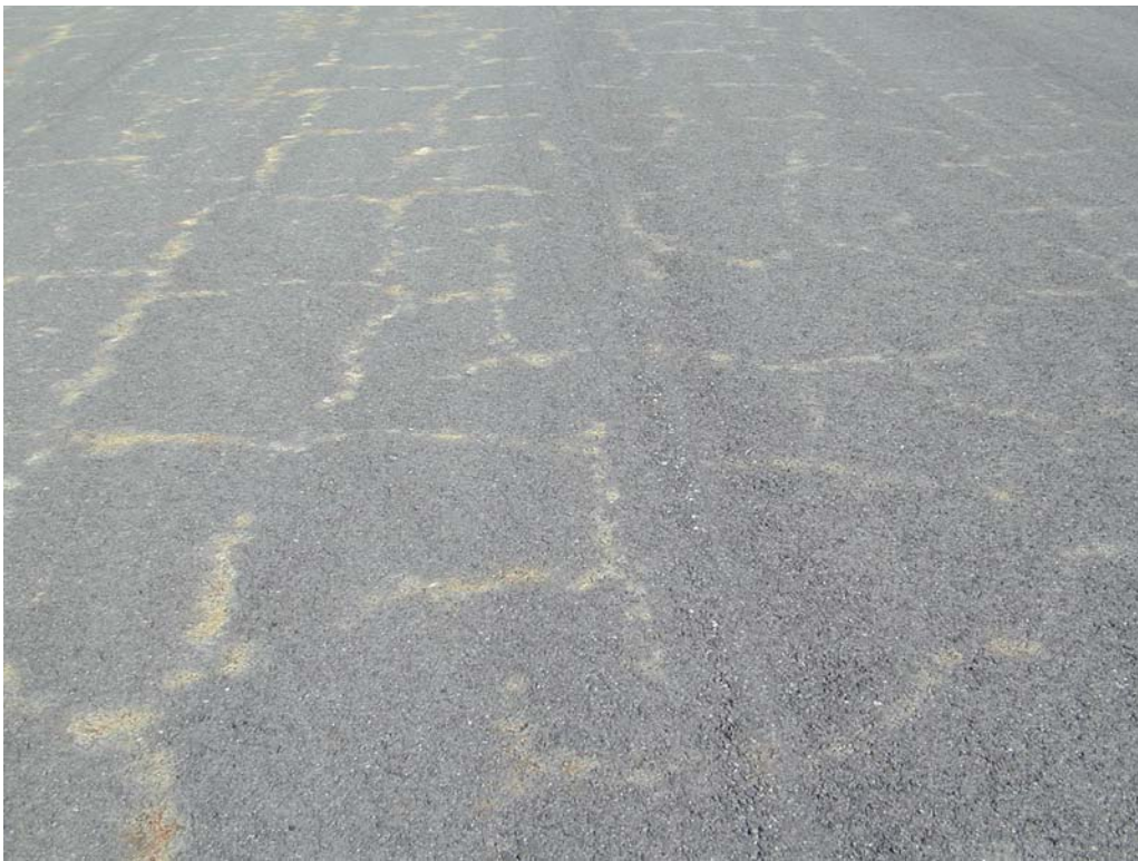
L&T cracking beginning to form blocks in section R422VL-10.
