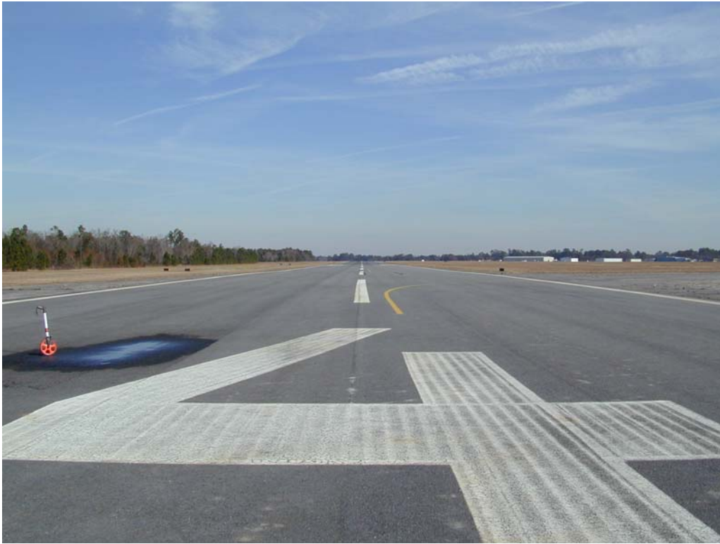
Overview of section R422VL-10.
