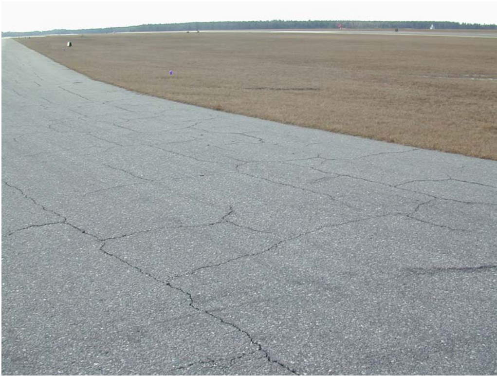
Block cracking in section TAVL-10.
