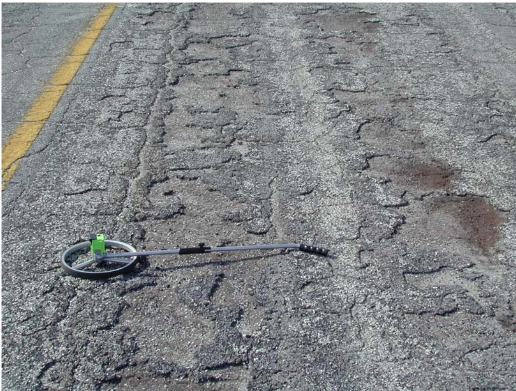
Raveling and weathering in section TCVL-10.
