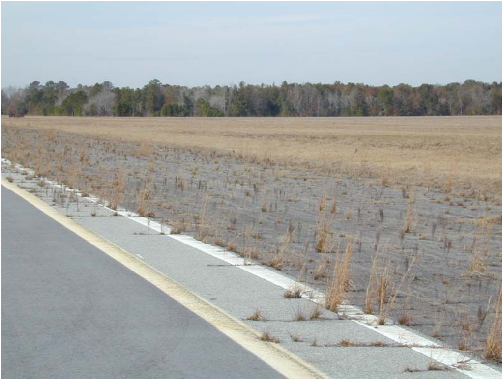
Overview of underlying pavement in section R1331VL-10.
