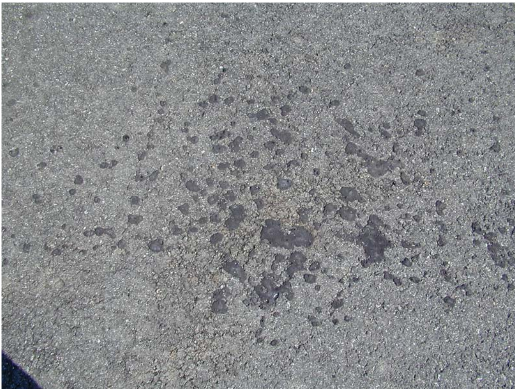
Bleeding in section R422VL-10.
