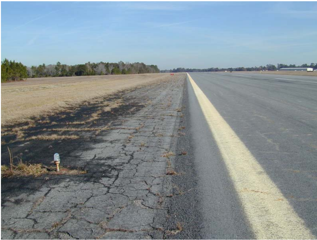
Overview of underlying pavement in section R422VL-10.
