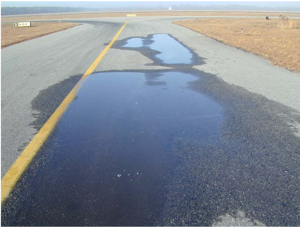
Depression with alligator cracking in sample unit 12 of section A01VL-40.
