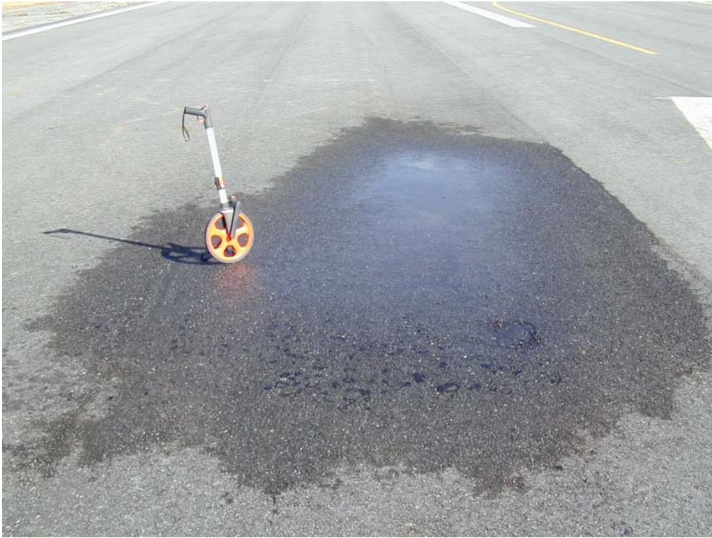
Depression and weathering in section R422VL-10.
