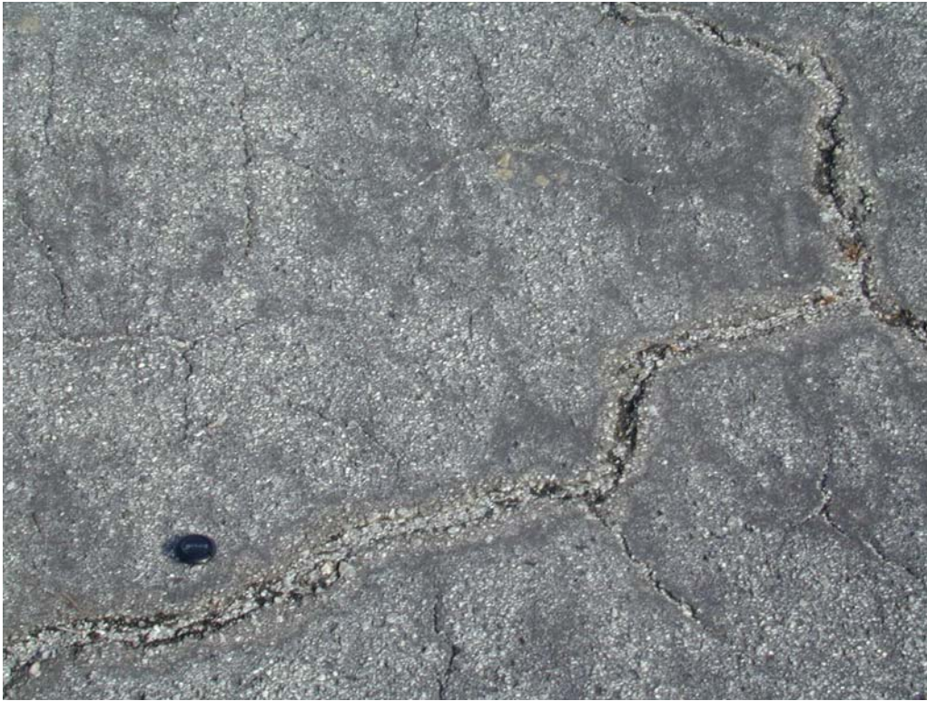
Block cracking in section TCVL-10.
