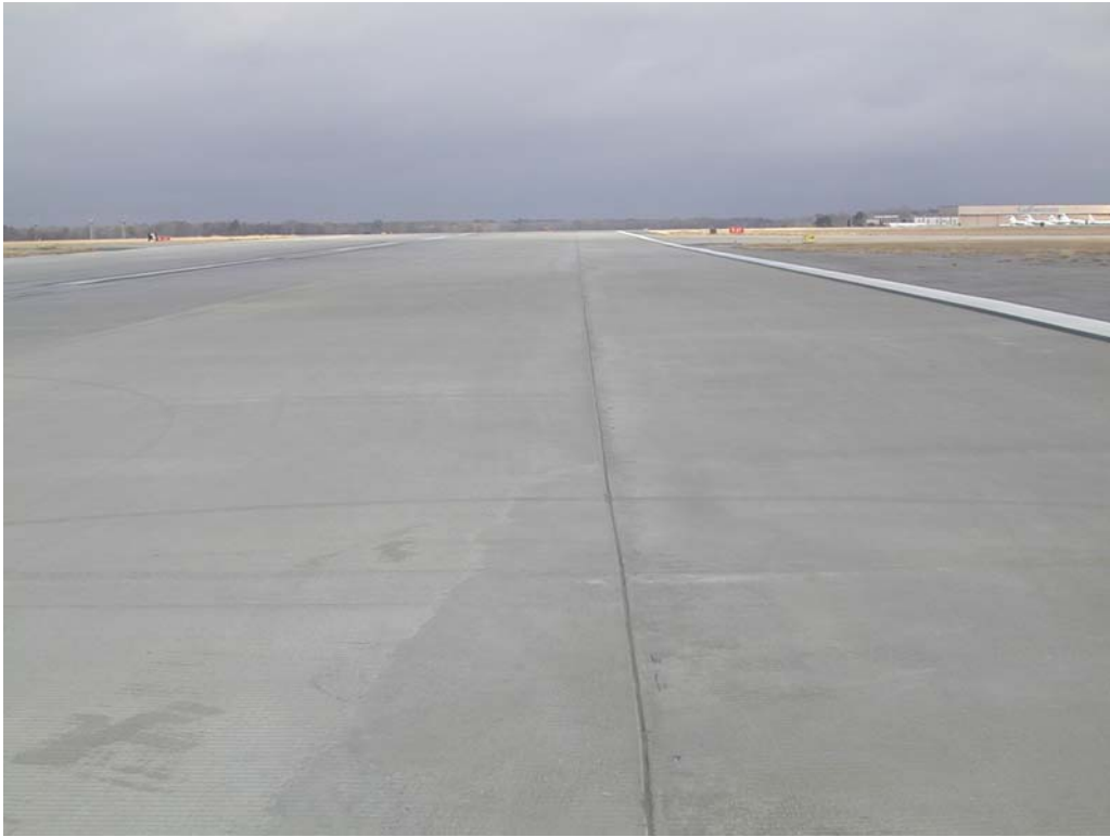
Overview of section R1836SV-20E.
