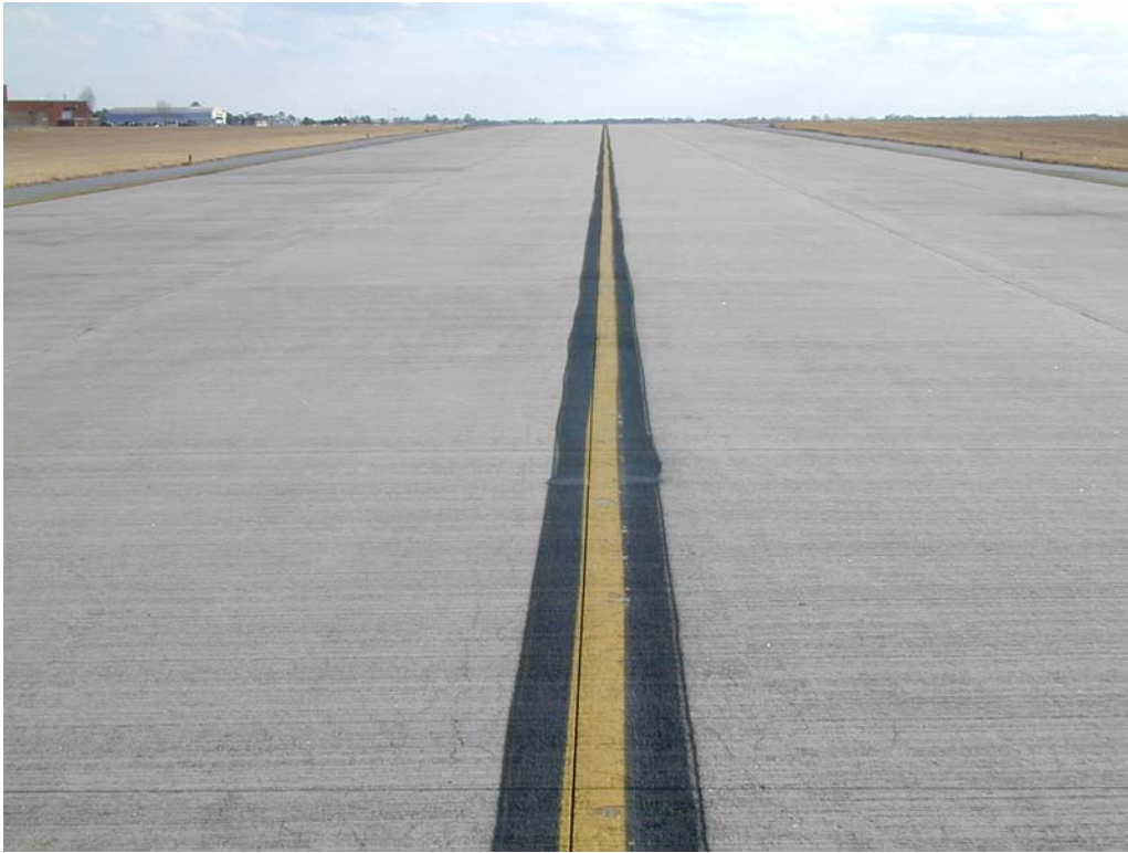
Overview of section TBSV-20.
