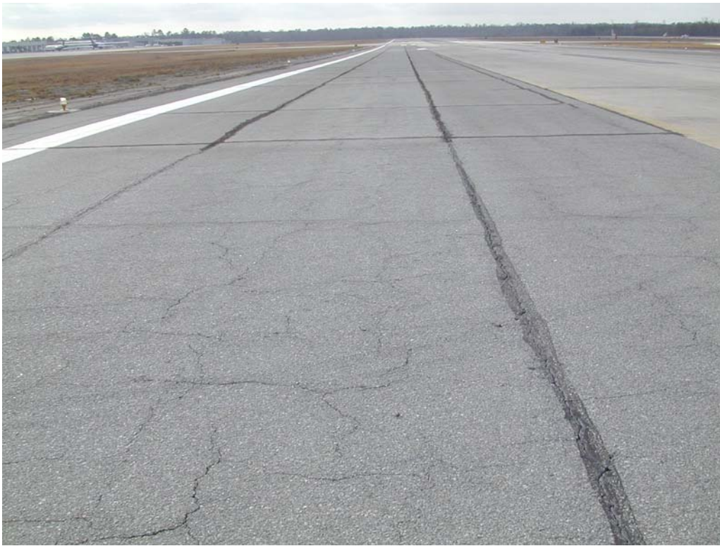
Overview of section R1836SV-10E.
