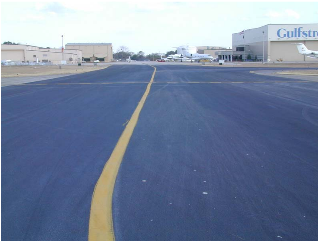
Overview of section TBSV-10.
