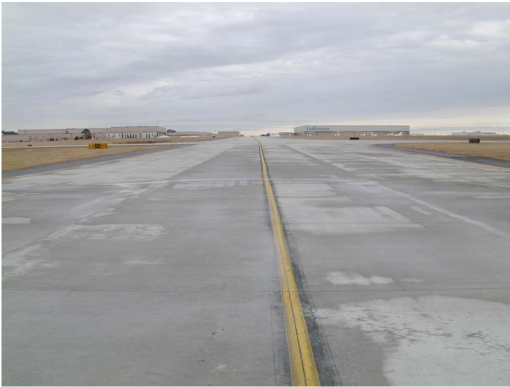
Overview of section TA2SV-10.
