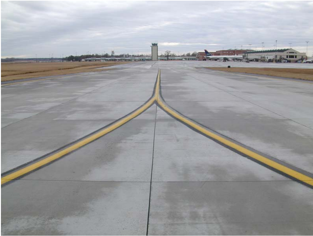
Overview of section TA3SV-10.
