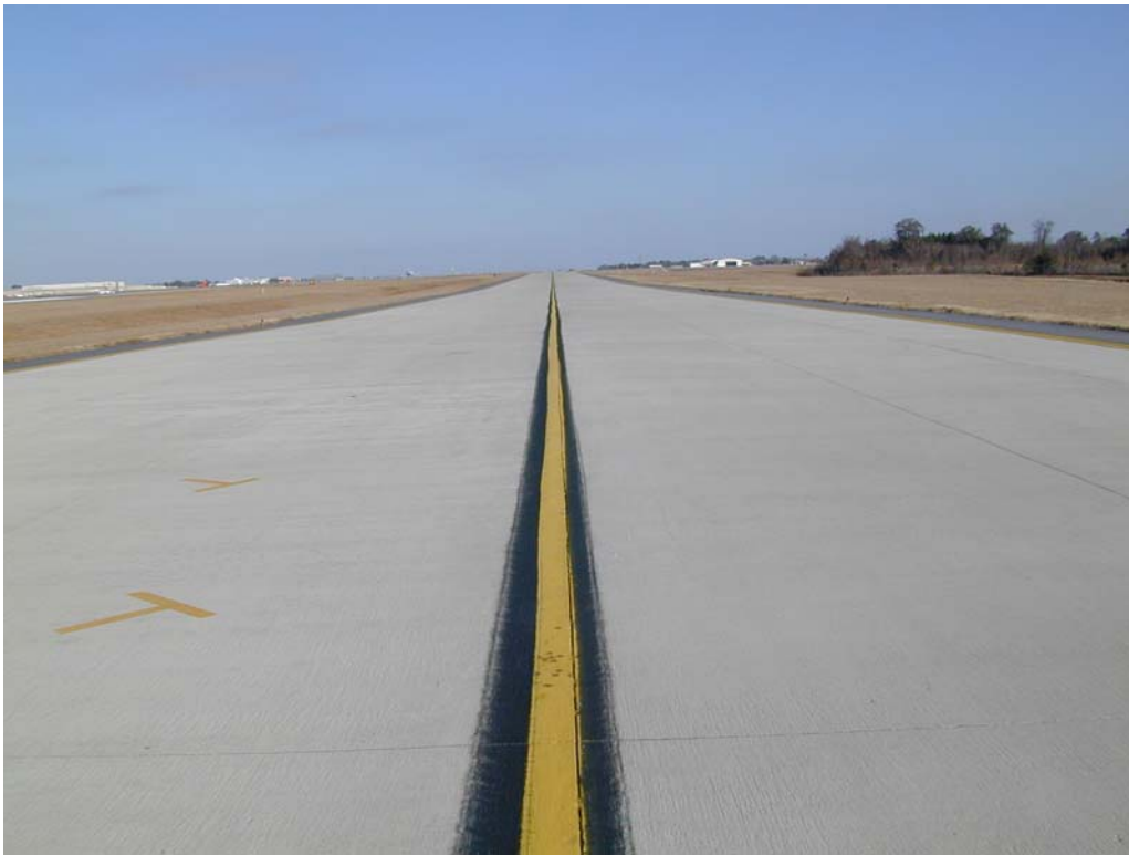
Overview of section TCSV-10.
