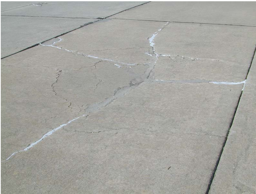
Shattered slab in section ASIGNORTHSV-20.
