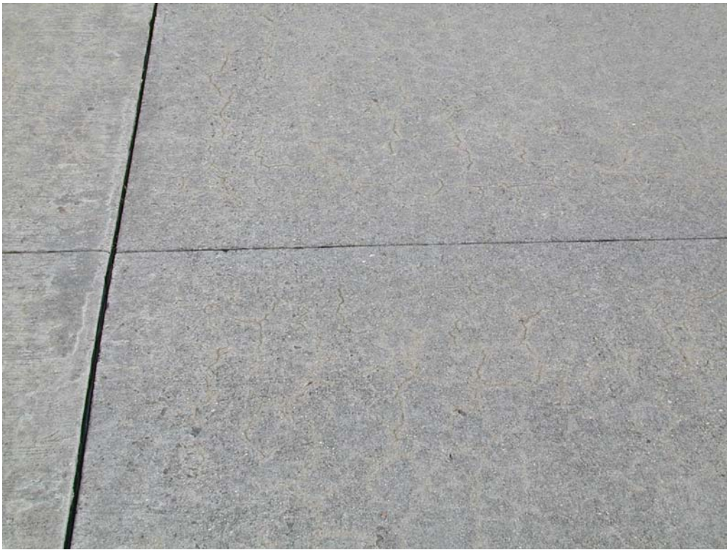
Shrinkage cracking in section TCSV-40.
