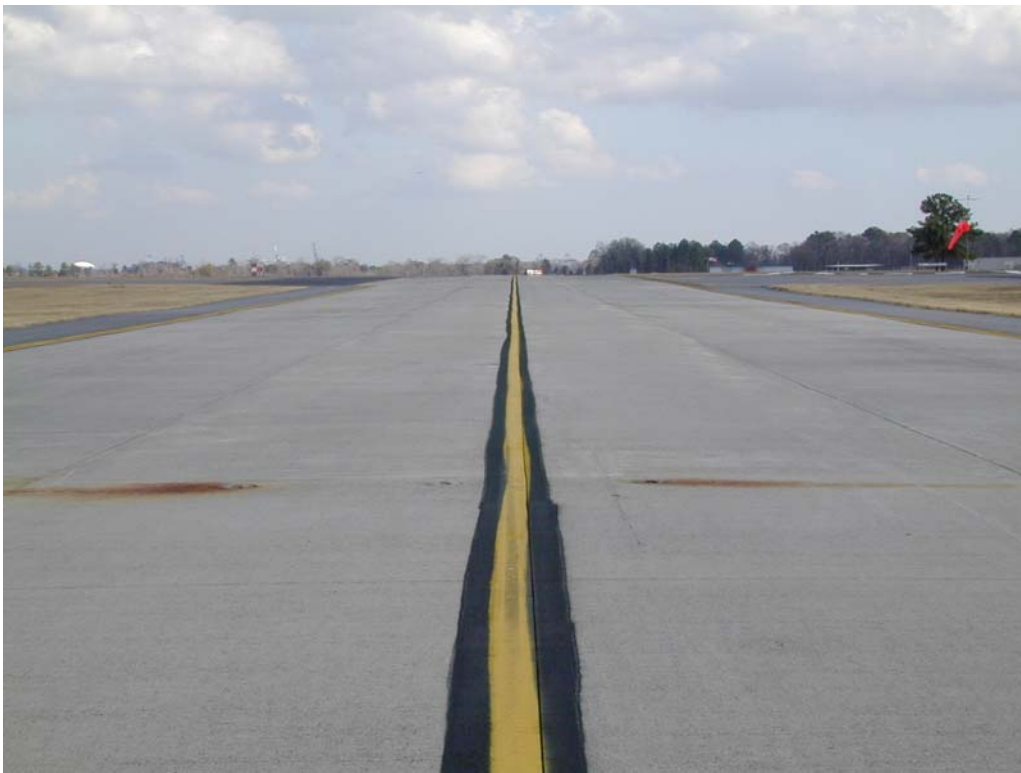
Overview of section TCSV-40.
