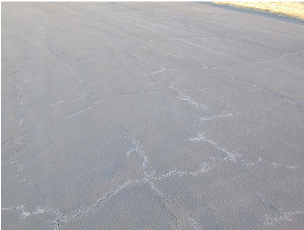
Block cracking in section TB2SV-10.
