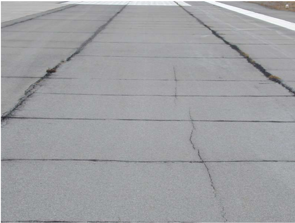
Overview of section R1836SV-10W.
