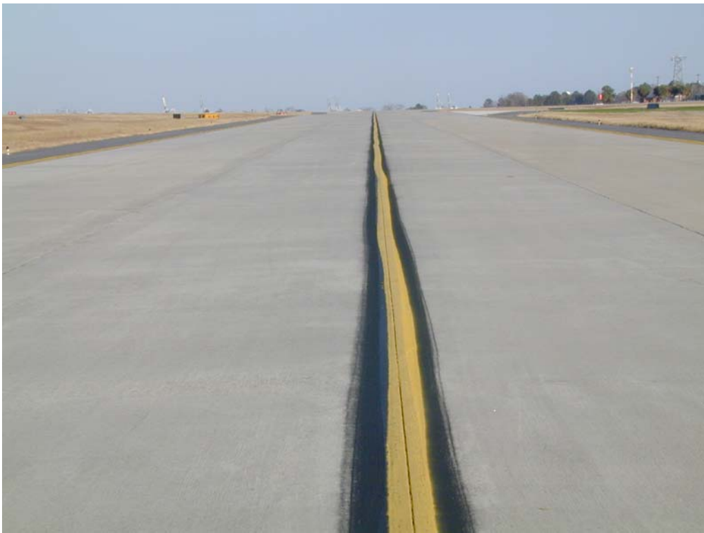
Overview of section TCSV-20.
