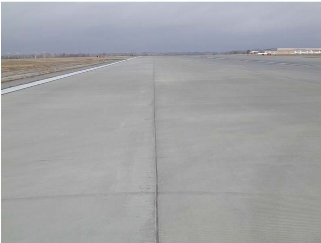
Overview of section R1836SV-20W.
