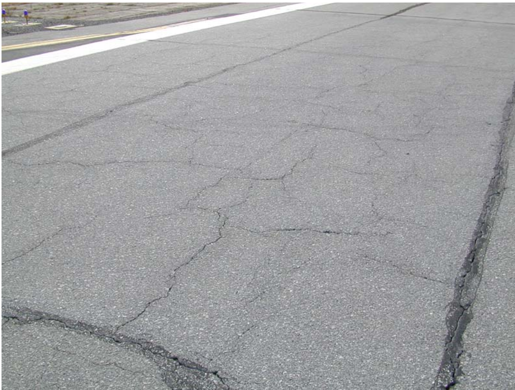
Block cracking in section R1836SV-10E.
