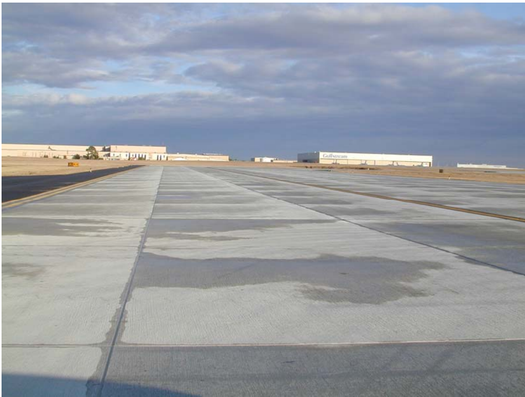
Overview of section TA1SV-10.
