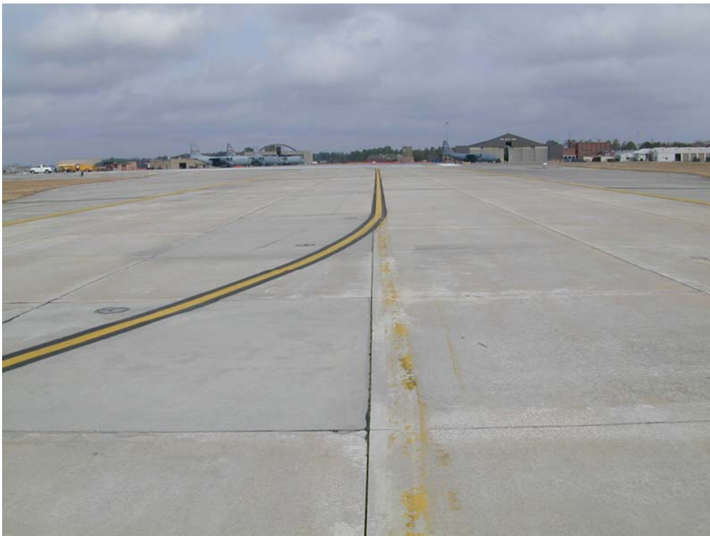
Overview of section TCSV-60.
