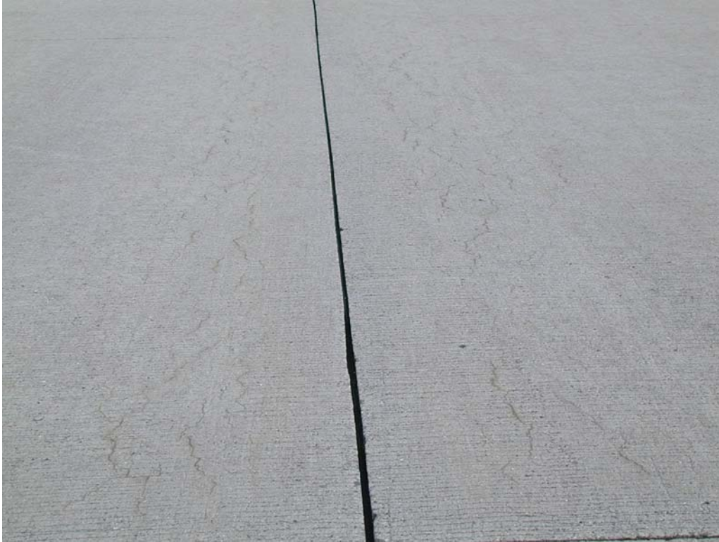
Shrinkage cracking in section TESV-20.
