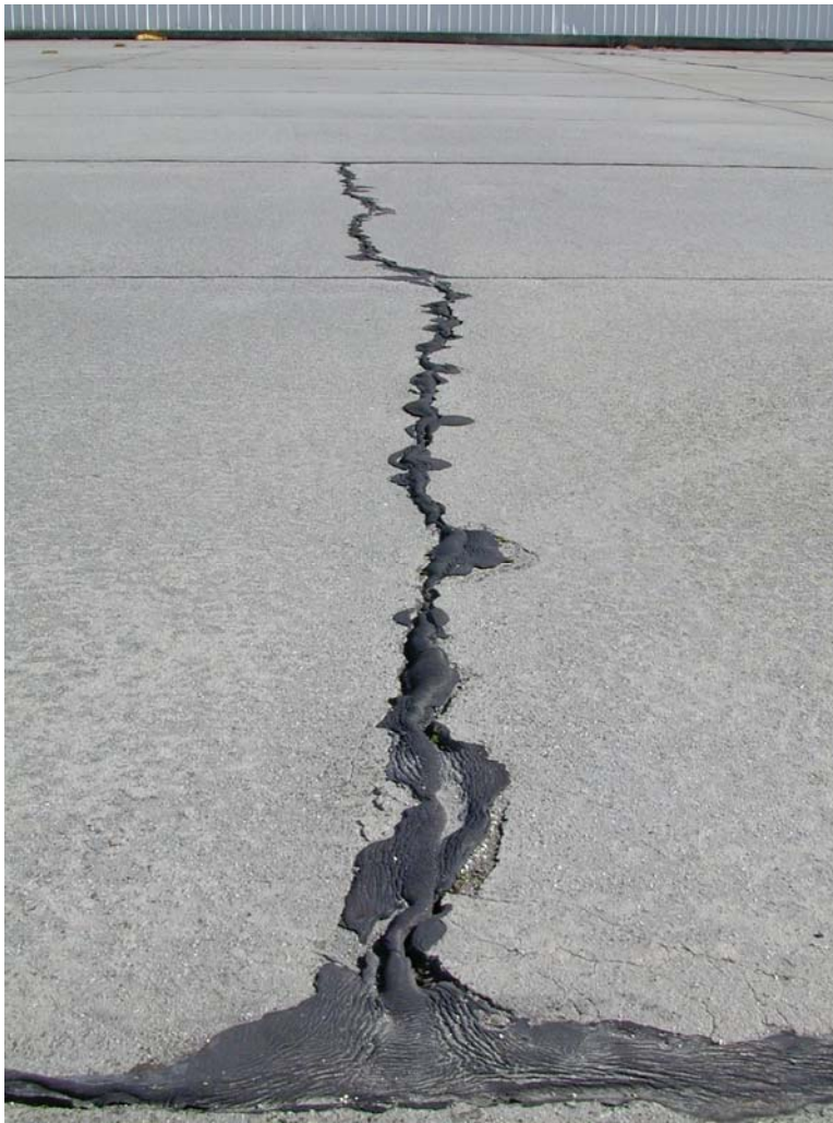
LTD cracking in section ASIGSOUTHSV-10.
