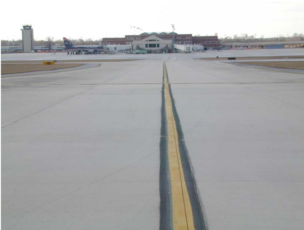
Overview of section TA2SV-20.
