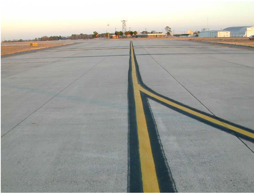
Overview of section TCSV-30.
