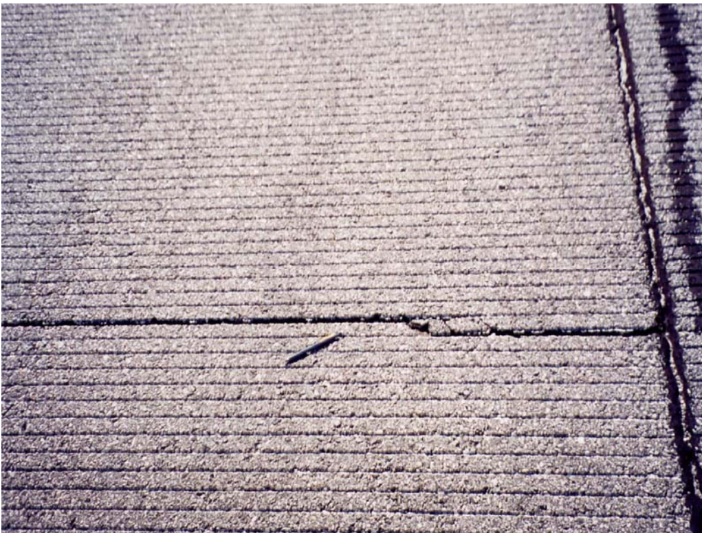
L&T cracking in section R725LW-10.
