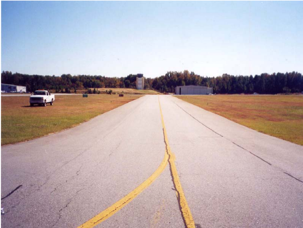
Overview of section TDLW-10.
