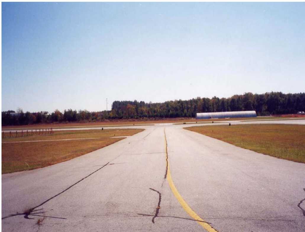
Overview of section TGLW-10.
