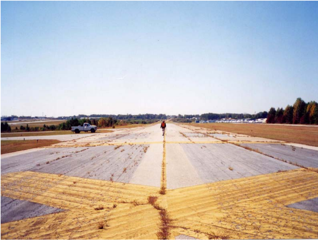
Overview of section TCLW-10.
