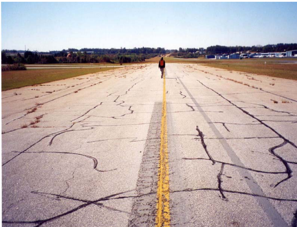
Overview of block cracking in section TCLW-10.
