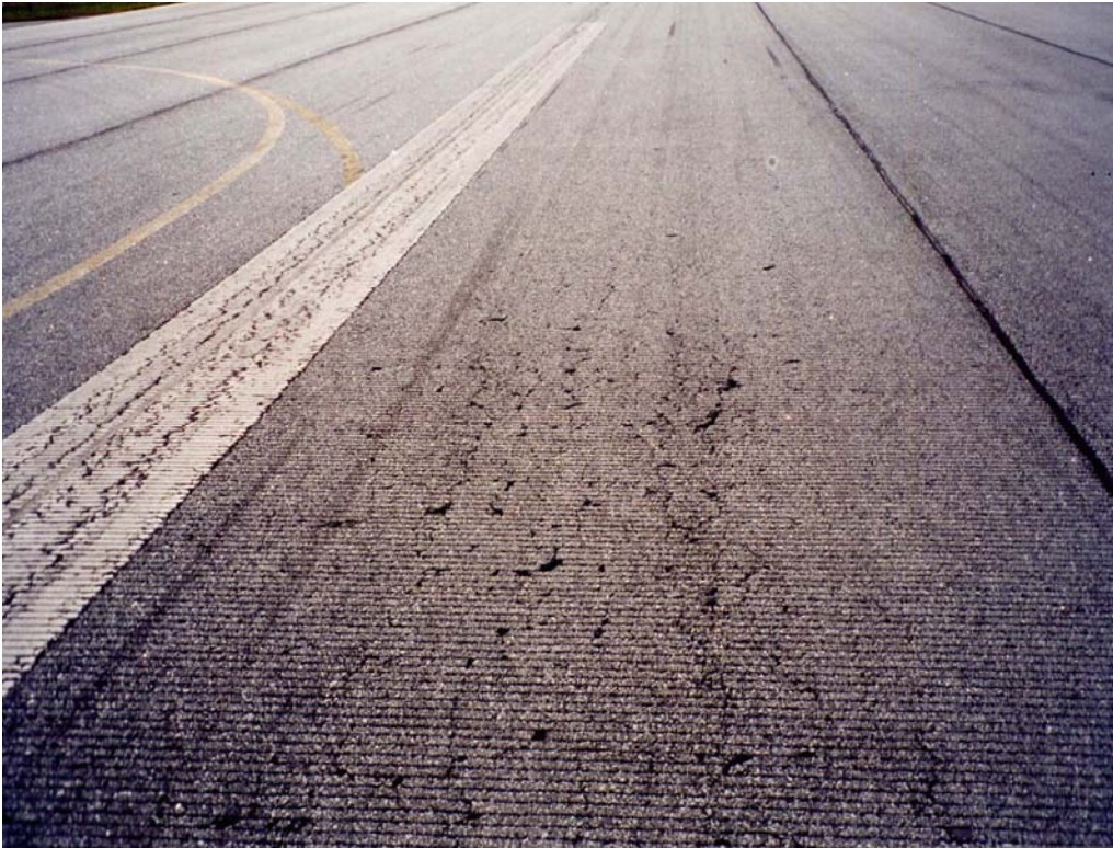
Alligator cracking in section R725LW-10.
