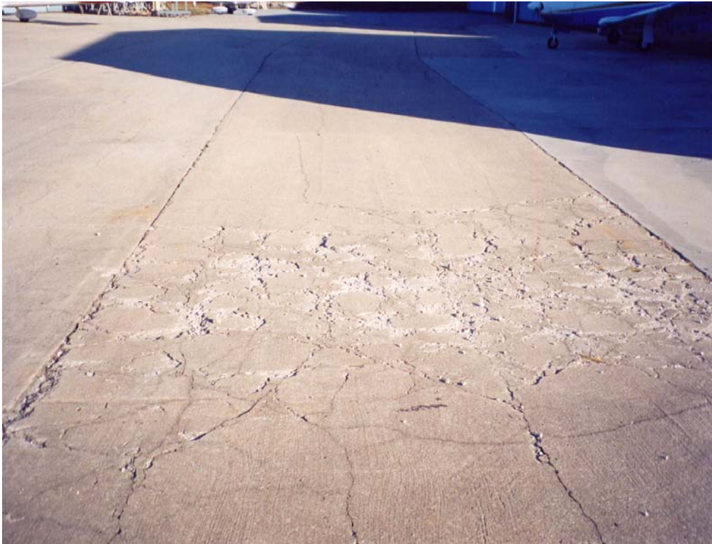
Shattered slab in section A01LW-40.
