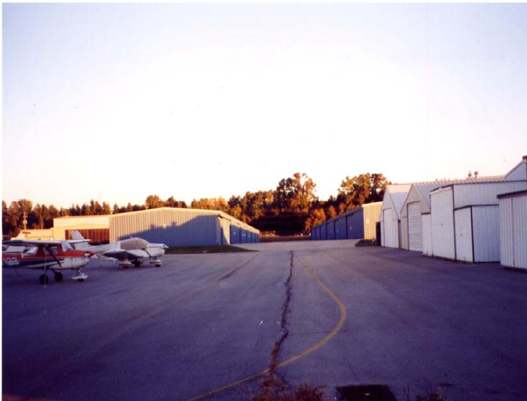
Overview of sections A01LW-10 and THANGLW-10.
