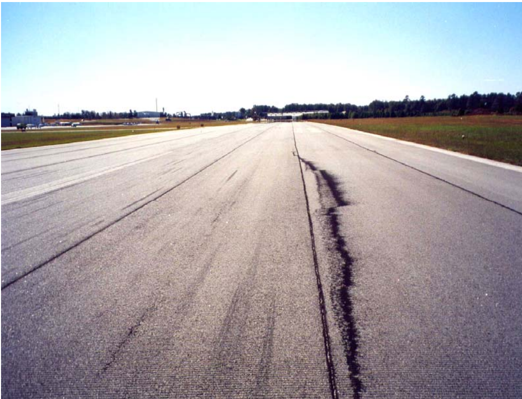
Overview of paving lane and longitudinal crack in section R725LW-10.
