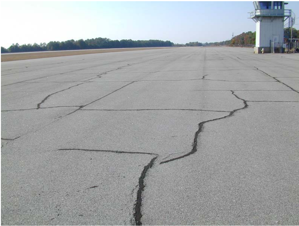
Overview of section ATOWERAG-10.
