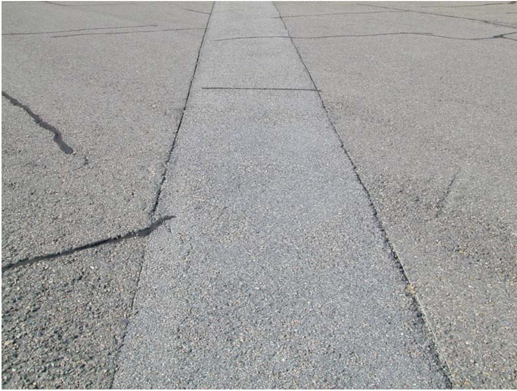
Patching in section ATERMAG-60.
