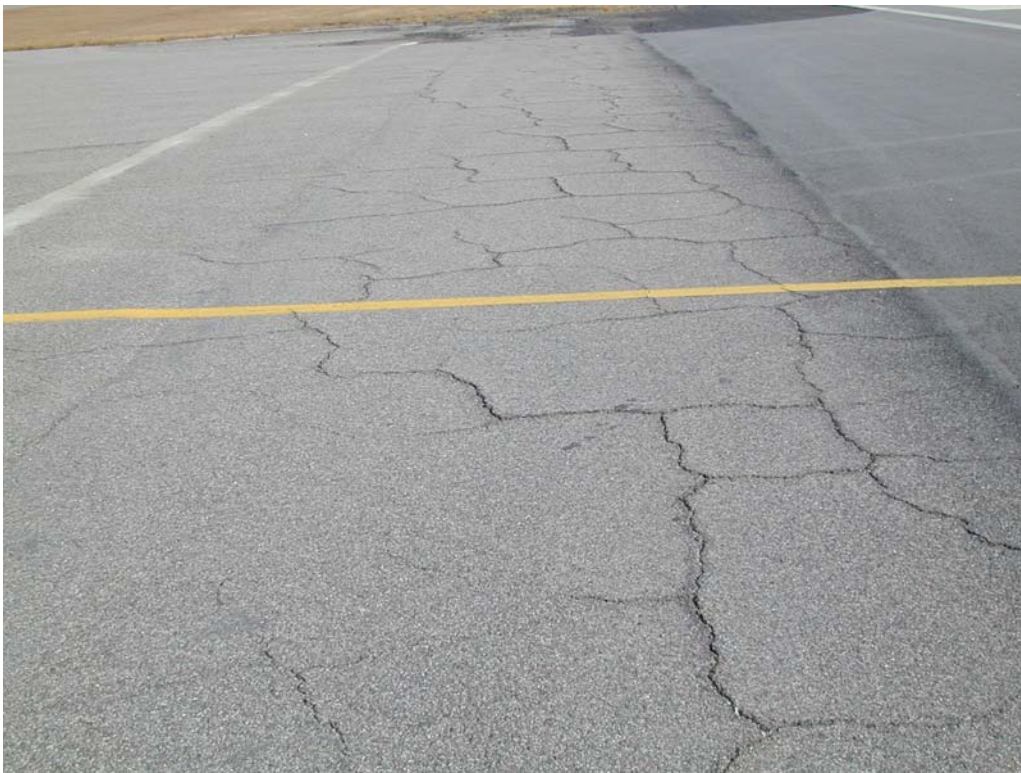
Block cracking in section ATOWERAG-20.
