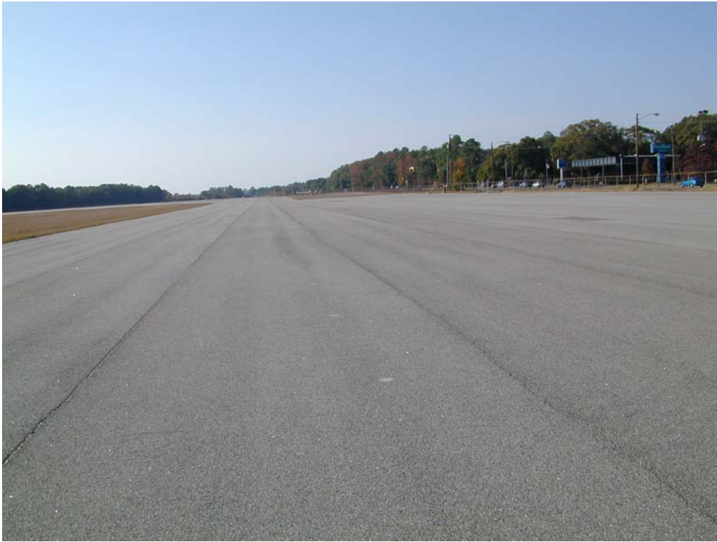
Overview of section ATOWERAG-20.
