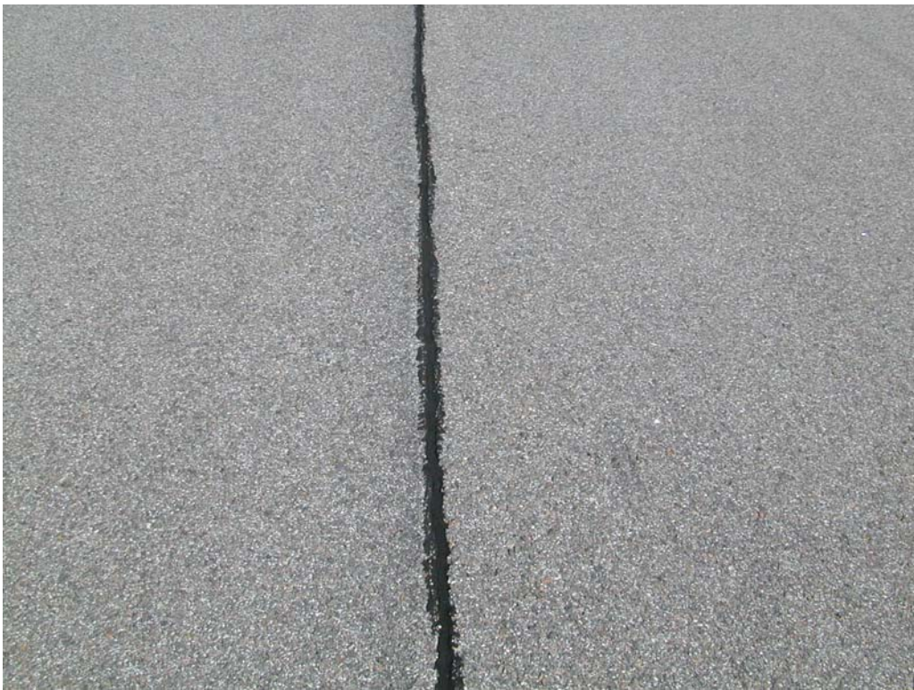
L&T cracking in section R523AG-10.
