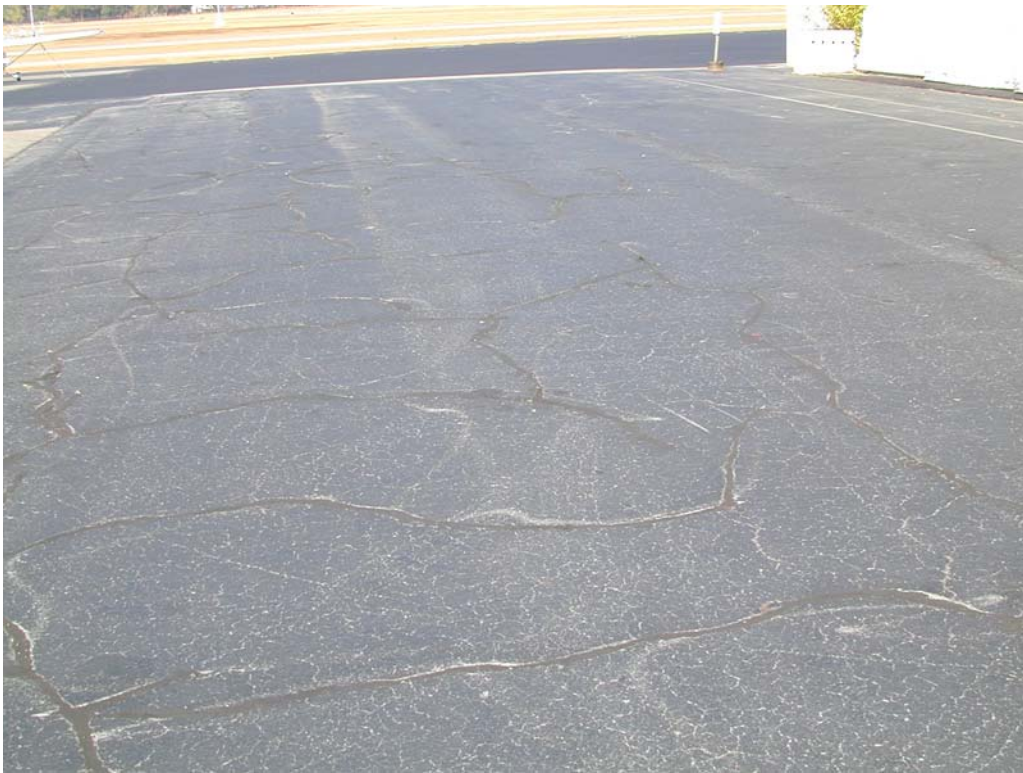
Block cracking in section ATERMAG-10.
