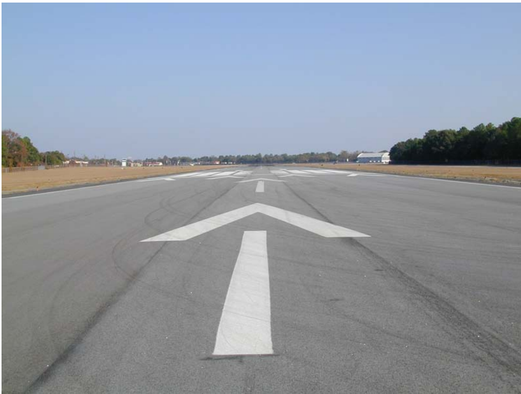
Overview of section R1129AG-10.
