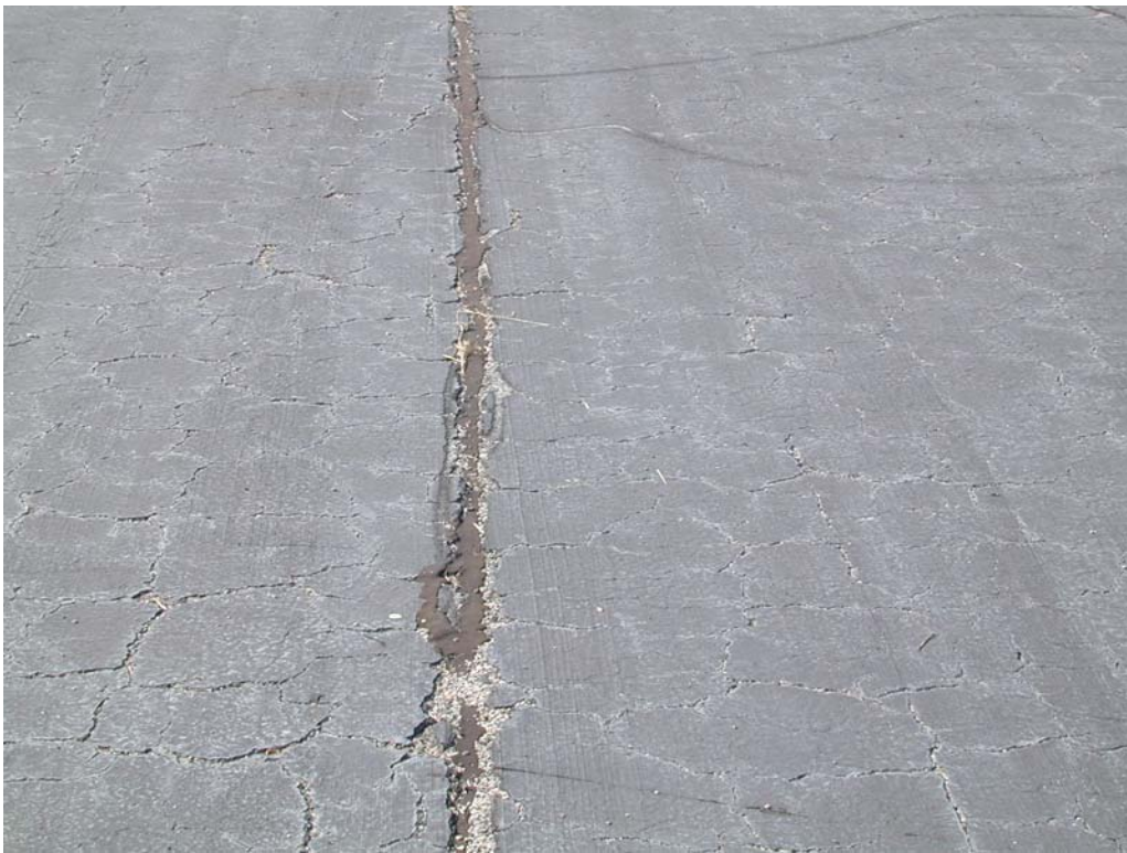
L&T Cracking in section ATERMAG-20.
