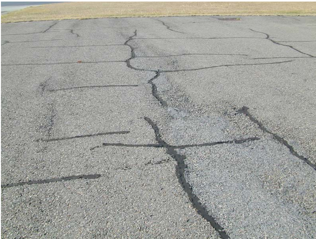
Block cracking in section ATERMAG-60.
