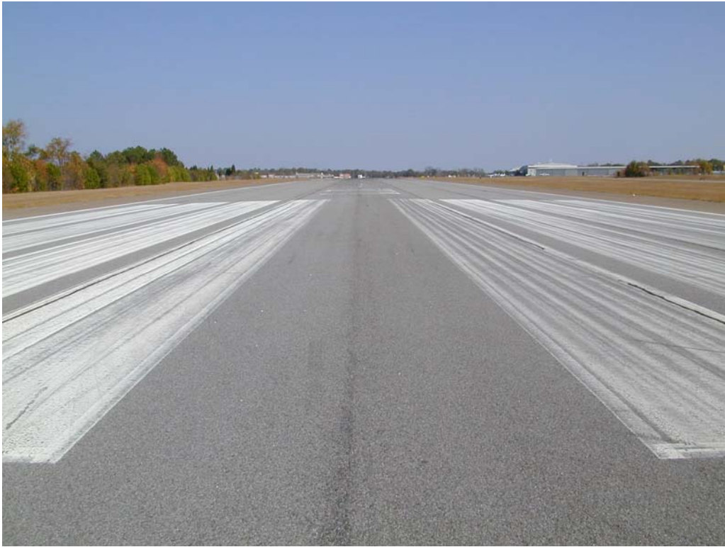
Overview of section R523AG-10.
