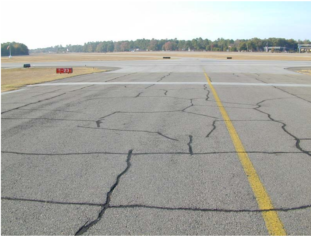
Block cracking in section TEAG-10.
