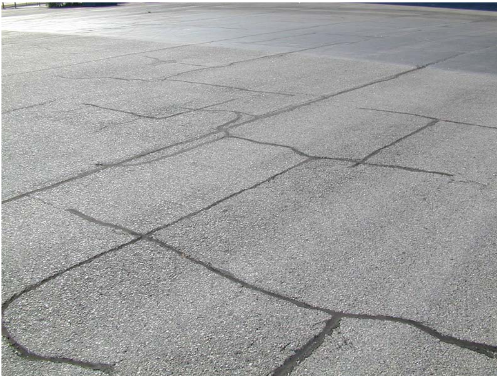
Block cracking in section ATERMAG-50.
