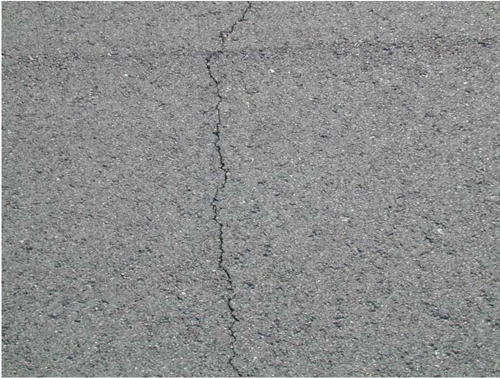
L&T cracking in section R1129AG-10.
