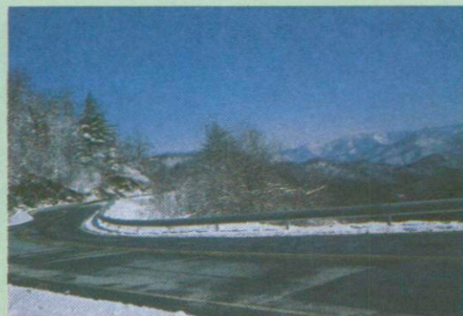
State Route 11, US 129, Union County
