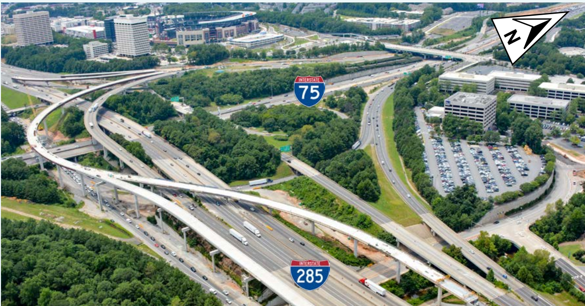
Aerial view of project progress at the I-75/I-285 Interchange
