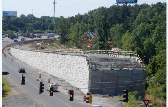
*New walls have been built next to the I-75 access ramps at North Marietta Parkway. These walls will eventually connect a bridge spanning over the intersection.*
