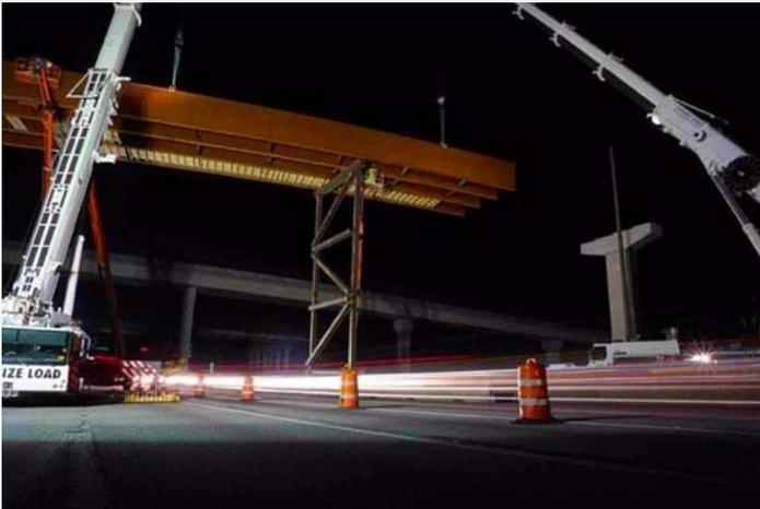
*Steel girder setting operation over I-75 for bridge construction in April.*
