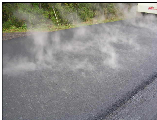
Figure 3-25 Paving of 9.5 mm Superpave mix
