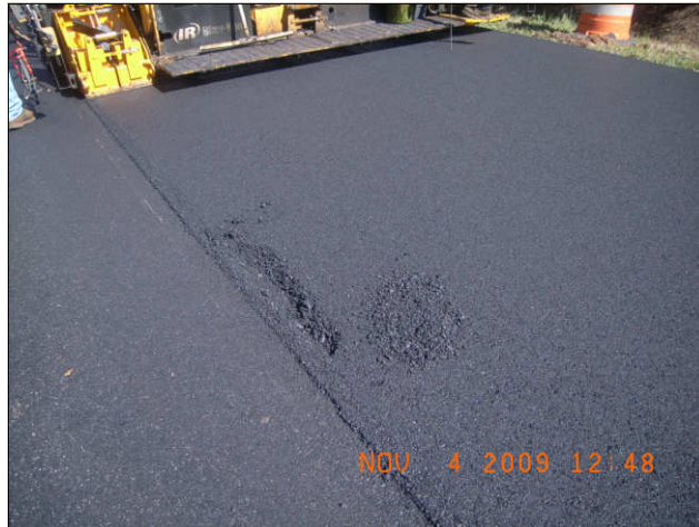
Figure 3-18 Blemish on Cecabase RT test section
