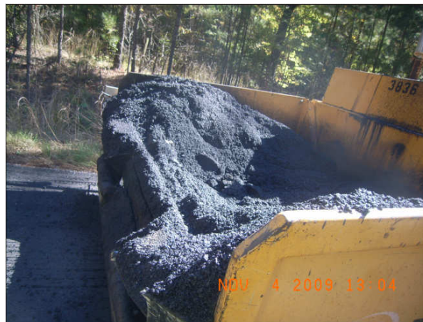
Figure 3-16 Cold mix clumps of Cecabase RT WMA in hopper
