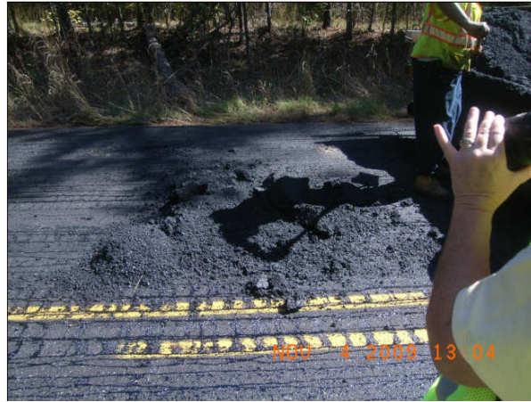
Figure 3-17 Removal of cold Cecabase RT WMA clumps from hopper
