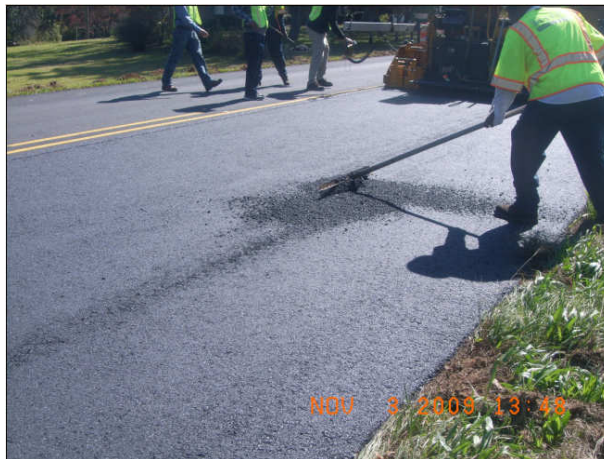
Figure 3-12 Blemish on Rediset WMA test section
