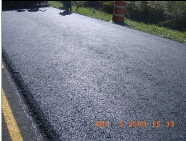
Figure 3-10 Gearbox stripping on Rediset WMA test section
