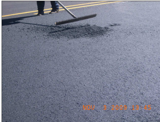
Figure 3-11 Blemish on Rediset WMA test section
