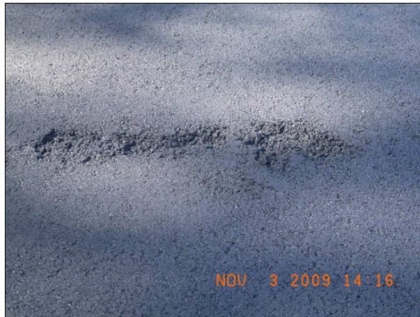
Figure 3-13 Blemish on Rediset WMA test section
