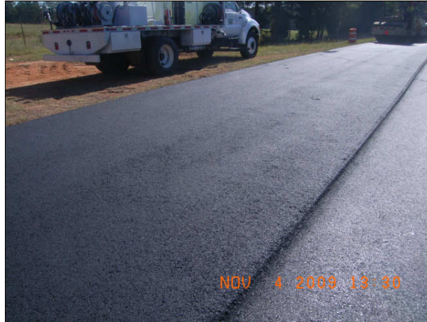
Figure 3-20 Pulling on Cecabase RT test section
