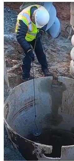
Figure 20. Photo. Entry view of a dry shaft.
