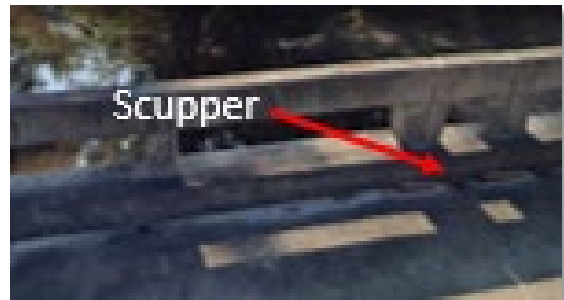
Figure 23. Photo. Bridge site SR297 from Google Maps showing scupper drain.
