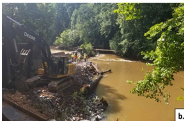
Figure 22. Photos of jetties. Temporary riprap construction structures implemented for bridge construction (a) and dam removal (b). The bridge construction picture (a) was taken at the Chattooga River Georgia Department of Transportation bridge construction site.
