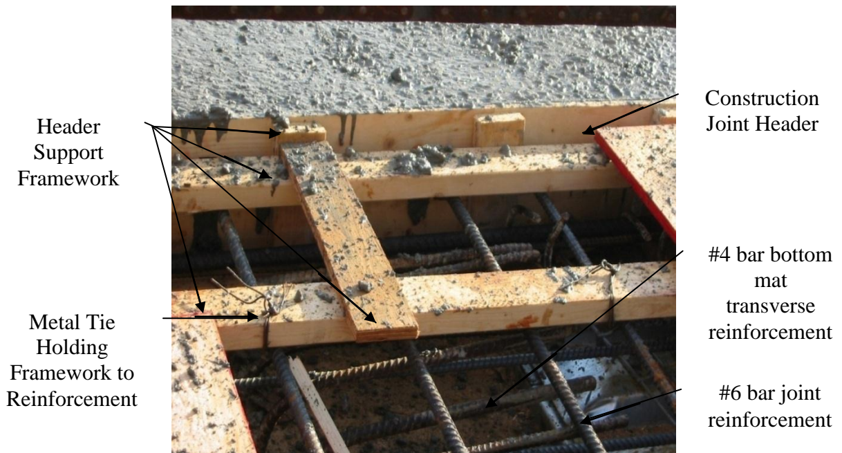
Figure 3.2.1.2 – Header construction layout for #6 bars in continuous deck detail (bridge supporting GA SR 113 at Etawah River)
