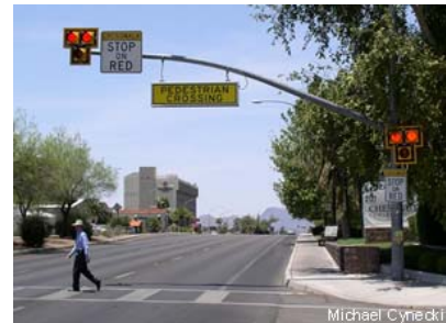
HAWK Signal, Tucson, AZ. Courtesy of The National Center for Safe Routes To School ( www.saferoutesinfo.org ).
