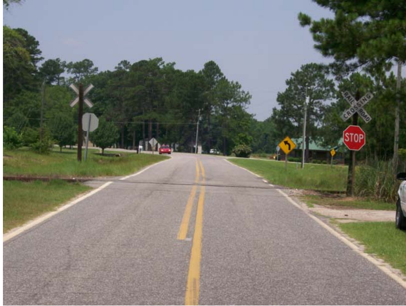
Rail Crossing 723450U - Blasingame Road, West of Old Albany Road
