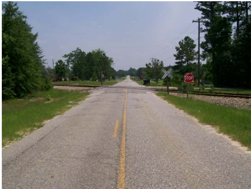
Rail Crossing 723449A - Old Albany Road, south of Blasingame Road
