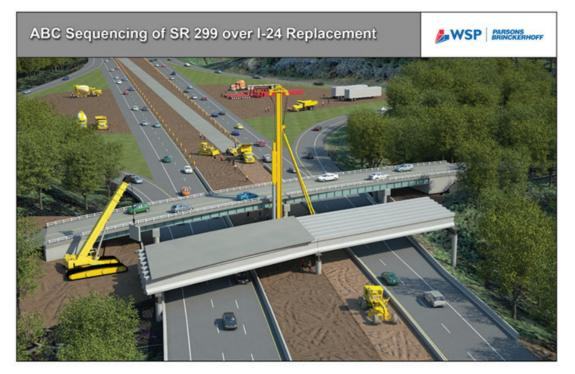
**Phase 2:** The existing bridge is demolished one side at a time and replaced in sections, while traffic is diverted to the opposite side on I-24.
