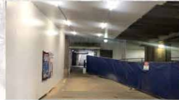
Protected Channelized Walkway
