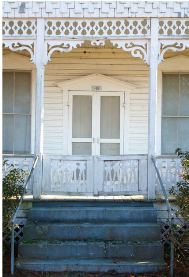
(Above) The double doors at the front entrance are capped with a pediment. The spindlework friezes and the ornamental porch balustrade are examples of components that were being mass-produced during the period of rapid industrialization from 1860-1900.
