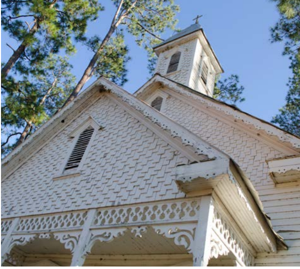
(Left) The louvered window openings on the bell tower allow the sound of the ringing bell to carry over the surrounding area. The bell can be rung by pulling a rope located in the interior of the church.
