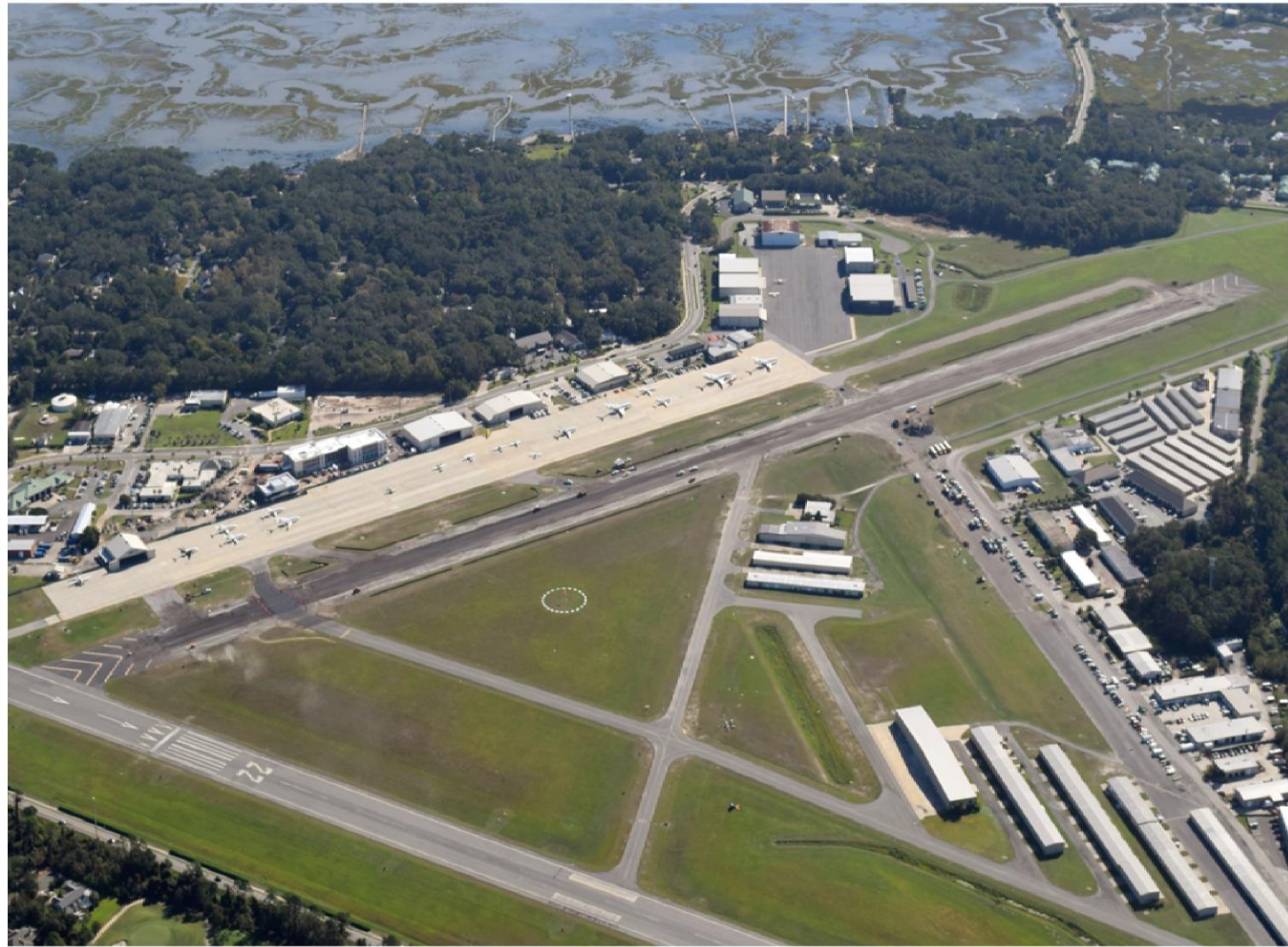
St. Simons Island – 16/34 Rehab & Replace Lighting $2,473,241
