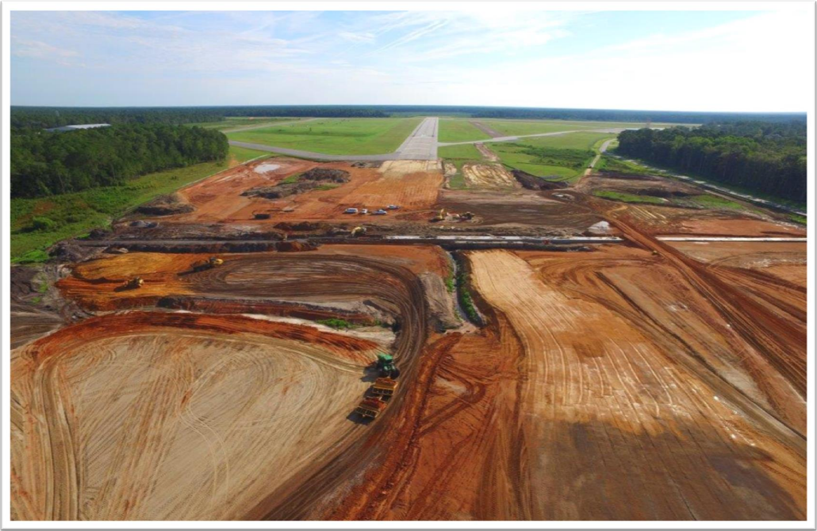
MidCoast Regional/Wright Army Airfield – Runway Extension $14,611,907
