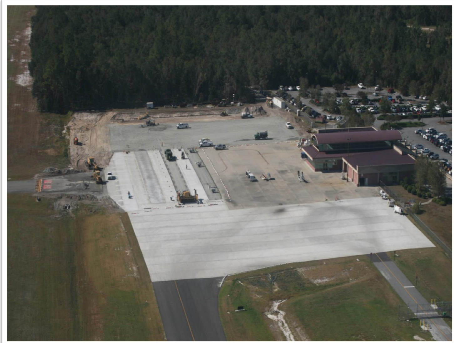
Valdosta –Terminal Apron Expansion $3,648,134
